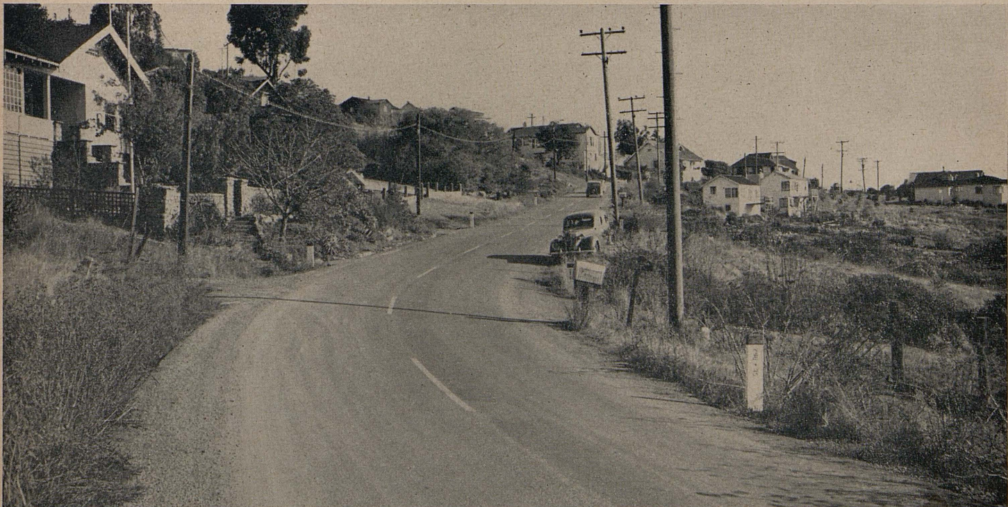
Marin Access Road to Dry Dock Training Center and Naval Net Depot on Tiburon Peninsula. View is looking north
