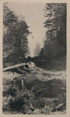
Grading a line change on north bank of Smith River, Del Norte, to by-pass a weak timber bridge
