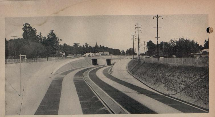
1—Looking easterly toward the Orange Grove Avenue overpass in South Pasadena. This is one of the bridges over the Arroyo Seco Parkway between Los Angeles and Pasadena opened to traffic in July, 1940. To save right of way cost, slopes were constructed on 1:1. Soil encountered was sandy gravel and clay loam.
