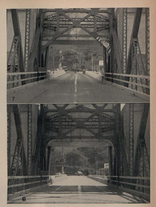
Improvement of vertical clearance by replacement of main trunion braces on the Petaluma Creek Bridge
