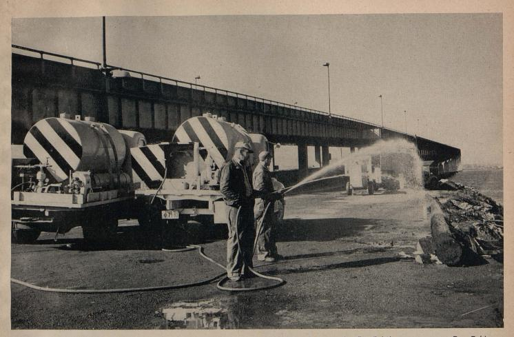
Truck-mounted tanks are 580-gallon capacity equipped with small, centrifugal pumps for fire fighting purposes on Bay Bridge
