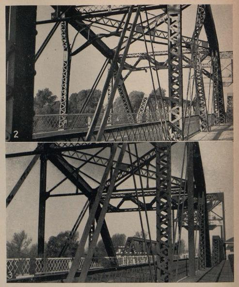
Before and after pictures of traffic damage repair on the Mossdale Bridge. Figure 3 shows the damaged posts replaced with H beams
