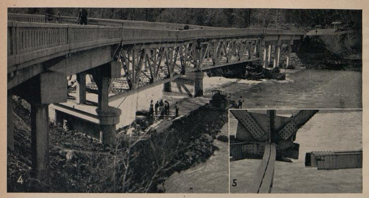
The damaged Trinity River Bridge with temporary repairs under way. Inset shows the severed lower chord
