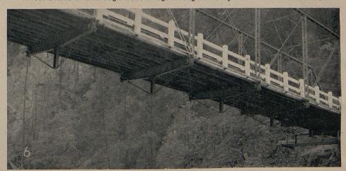
type floor may provide the proper strengthening by better distributing the wheel loads to existing stringers.
