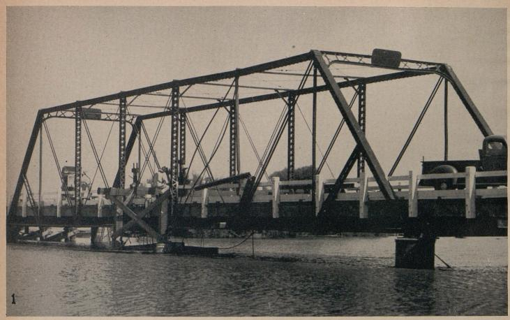
Repair of traffic damage at Kings Slough Bridge. Truss has been jacked back to grade through C. M. P. caissons and temporary supports placed under top chord. The broken vertical posts, bent almost double, shown in the center foreground
