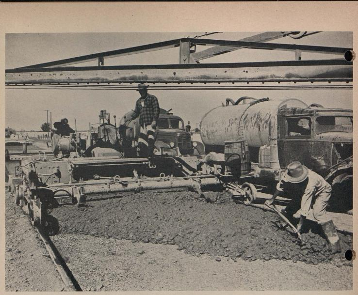
Vibrator spreader attached to tamping and kneading machine. Operator is backing up header where key is attached
