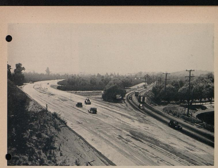
Redlands project showing old road on right and grading for new 4-lane highway construction on left
