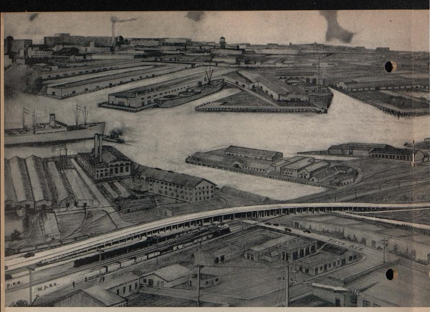
Engineer's sketch of Fifth Avenue Overhead, initial unit of the East Shore Freeway in Oakland, now under construction. The overhead structur tracks of the Western Pacific Railroad, the tracks of the Southern Pacific Company, and finally Fifth Avenue. After an easy descent, the overh
