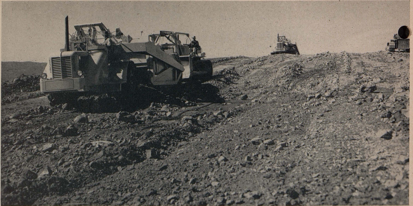
Here a Terra-Cobra with caterpillar dozer pusher is excavating rocky material
