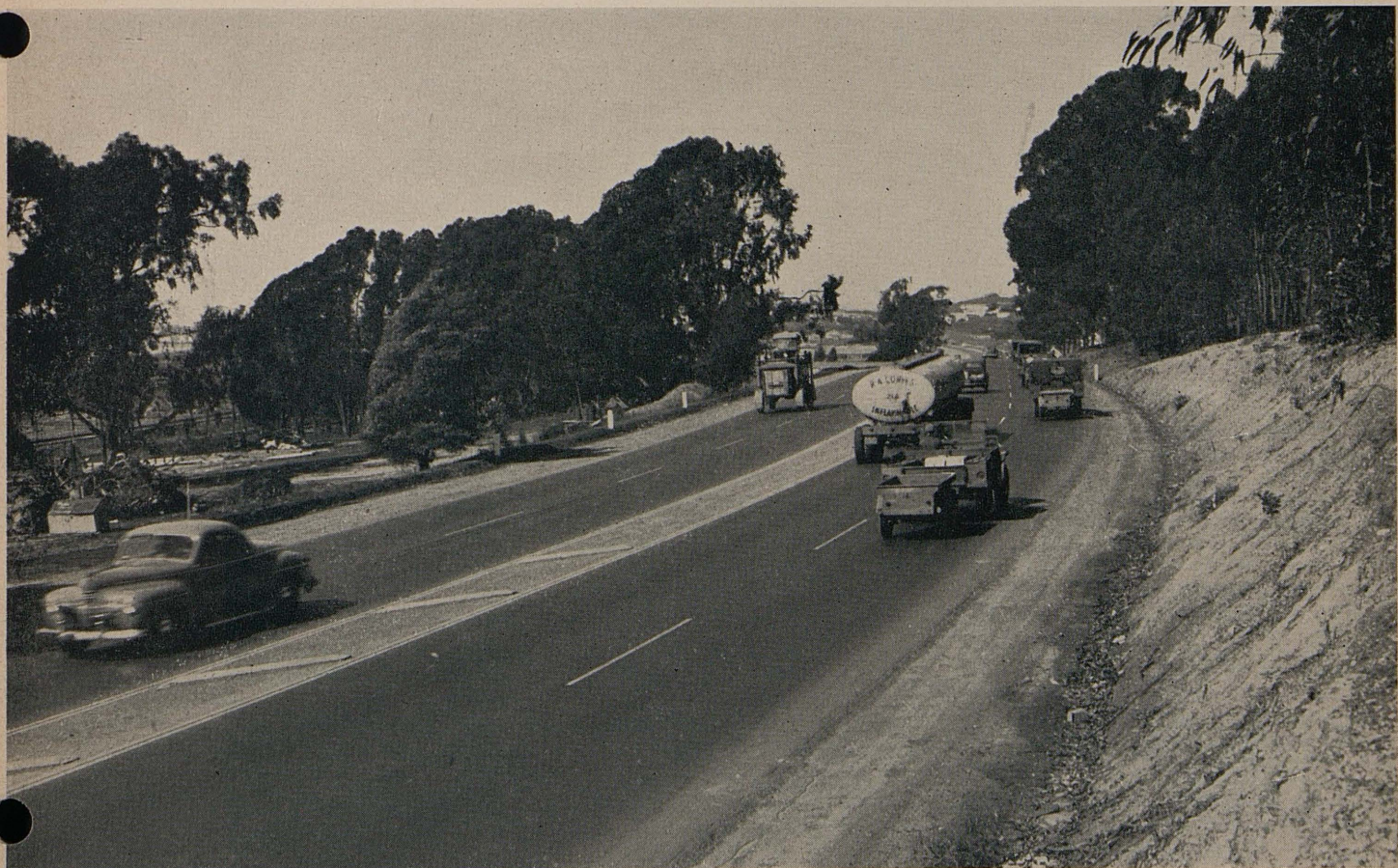
Two 21-foot lanes of asphalt concrete pavement on U. S. 40 in Alameda County, near El Cerrito Overhead
