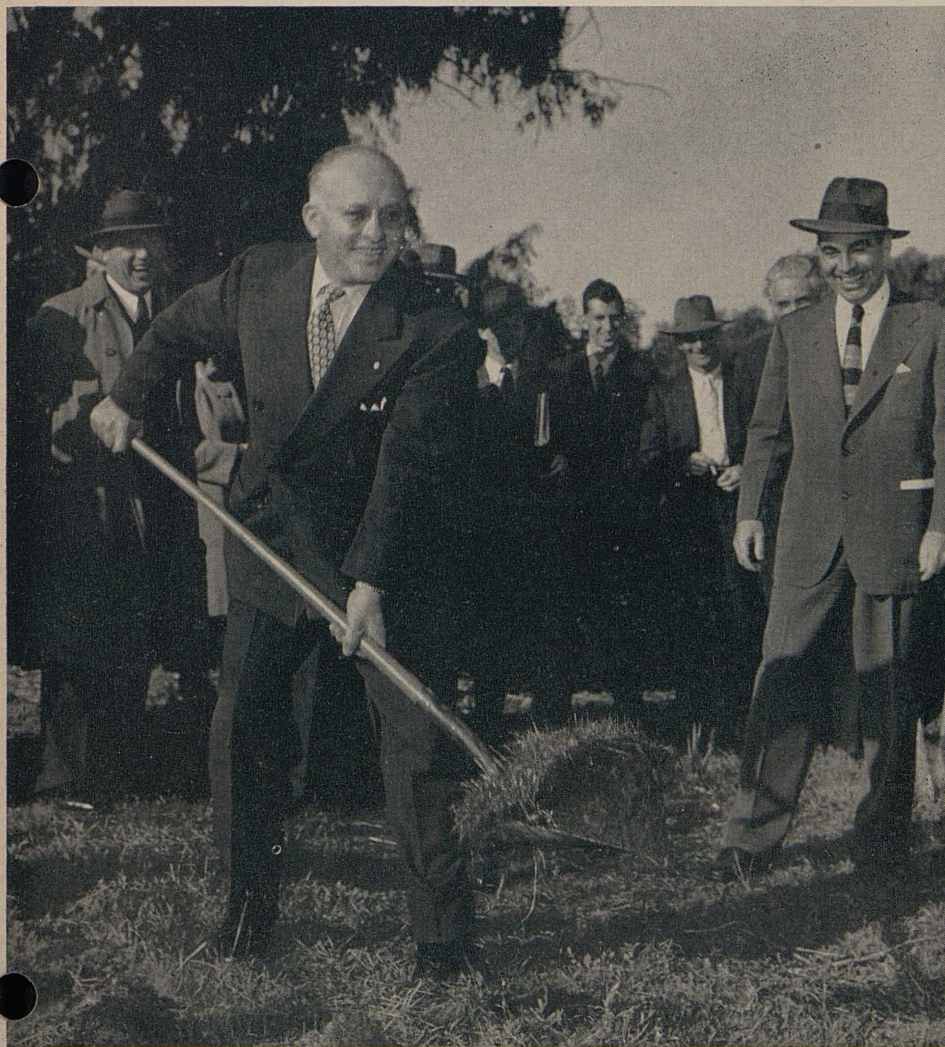
While Highway Commissioner C. Arnholt Smith (right) looks on, Mayor Harley Knox of San Diego breaks ground for the new Cabrillo Freeway
