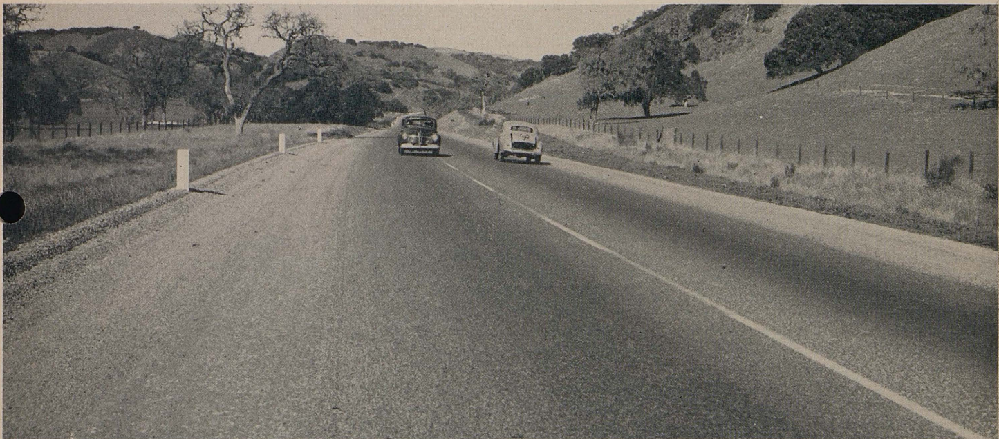
This photograph shows a plant-mix surface repair project north of Buellton in Santa Barbara County
