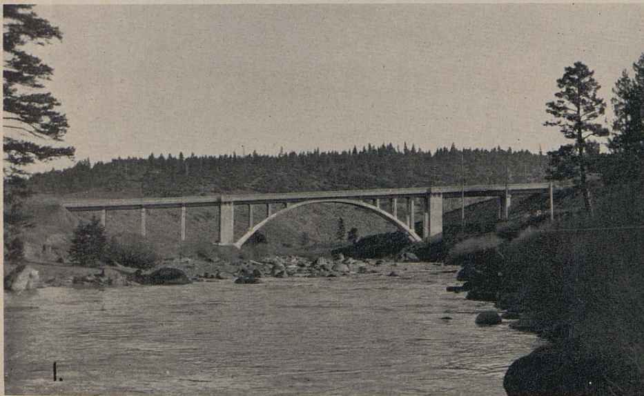
Truckee River Bridge near Polaris on U. S. Highway 40
