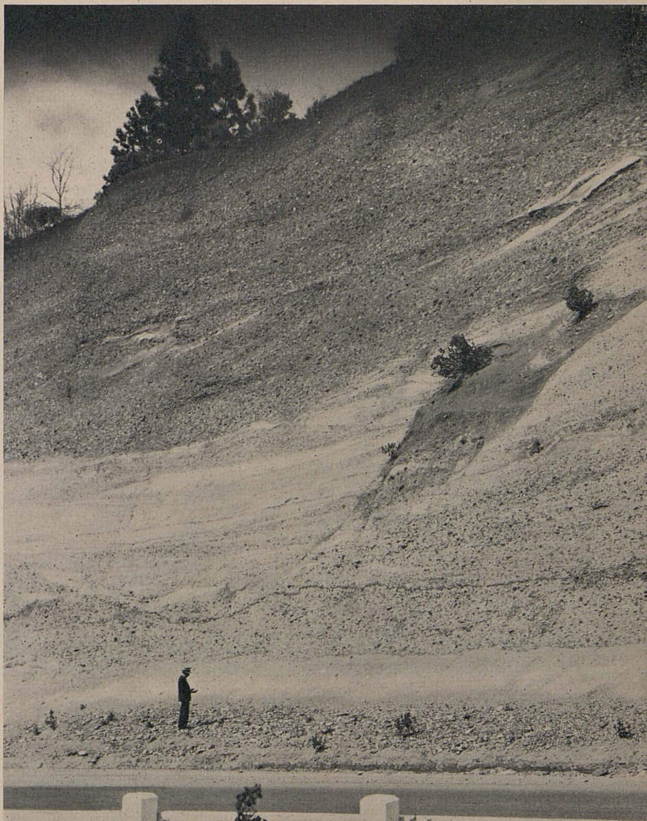
Section of gravel deposits, thirty million years old, on U. S. 40 near Gold Run
