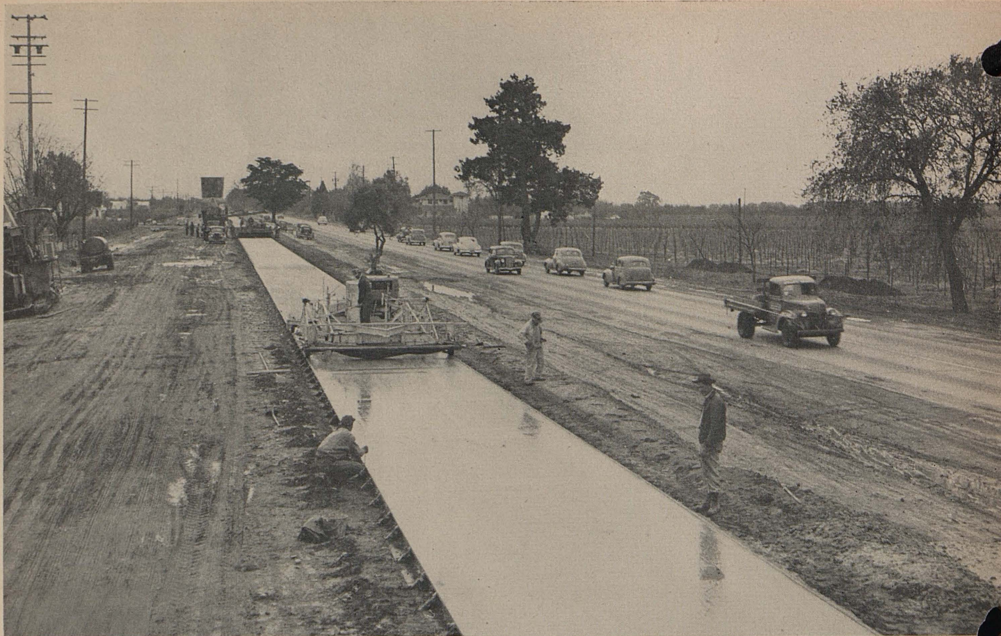
Johnson finishing machine at work on newly laid Portland cement concrete
