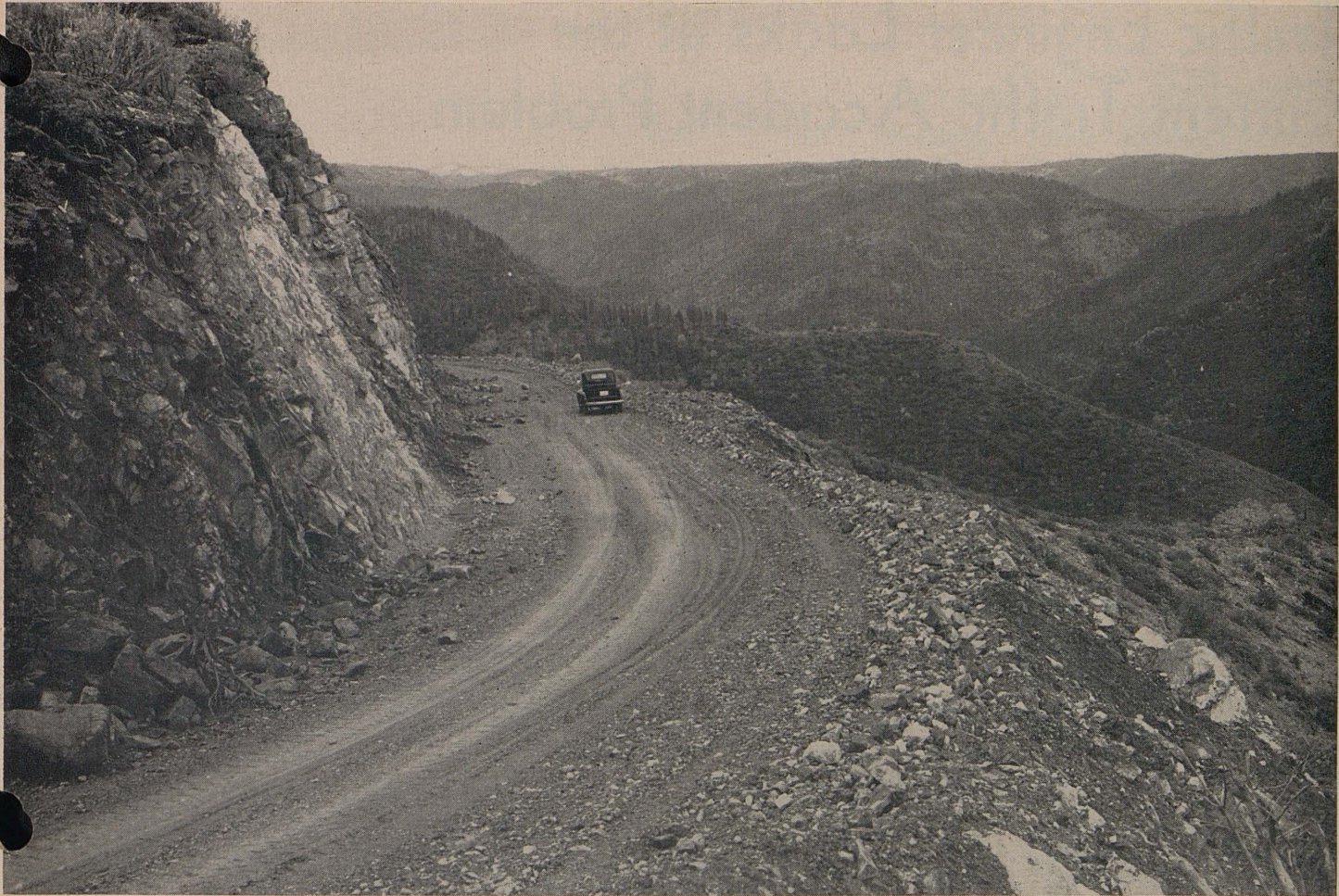
This road when completed will carry to market millions of board feet of sorely needed lumber
