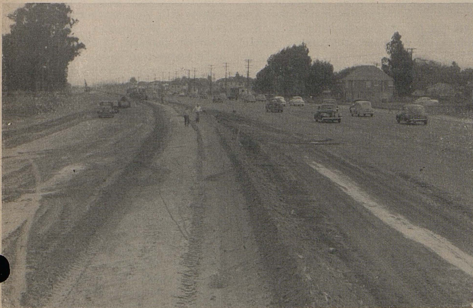
Looking south showing construction of final subgrade
