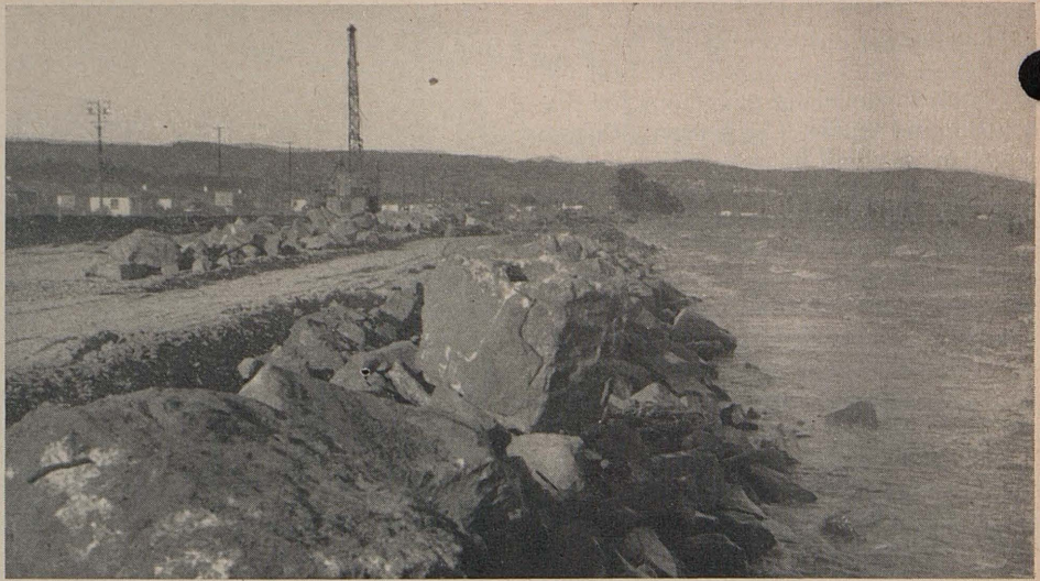
Looking north along riprap wall and adjacent fill
