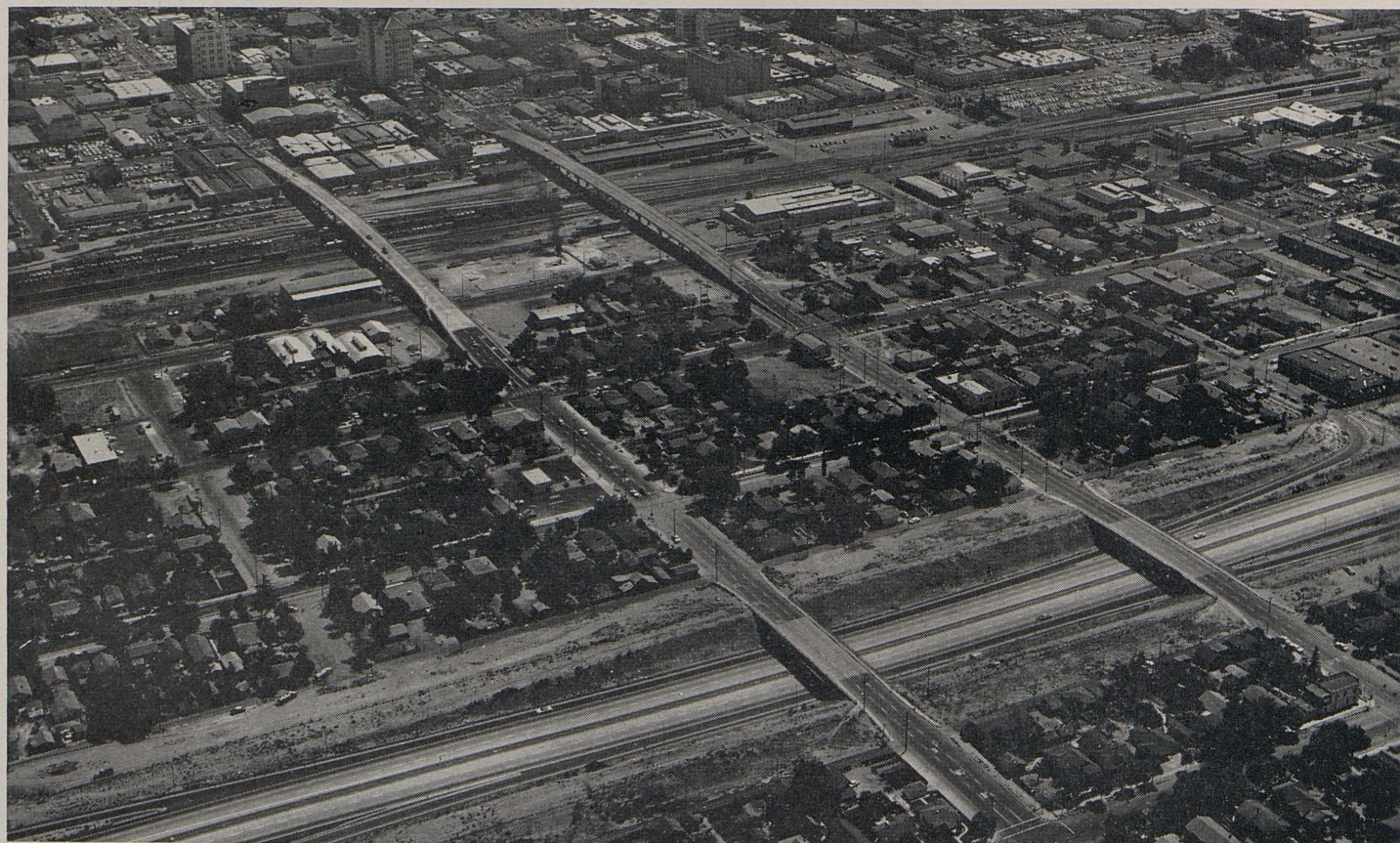
UPPER—The new separation structure carries traffic over Garces Circle in Bakersfield. This view is to the south along Chester Avenue with US 99 crossing the photo from left to right. LOWER—A view eastward over the City of Fresno. Tuolumne and Stanislaus Streets cross the Southern Pacific Railroad in the center and the US 99 freeway in the foreground.
