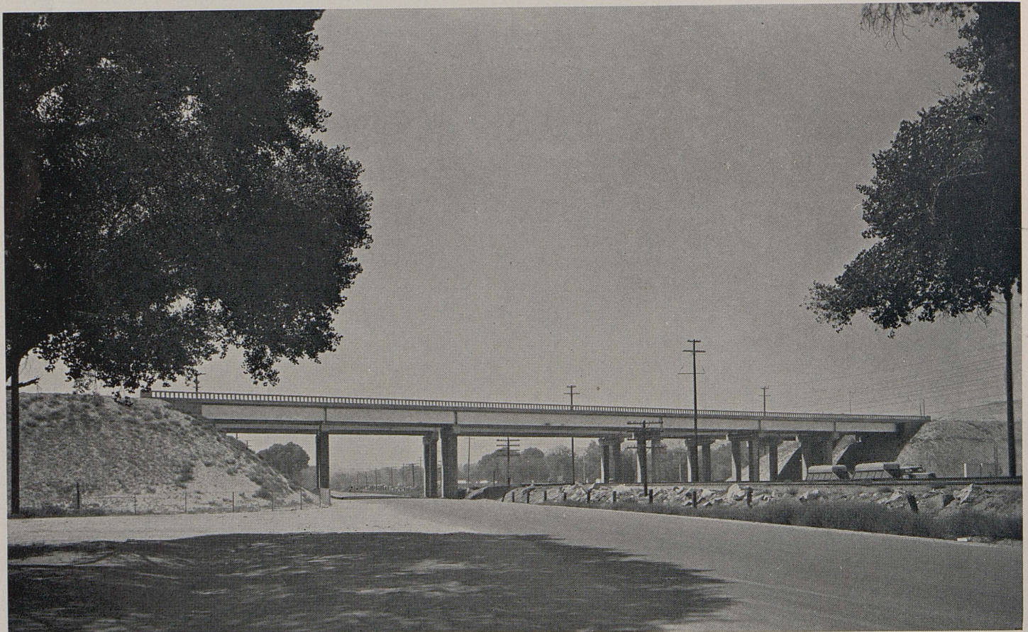
The Victorville Overhead carries the new freeway over the old highway and railroad tracks
