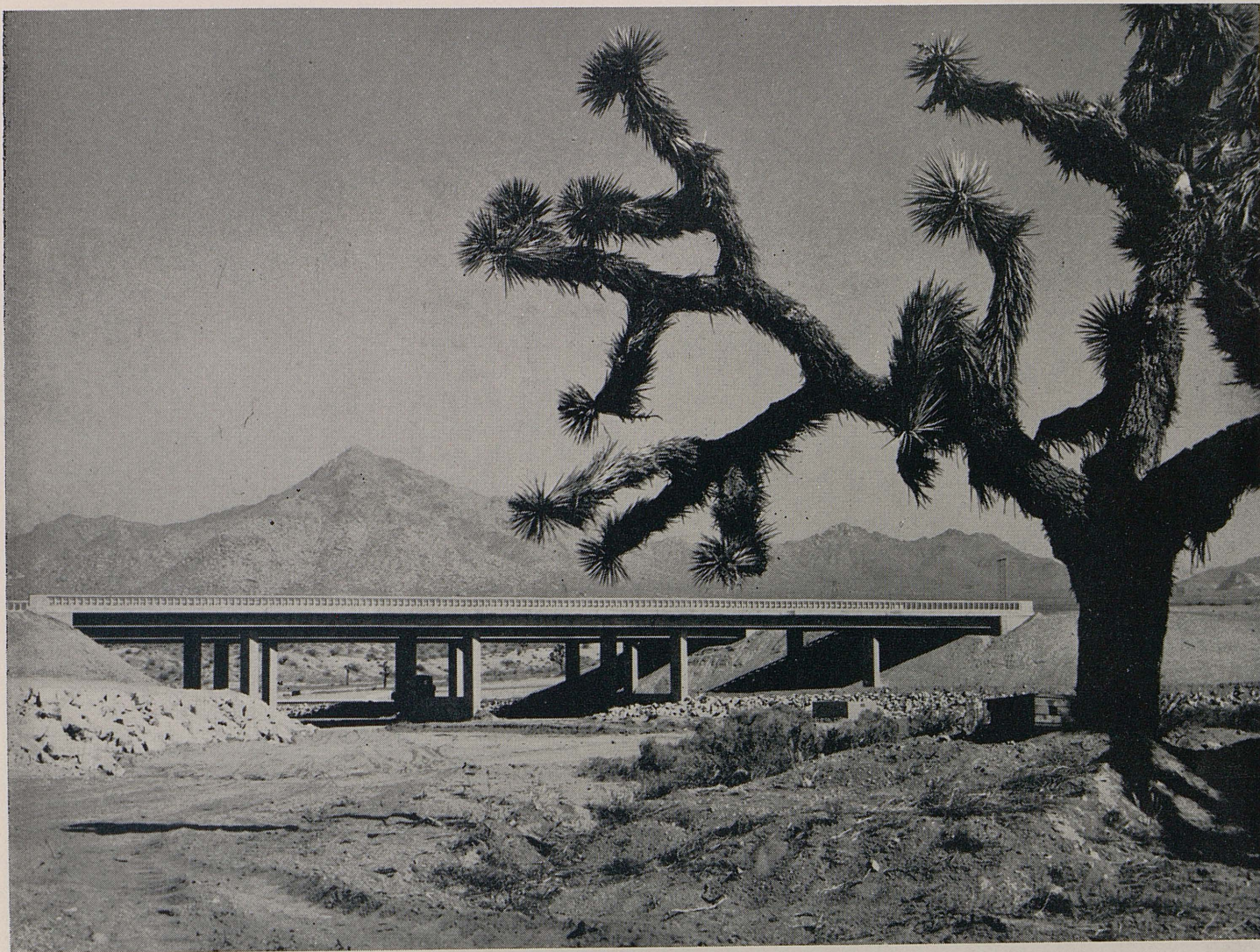
A typical drainage facility along the new freeway is the Bell Mountain Wash Bridge, shown above
