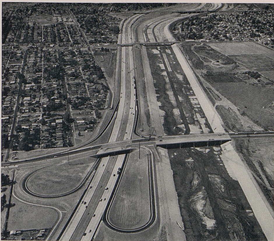
An aerial of the Olive Street Interchange on the Long Beach Freeway. The view is northward.
