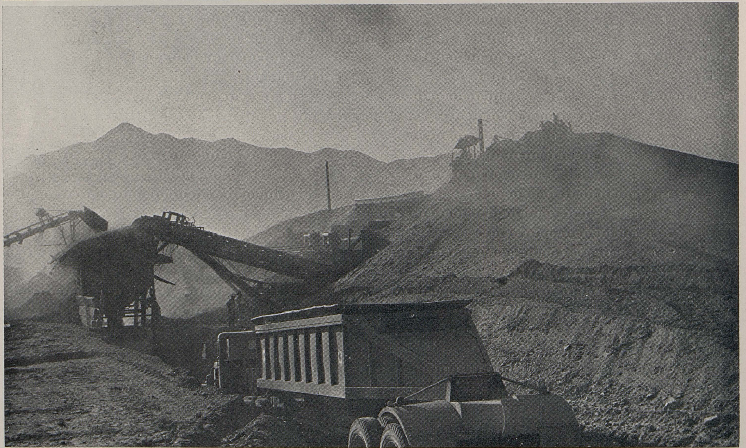
UPPER—Trucks wait in line on the Victorville-Barstow job and then (LOWER) they are loaded at the Wild Wash base material plant
