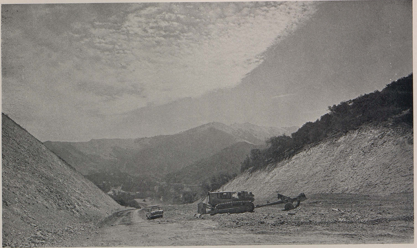
Relocation of Sign Route 166 because of the construction of Twitchell Dam and eventual flooding of the present highway by the reservoir has required several large cuts and fills through rugged mountain terrain
