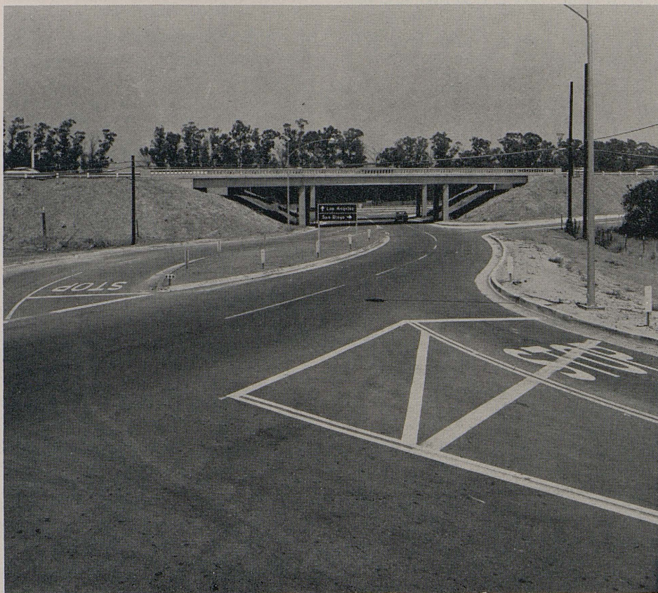
UPPER—A view southeast from Jeffrey Road toward the Town of Irvine along the newly completed section of the Santa Ana Freeway. LOWER—The Culver Road undercrossing on the new freeway. Culver Road connects with the county highway leading to the main entrance of the El Toro Marine Air Station.
