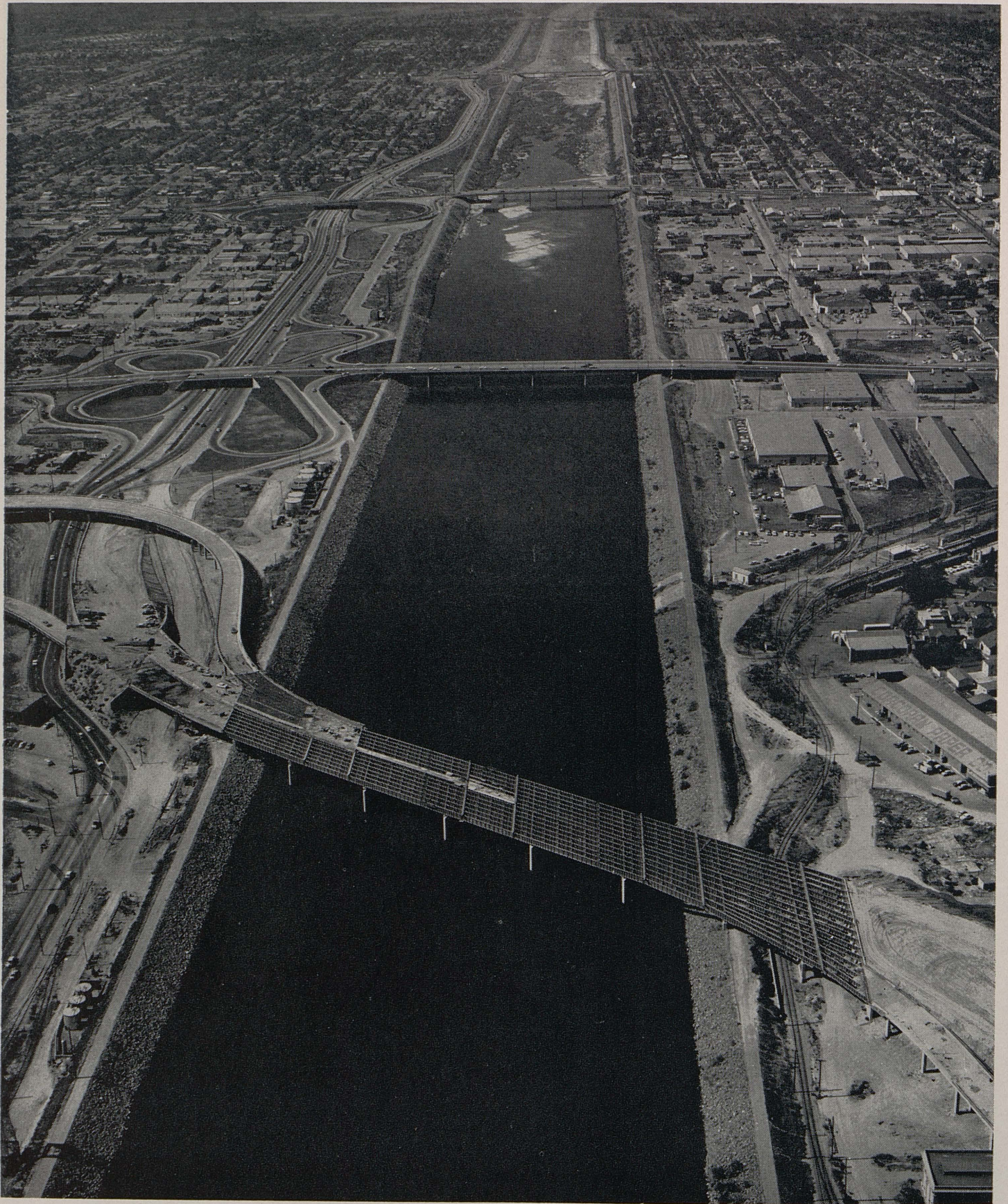
Looking north along the Los Angeles River and Long Beach Freeway showing the Ninth Street Bridge in the foreground, the Anaheim Street Bridge next and then the Pacific Coast Highway
