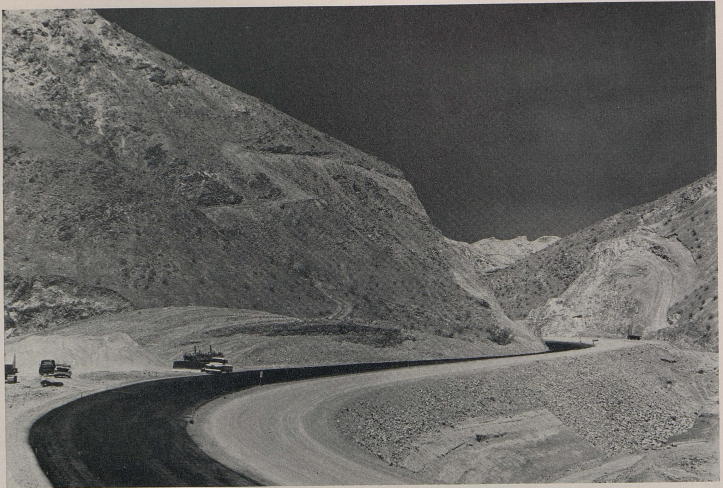
New four-lane expressway construction in Red Rock Canyon north of Mojave on US 6. The high rock cut and channel excavation on the right were necessary to make room for the highway and flood channel in the canyon.
