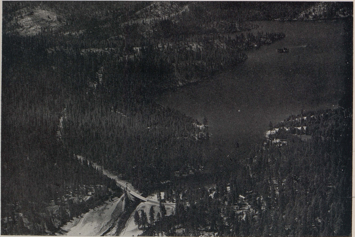
Sign Route 168 crosses Rancheria Creek at Huntington Lake in Fresno County. The China Peak ski area is in the upper left corner of the photo.
