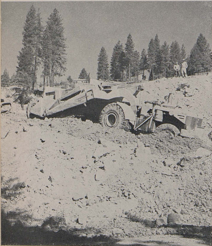
Self-propelled scrapers and bulldozers cutting stabilization trenches near Alta.
