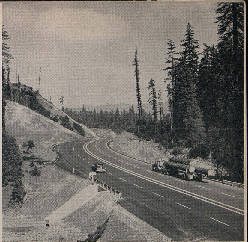
A portion of the completed first unit of the Redwood Parks Freeway on U. S. Highway 101 north of Dyerville at High Rock Road Undercrossing.
