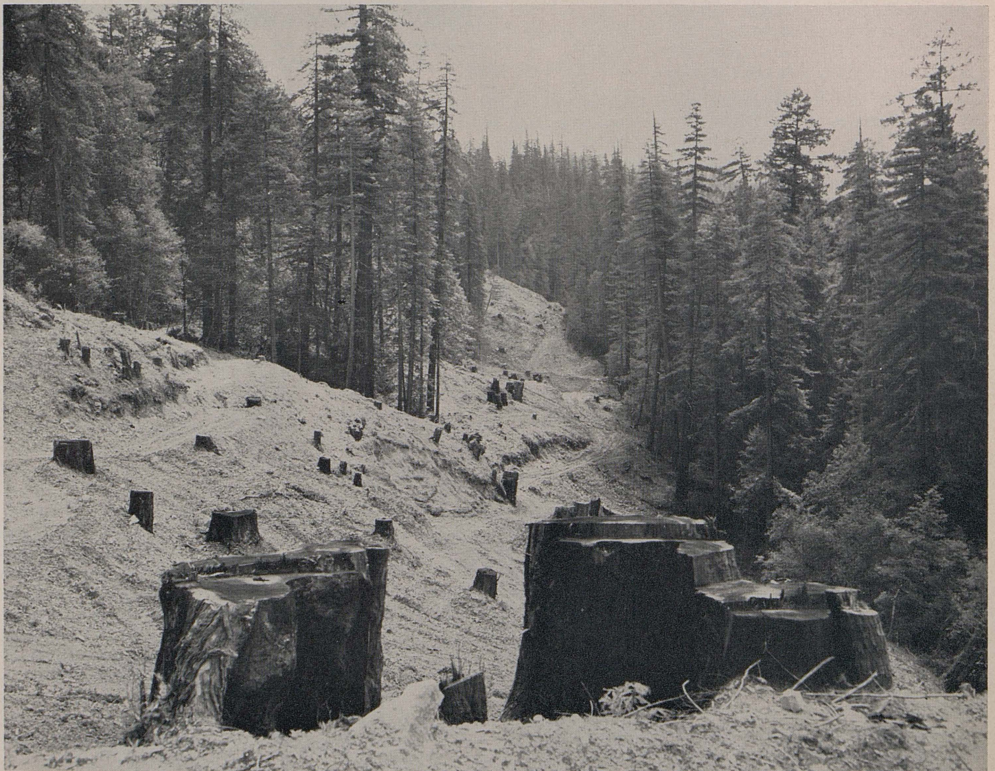
A cleared area prior to grading operations on the second unit of the Redwood Parks Freeway (US 101) between Myers and Dyerville in Humboldt County.
