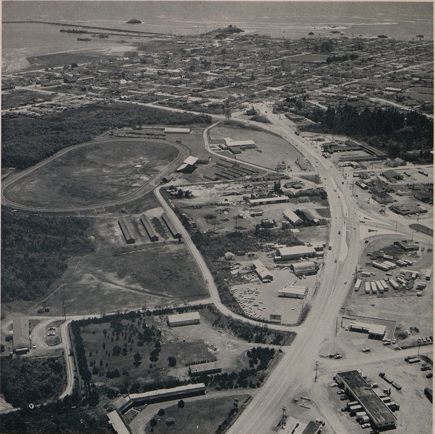
A recent improvement made US 101 through Crescent City in Del Norte County a one-way couplet with four-lane approaches. This southwest view shows the US 101-Northcrest Drive intersection in the right center.
