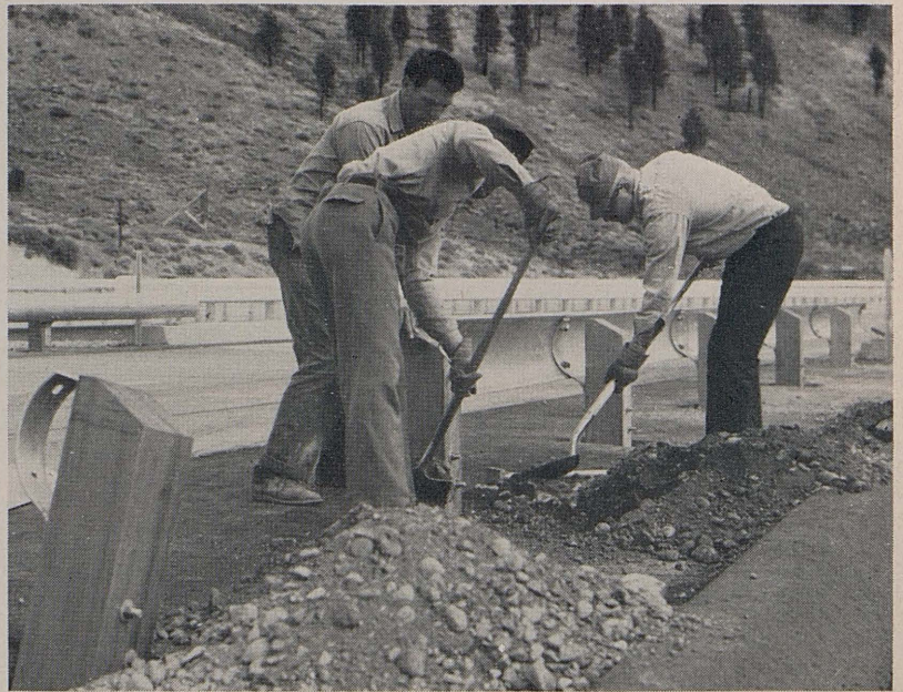
Crew setting guard railing on Boca Bridge approach.
