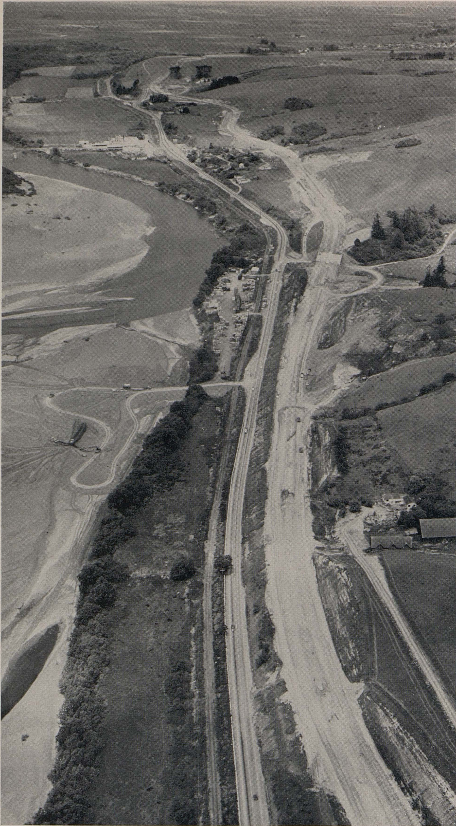
Looking north along the construction of the freeway on US 101 between Fortuna and one mile north of Fernbridge in Humboldt County.
