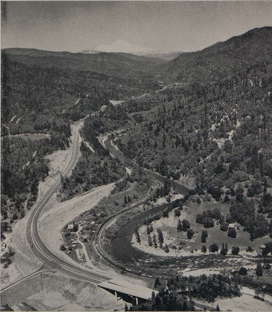
A new expressway section on U. S. 99 in the Sacramento River Canyon, Shasta County. Slate Creek Bridge is in the foreground; Mount Shasta in the background.
