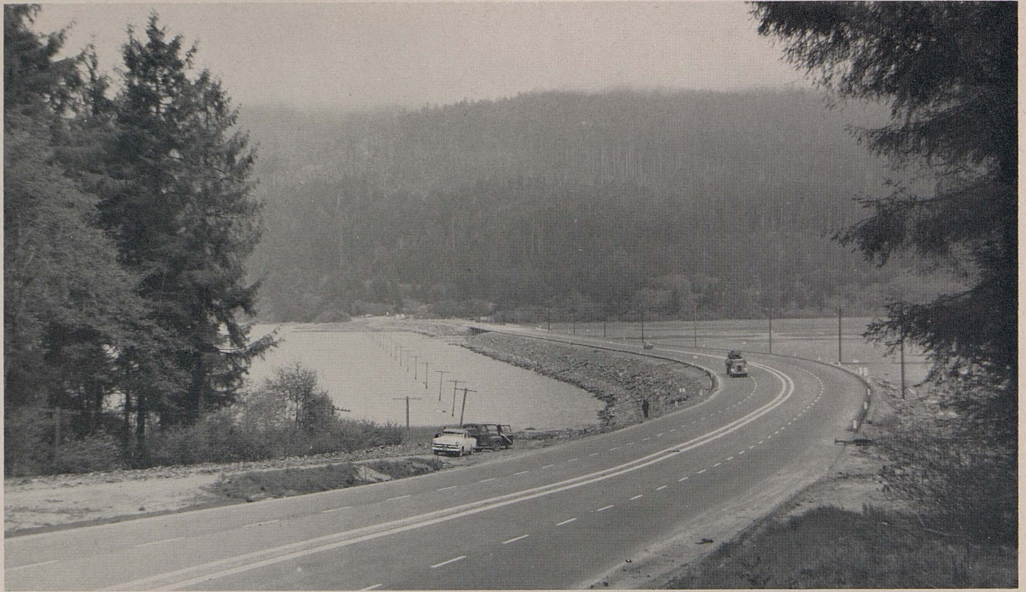
A recently completed freeway section on US 101 between Patricks Point and Big Lagoon in Humboldt County. This northward view shows the embankment across Big Lagoon which replaced the former timber trestle.
