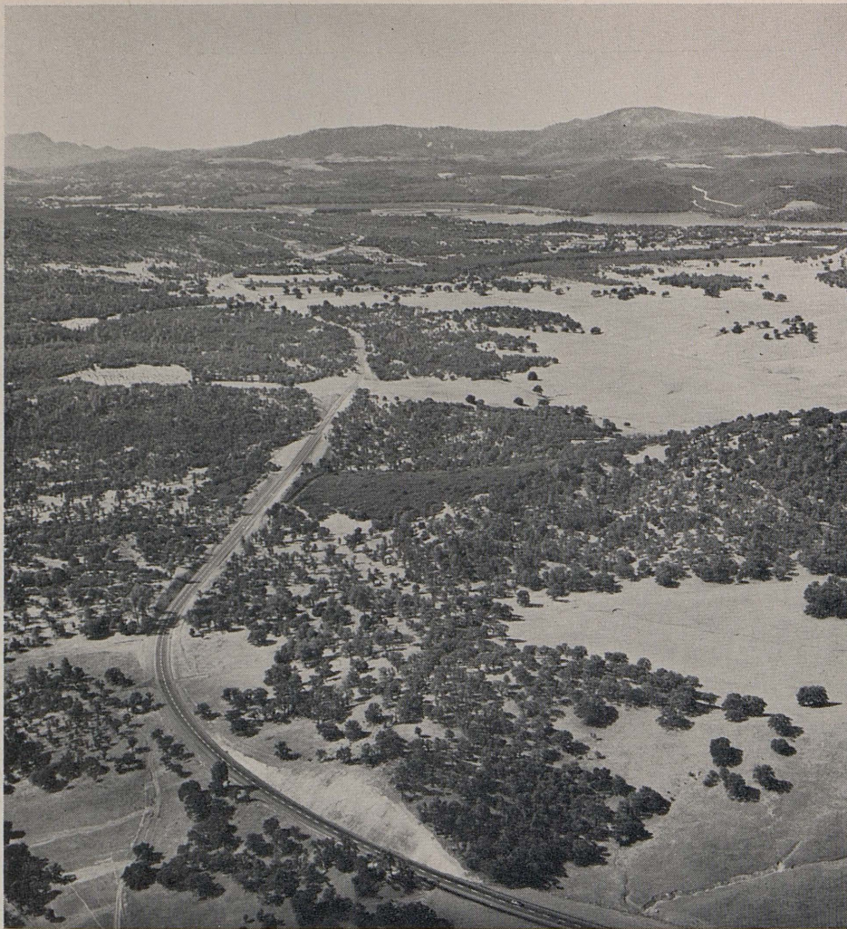
A southward view of the Sign Route 53 relocation in Lake County showing the south end of Clear Lake in the background.
