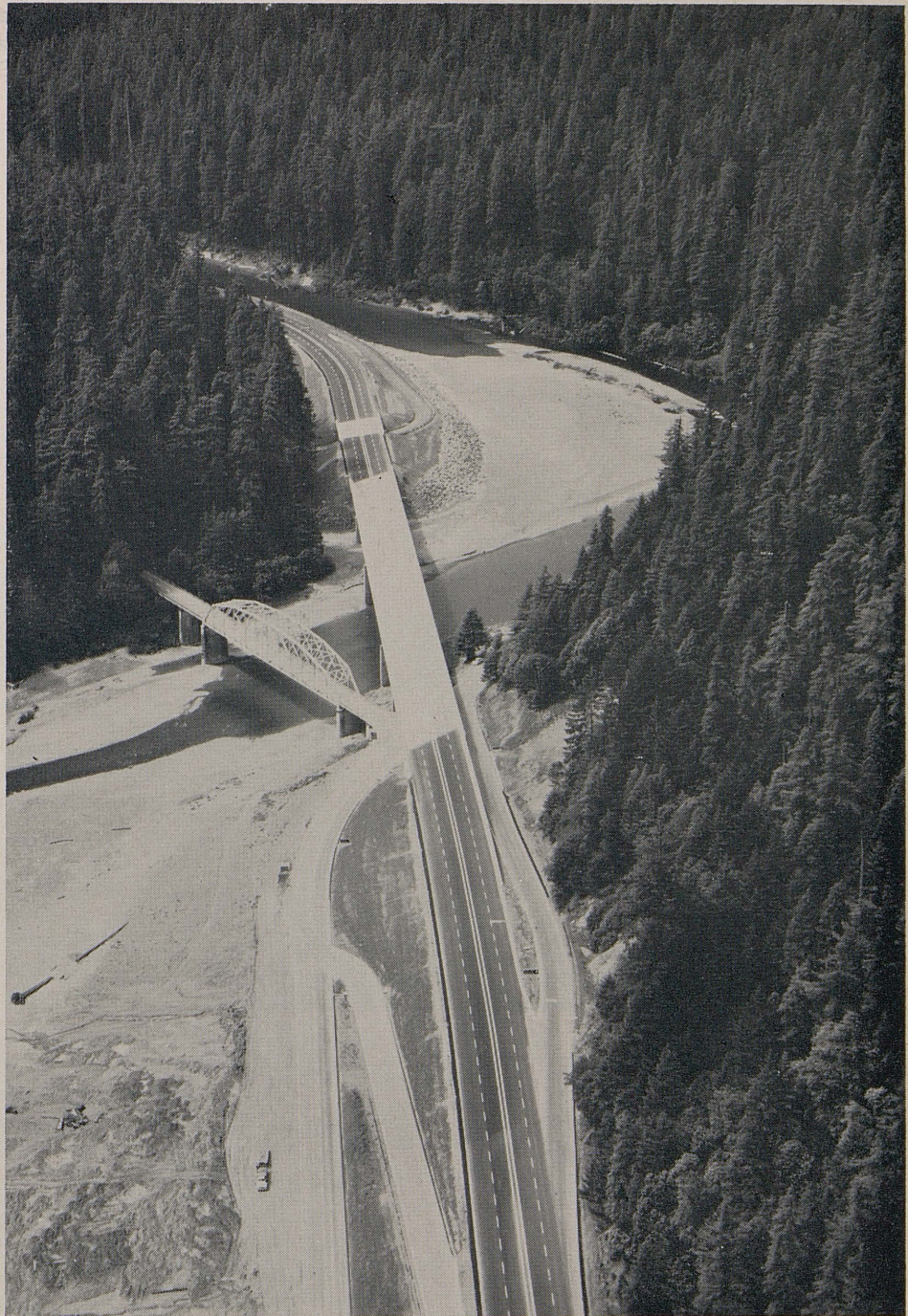
A view southward showing the new George M. Leatherwood Memorial Bridge on the recently completed first unit of the Redwood Parks Freeway (US 101) at Dyerville in Humboldt County. The old highway bridge can be seen to the left of the new one. (See photo on page 25.)
