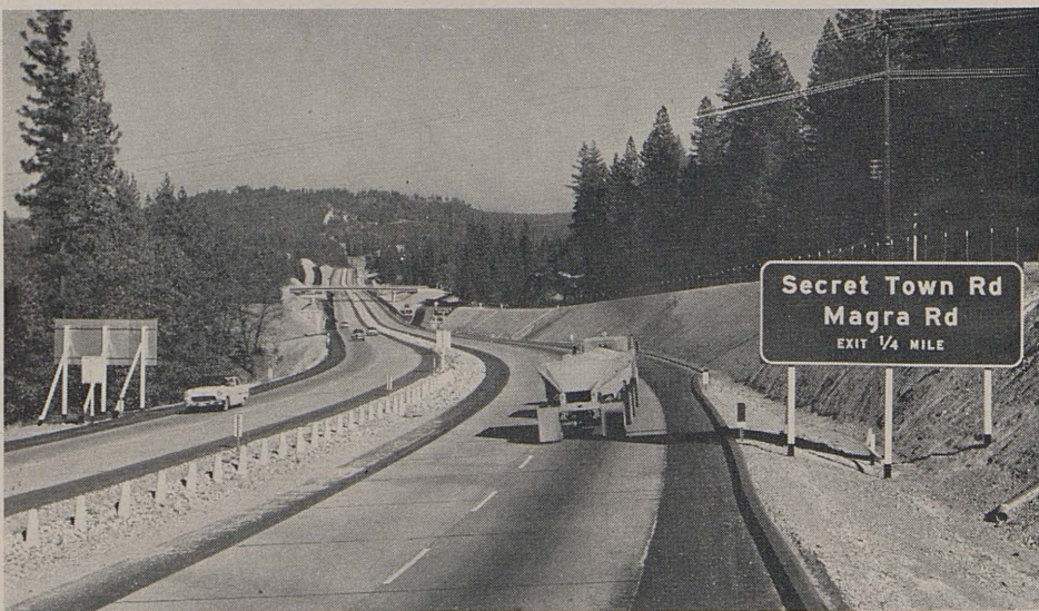
Recently opened new section looking east toward Magra Overhead.
