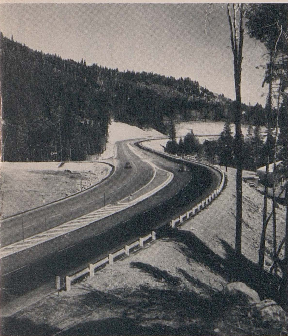
MAIN COVER —Recently completed expressway construction on U.S. 99 north of Shasta Lake. The channelized intersection will ultimately be replaced with an interchange when this section is developed to a full freeway under the Interstate Program. The orange snow markers have been placed for the winter season to guide the snowplow operators. (See Report From District II, page 12.)
