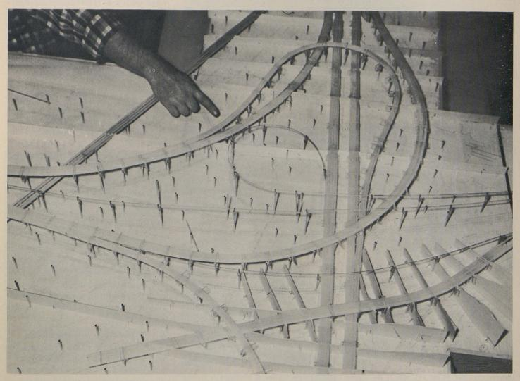
Use of plastic strips for roadways and "T" pegs for supports permits extreme flexibility of design.
