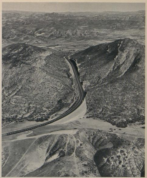
An aerial looking northward showing the 84-foot rock cut and the 85-foot embankment involved in the highway reconstruction.
