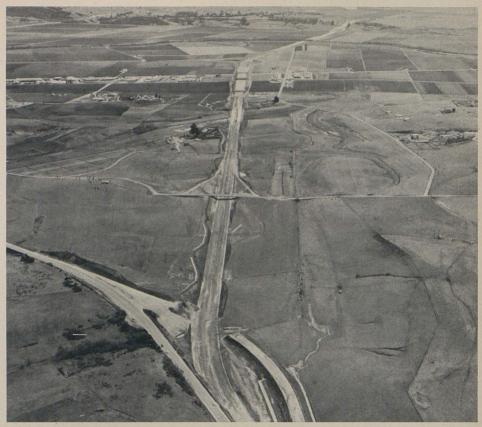
The first phase of construction on the Watsonville Bypass has been completed. For the next year the work will be allowed to stand while foundation materials settle; then the final phase of the work will be started. The view is southeast, toward Monterey County.
