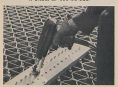
Studs were inserted in the gun from a holding board made by the crew to speed the operation.
