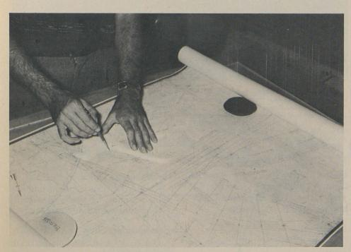
Transferring a shaped contour interval to a drawing.
