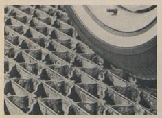
A view of the bridge deck after the studs had been welded giving a hobnail effect which greatly reduces skidding accidents.
