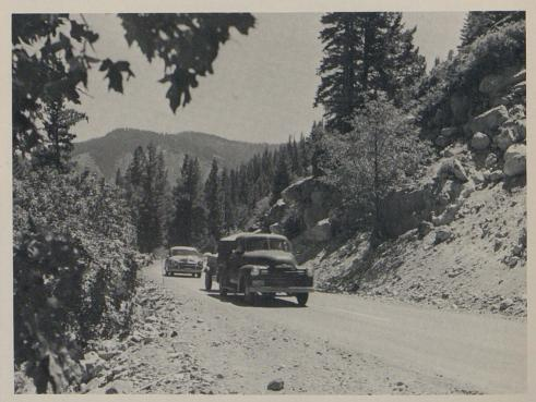
A typical section of the old highway before widening and improvement. Slope cuts (right) were through glacial material of round, loosely packed rocks which presented a tough maintenance problem of constant sloughing and falling rock resulting from the freeze-thaw cycle in winter and spring.
