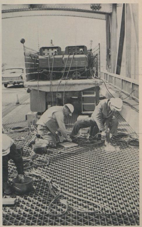
A state crew welds studs into the deck grid with battery-powered units set on truck.
