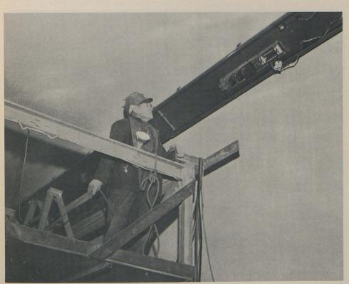
Caldecott Tunnel construction. After the walls were painted, new fluorescent strip lighting fixtures were installed. Here a workman inspects the ballast wiring for a strip section.
