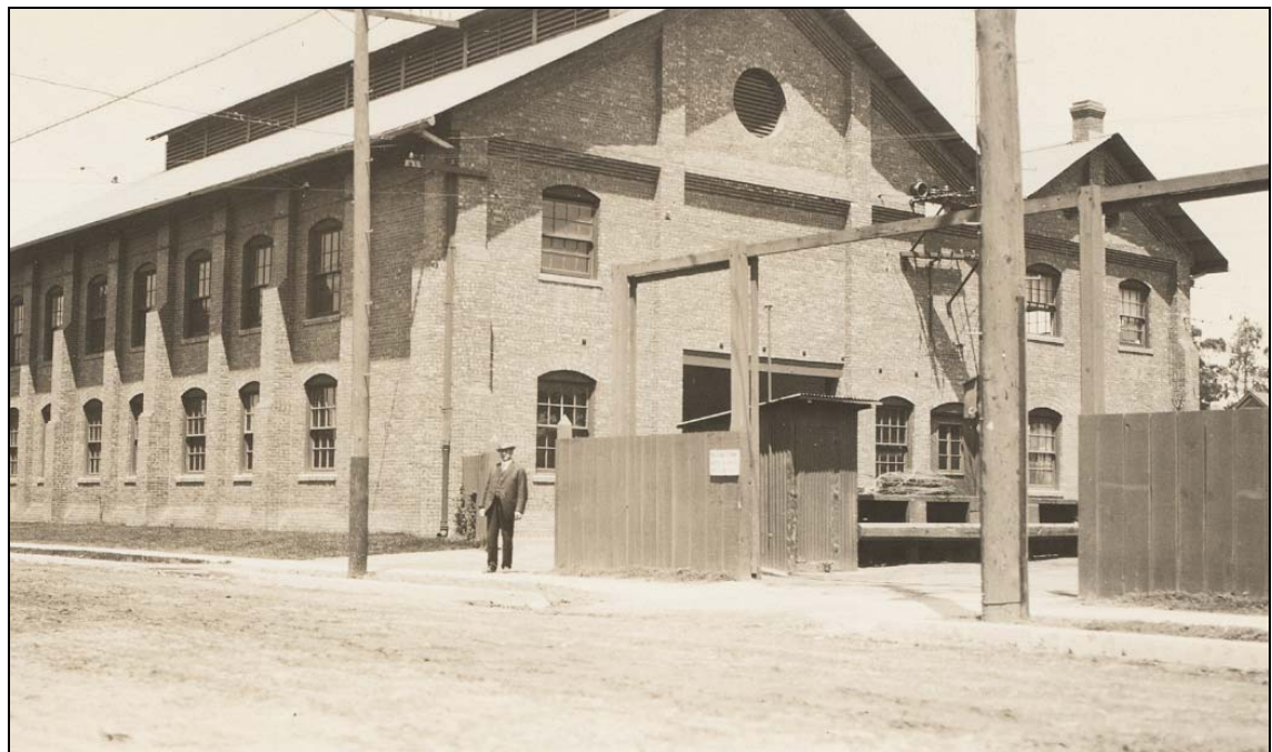
Figure 5. LARy 16 th Street Substation, demolished by RTD in the 1970s 12
