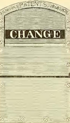
Change Gate. Outside View.
