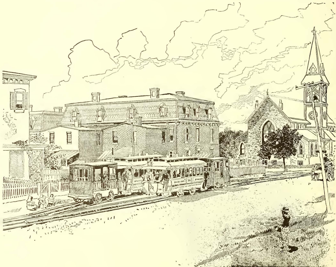
THE DAFT ELECTRIC STREET RAILWAY SYSTEM IN OPERATION AT BALTIMORE, MD.
