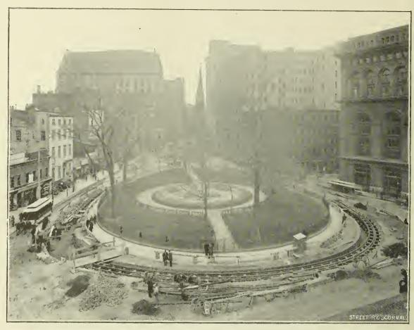
FIG. I.—BOWLING GREEN LOOP—BROADWAY CABLE RAILWAY.
