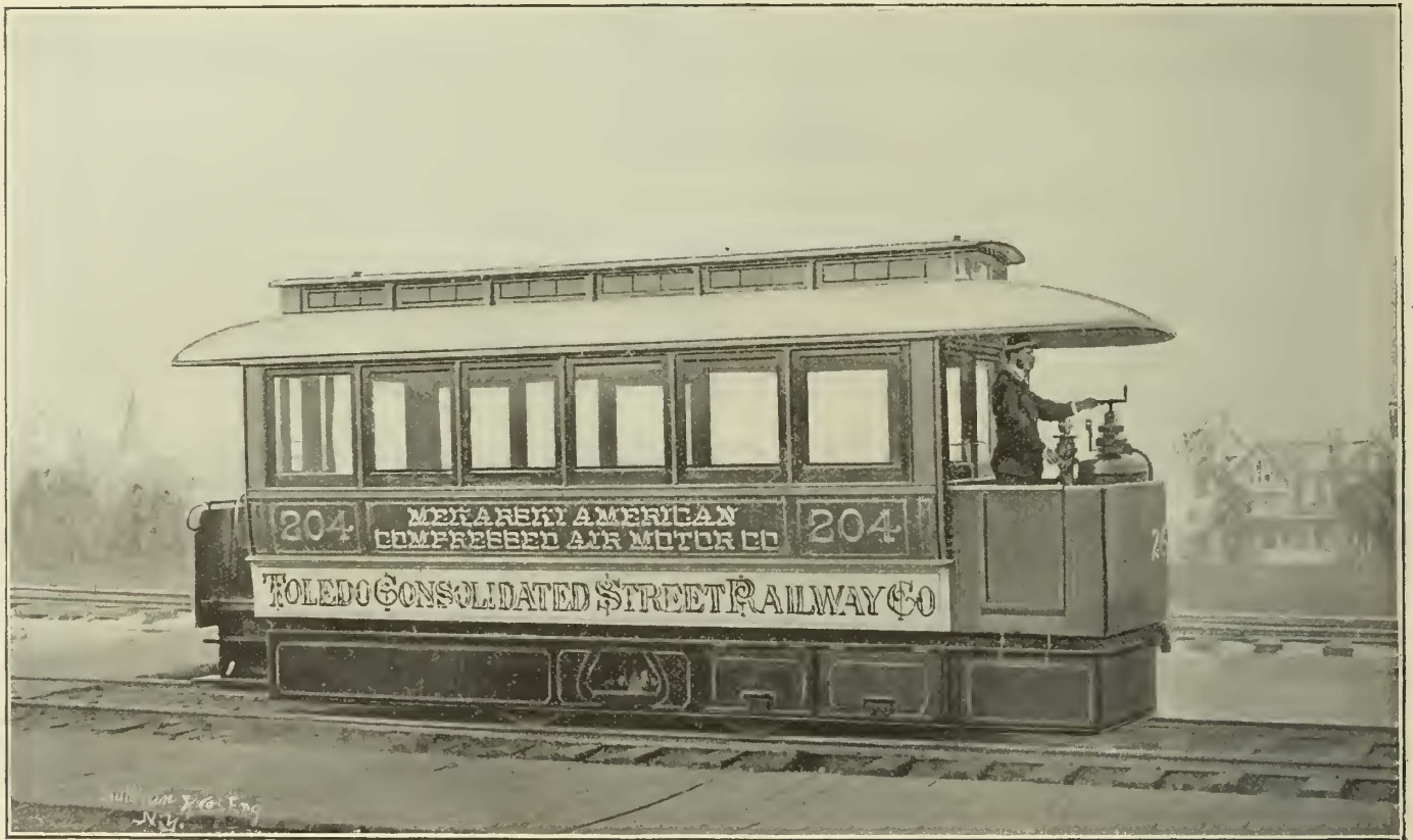
FIG. 1.—MEKARSKI COMPRESSED AIR MOTOR CAR—TOLEDO CONSOLIDATED STREET RAILWAY CO.
