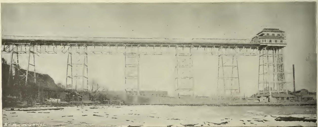
VIEW FROM RIVER—WEEHAWKEN VIADUCT.
