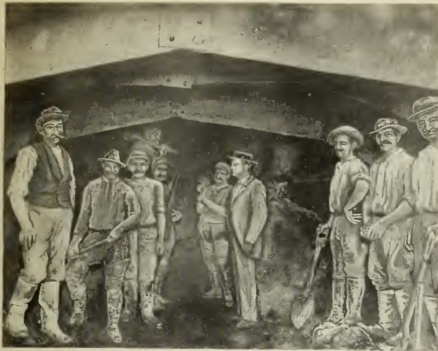
FIG. 5.—INTERIOR OF TUNNEL—BALTIMORE BELT RAILWAY.
