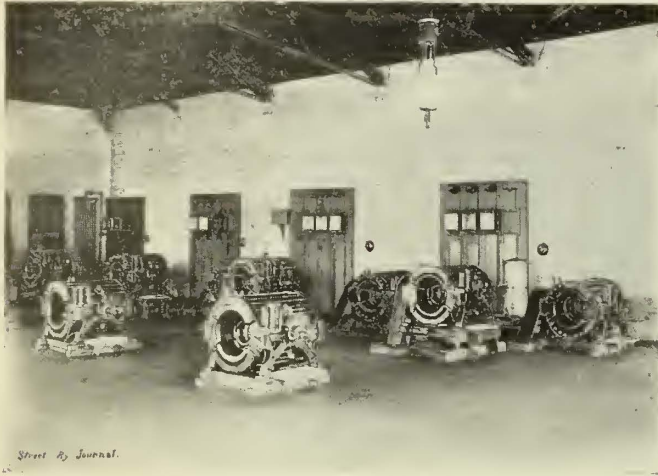
CHICAGO AVENUE ELECTRIC LIGHT STATION—DYNAMO ROOM.
