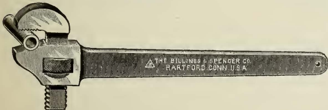
FIG. 2.—PIPE WRENCH.
