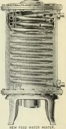
contraction is wholly obviated by the use of this spiral coil. The increased area of the shell above that of the exhaust wholly obviates any chance of causing back pressure on the engine; instead it causes a slight vacuum, thereby giving immediate relief to the engine. In fact, it is not neces-
