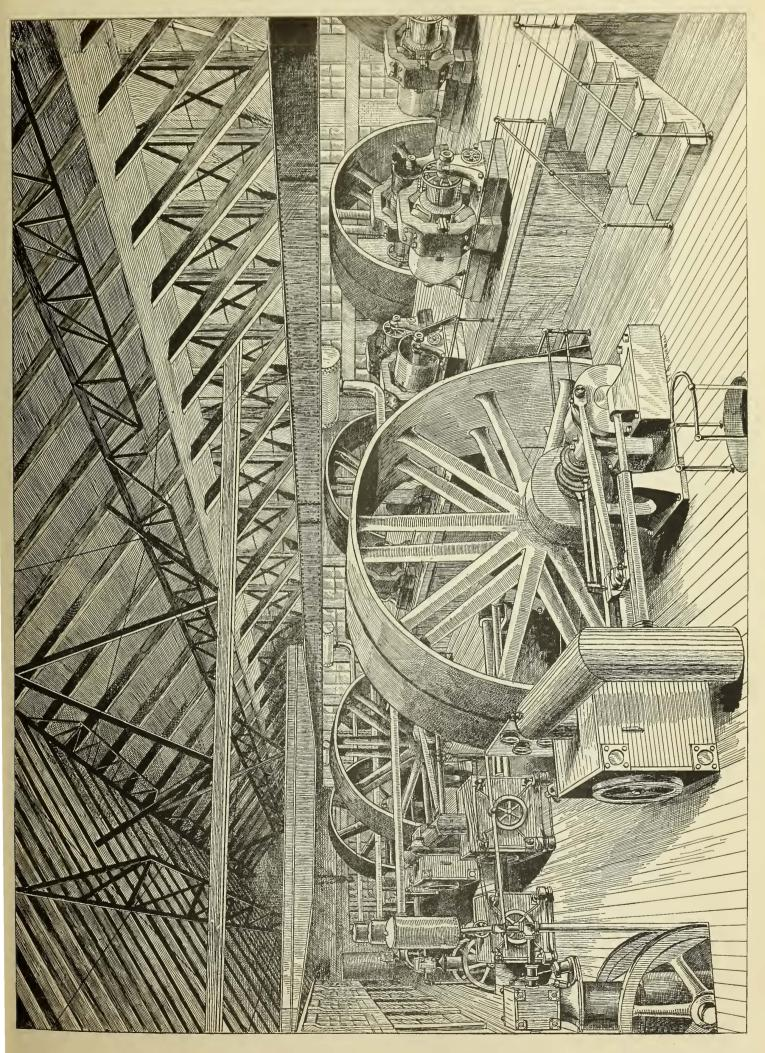
leading to the engines are in duplicate throughout, and the mains are led along near the roof over the generator floor (Fig. 1), from which the connections to each engine curve down, and pass under the truss to the high pressure cylinder, a separator being located in each at the point of entering the engine room proper.
