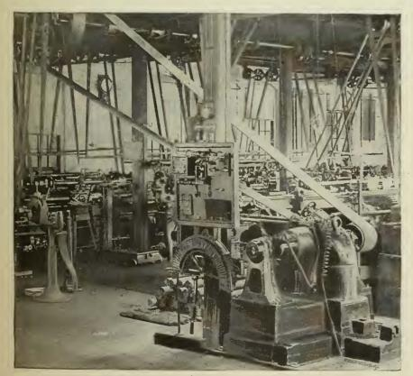
FIG. 16,-STATIONARY MOTOR DRIVING SHAFTING.
