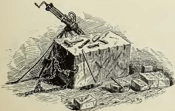
FIG. 11.—STEAM DRILL AND OTHER TOOLS EMPLOYED FOR CUTTING GRANITE.
