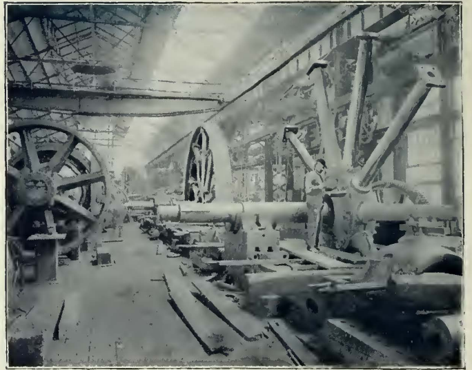
BUILDING UP A THIRTY TWO FOOT CABLE DRIVING DRUM.
