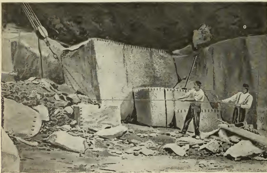
FIG. 5.—HOISTING THE BLOCKS FROM THE QUARRY.
