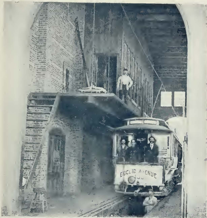
TROLLEY AND MOTOR INSPECTION ROOM—EAST CLEVELAND RAILROAD CO.
