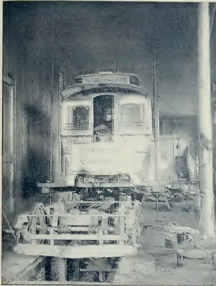
MOTOR REPAIR SHOP—BROADWAY & NEWBURGH STREET RAILROAD CO.
