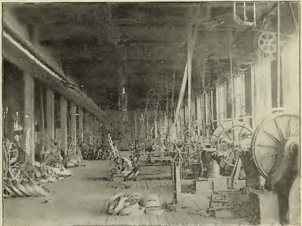
FIG. 2.—VIEW OF PULLEY ROOM—FALLS RIVET & MACHINE CO.'S WORKS.
