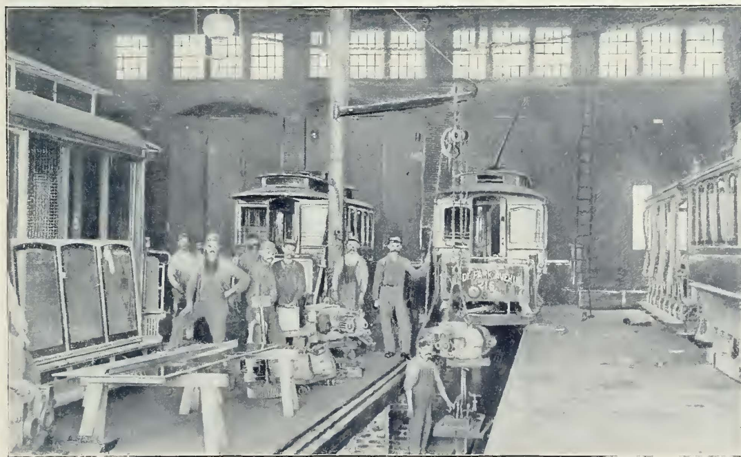
MOTOR REPAIR SHOP—EAST CLEVELAND RAILROAD CO.
