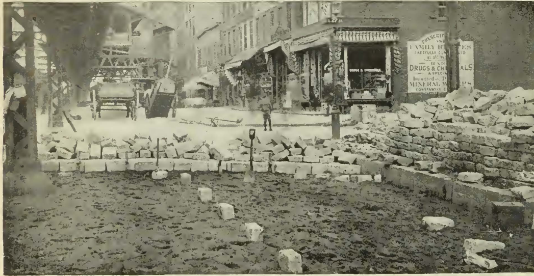
FIG. 8.—FINAL STAGE—PLACING THE BLOCKS IN THEIR LITTLE BED.
