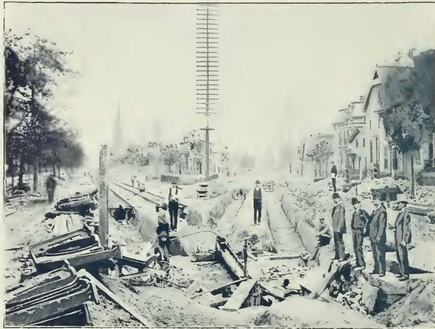
STREET SCENE DURING THE CONSTRUCTION OF THE CABLE LINES.
