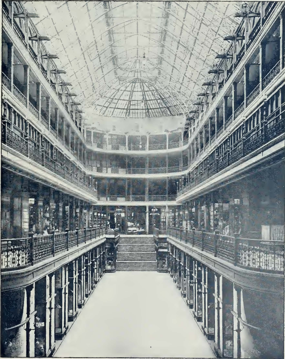
INTERIOR OF THE ARCADE BUILDING.
