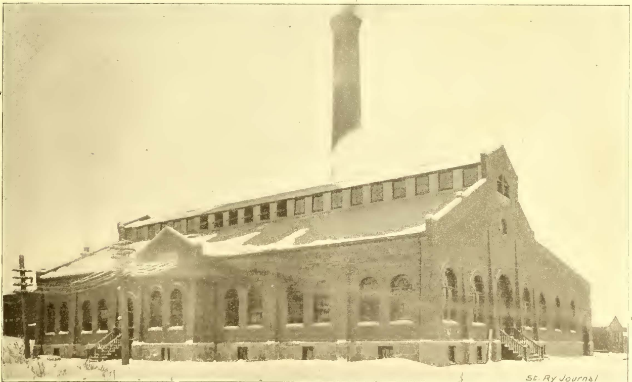
FIG. 3.—EXTERIOR OF SALEM POWER STATION—LYNN & BOSTON RAILROAD CO.
