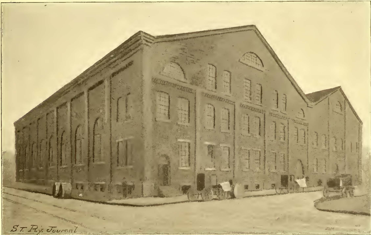
FIG. 1.—EXTERIOR OF 13TH STREET STATION—PHILADELPHIA TRACTION CO., PHILADELPHIA, PA.
