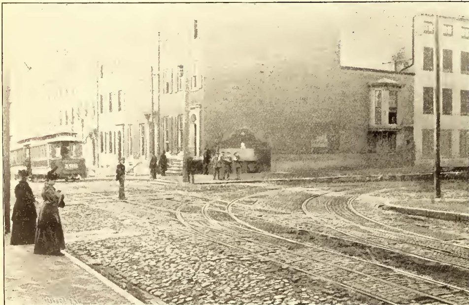
FIG. 5.—JUNCTION OF CABLE LINES—BALTIMORE TRACTION CO.
