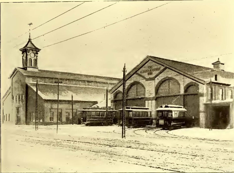
FIG. 4.—EXTERIOR OF CAR HOUSE—ALBANY RAILWAY.
