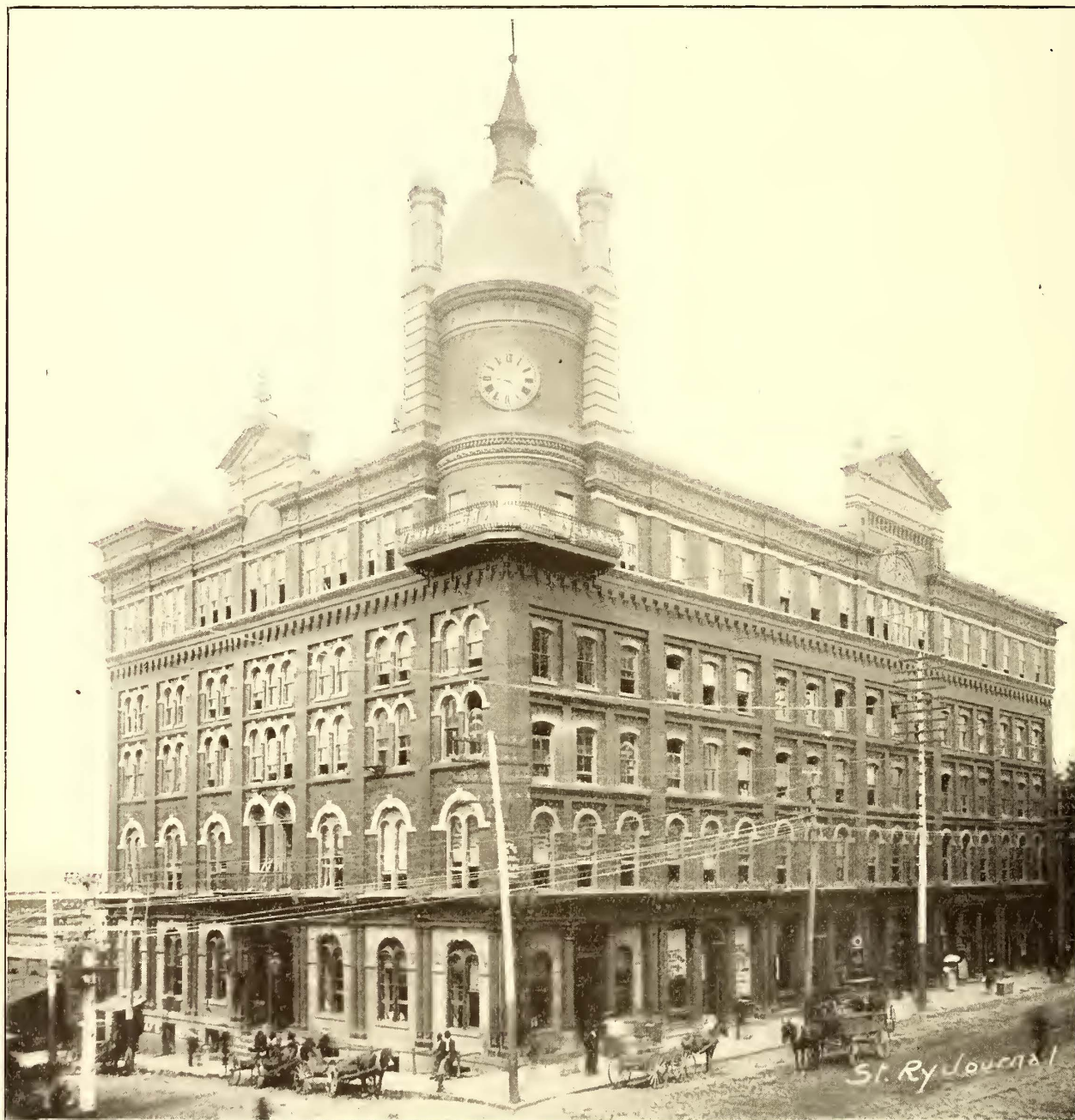
FIG. 14.—OLD CAPITOL BUILDING—ATLANTA, GA.
