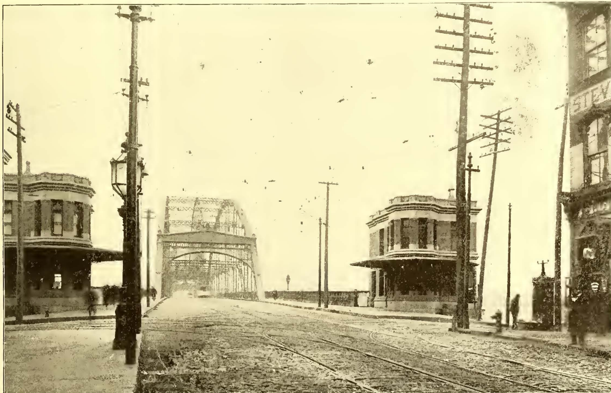
FIG. 1—NEAT OVERHEAD WIRING—PITTSBURGH, ALLEGHENY & MANCHESTER TRACTION CO.
