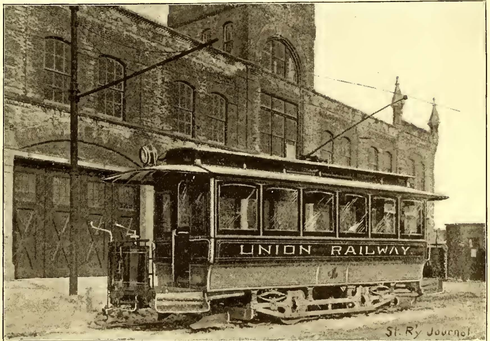
FIG. 2.—CAR EQUIPPED WITH TWIN SERIES MOTOR—UNION RAILWAY, NEW YORK CITY.
