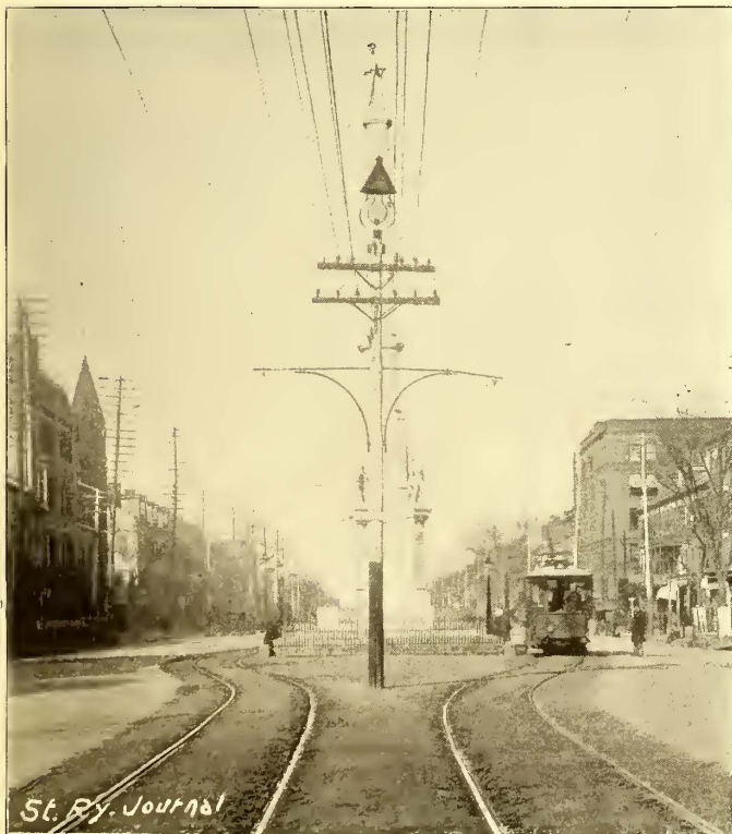
FIG. 4.—CONFEDERATE MONUMENT, CORNER BROAD AND JACKSON STREETS, SHOWING BRICK PAVEMENT BETWEEN TRACKS—AUGUSTA, GA.
