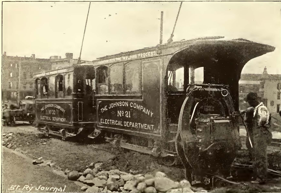
FIG. 1.—RAIL WELDING EQUIPMENT—NASSAU ELECTRIC RAILWAY, BROOKLYN.
