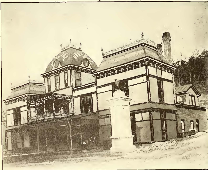
FIG. 2.—ONE OF THE BATH HOUSES—HOT SPRINGS, ARK.
