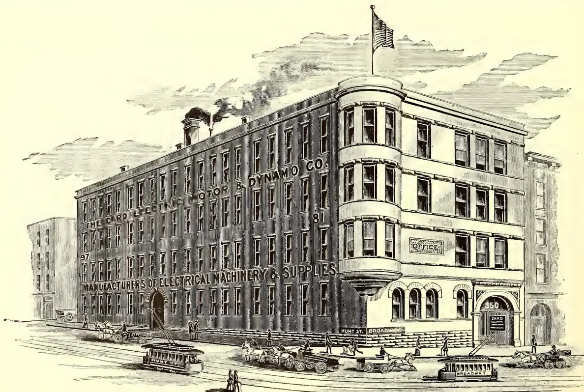
FIG. 1.—WORKS OF THE CARD ELECTRIC MOTOR & DYNAMO CO., CINCINNATI.
