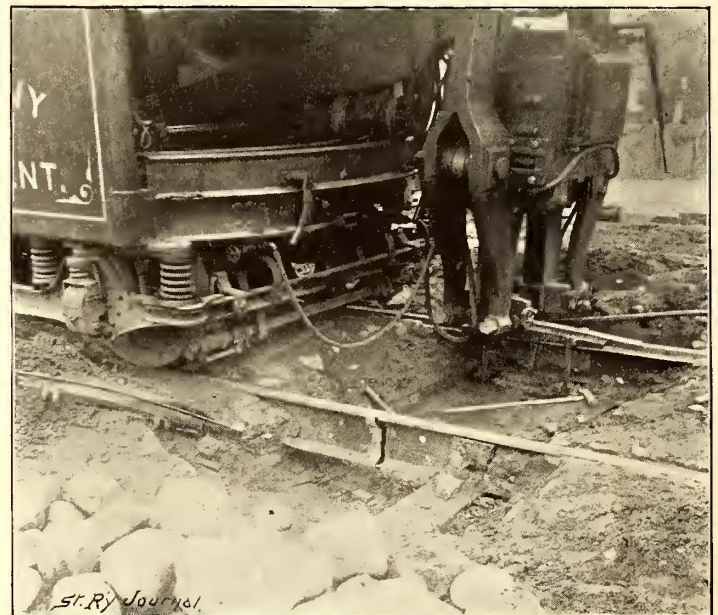
FIG. 3.—METHOD OF WELDING RAILS.
