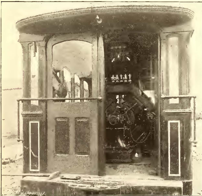
FIG. 2.—INTERIOR OF TRANSFORMER CAR—BROOKLYN.
