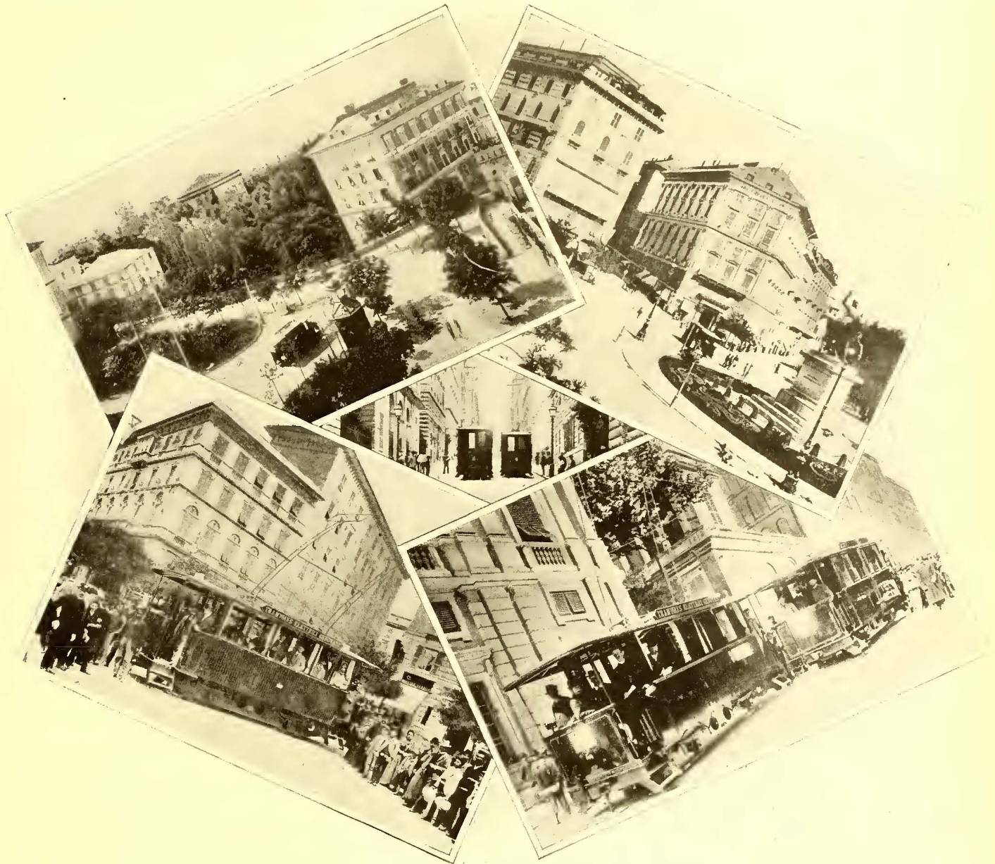
FIG. 2.—VIEWS ON THE LINE OF THE GENOA ELECTRIC RAILWAY.
