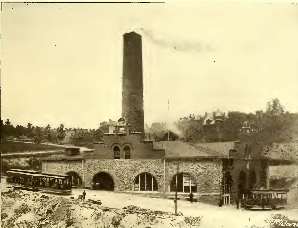
FIG. 12.—POWER STATION—MT. AUBURN CABLE RAILWAY CO., CINCINNATI.
