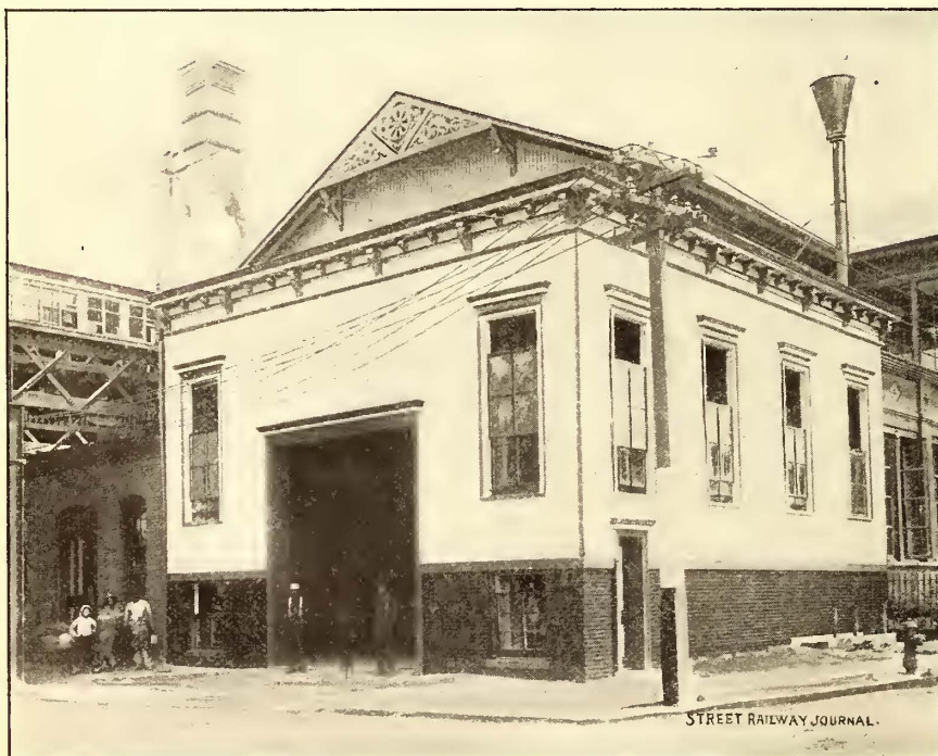
FIG. 1.—PATROL HOUSE—NORTH HUDSON COUNTY RAILWAY, HOBOKEN.
