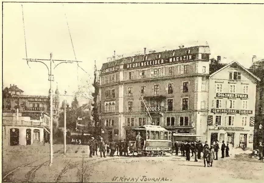
FIG. 1.—VIEW AT THE KREUZPLATZ—ZURICH ELECTRIC RAILWAY.
