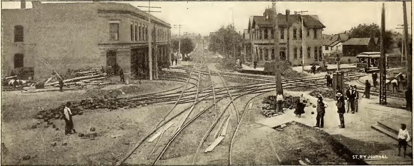
VIEW DURING CONSTRUCTION OF FARWELL AVENUE CROSSING, MILWAUKEE.
