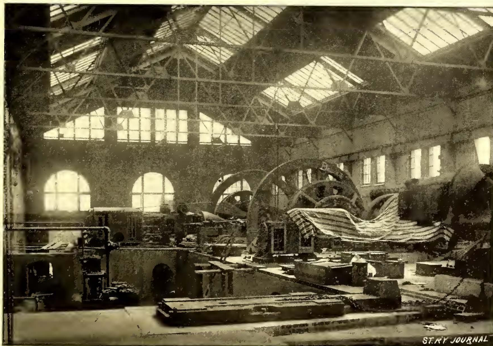
FIG. 7.—INTERIOR OF DELAWARE AVENUE POWER STATION—ELECTRIC TRACTION CO., PHILADELPHIA.
