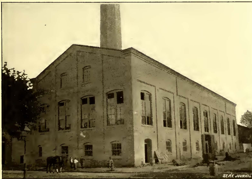
FIG. 1.—EXTERIOR OF DAUPHIN STREET POWER STATION—PHILADELPHIA TRACTION CO.
