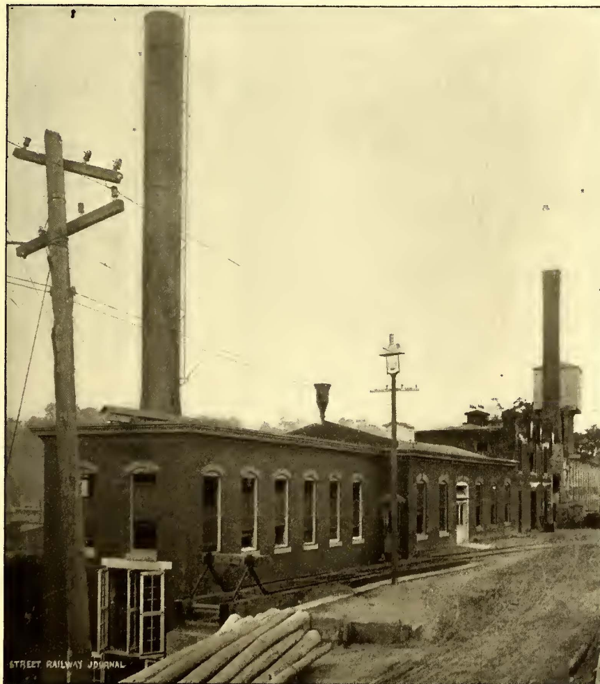
FIG. 3.—EXTERIOR OF STATION—WISSAHICKON ELECTRIC PASSENGER RAILWAY CO.
