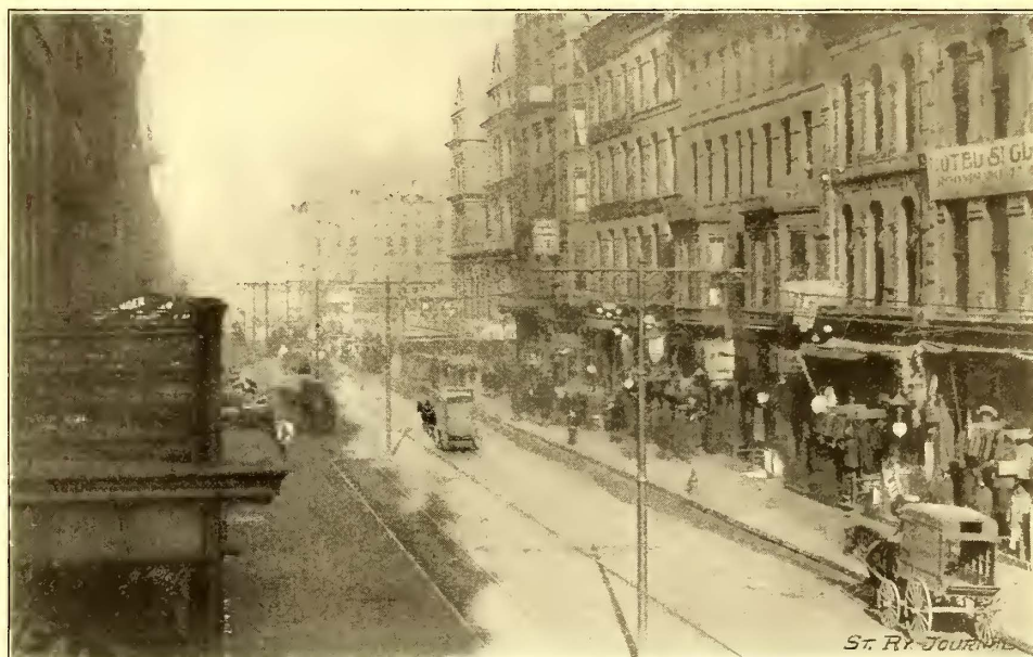
ELECTRIC CONSTRUCTION ON CLARK STREET, CHICAGO.
