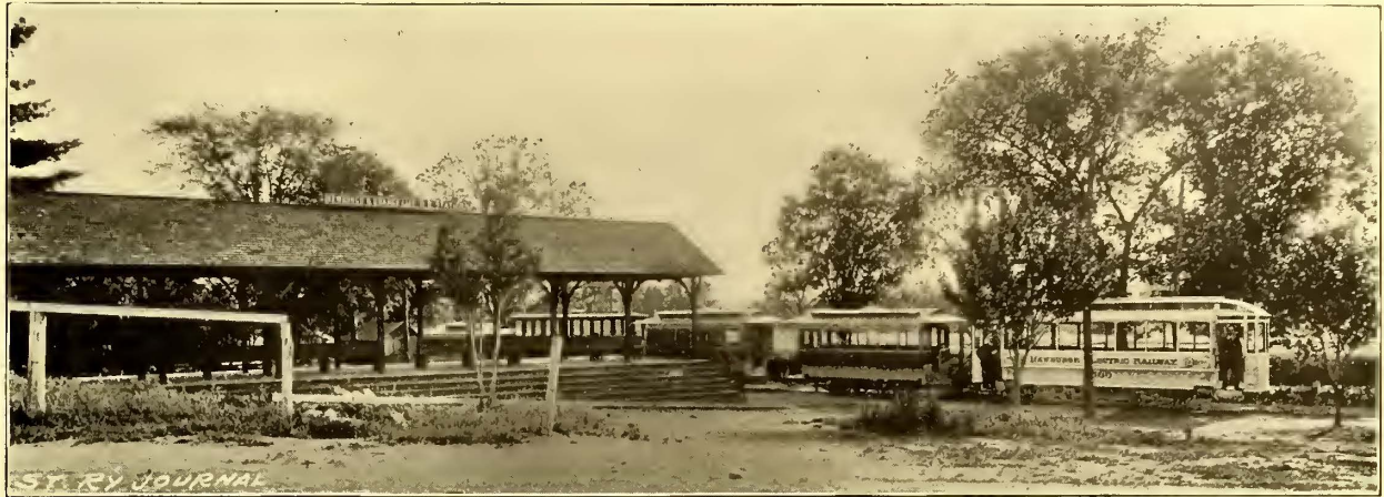
FIG. 13.—CAR HOUSE AT ORANGE LAKE—NEWBURGH ELECTRIC RAILWAY.
