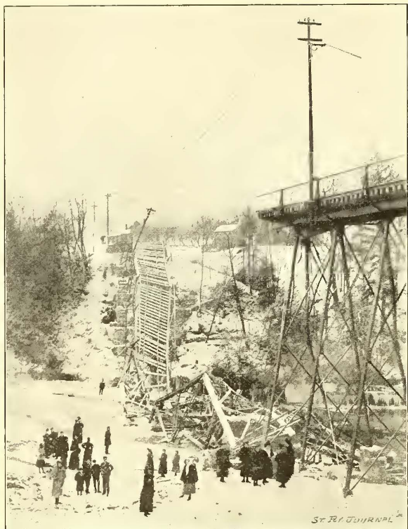
FIG. 7.—BRIDGE ACROSS TINKER'S CREEK AFTER THE DISASTER.
