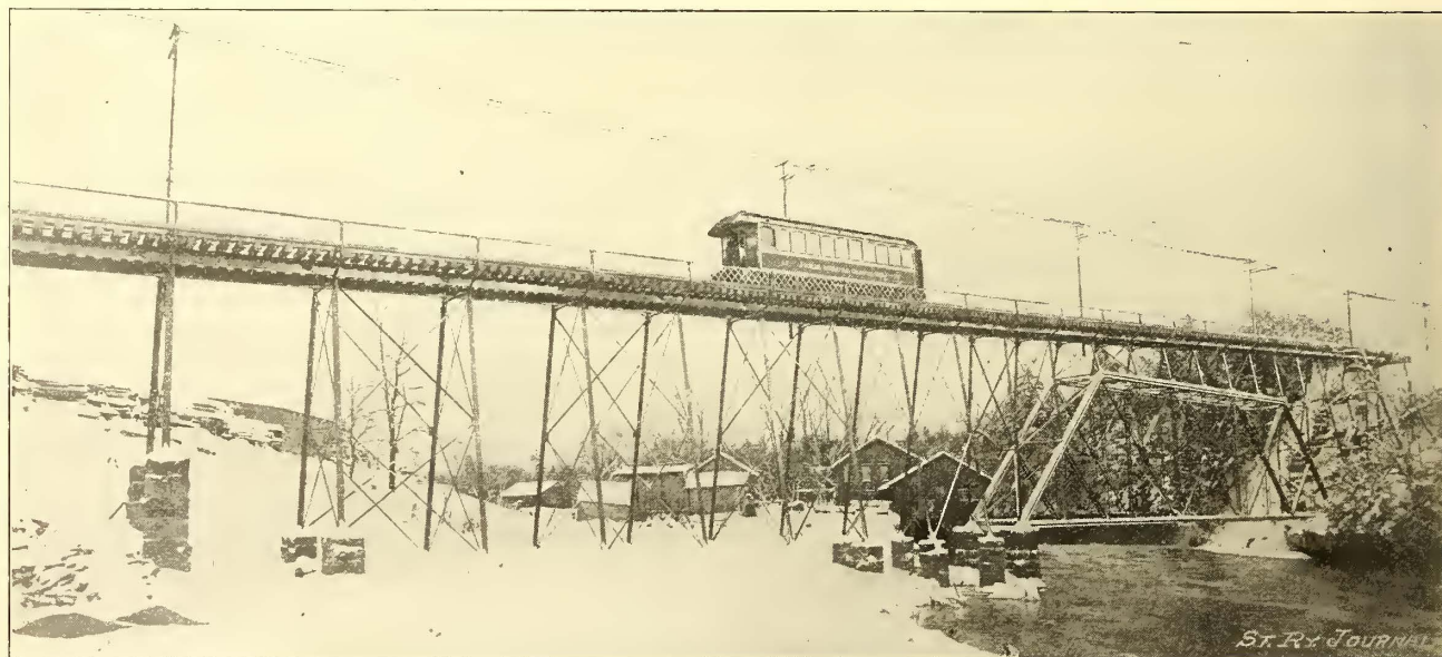
FIG. 8.—BRIDGE ACROSS TINKER'S CREEK BEFORE THE DISASTER.
