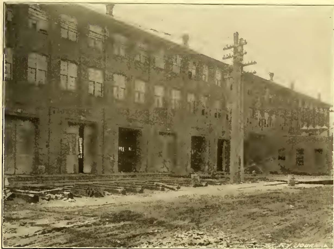
FIG. 1.—EXTERIOR OF CENTRAL REPAIR SHOP—WEST END STREET RAILWAY.
