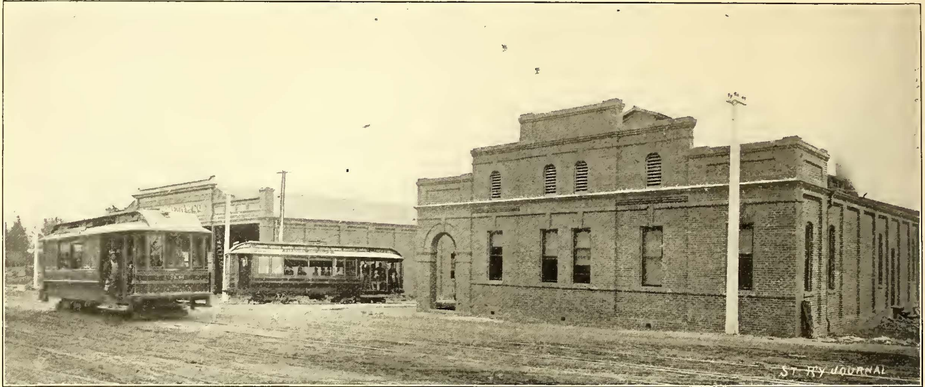
FIG. 15.—POWER STATION AND CAR HOUSE—PASADENA & PACIFIC ELECTRIC RAILWAY.
