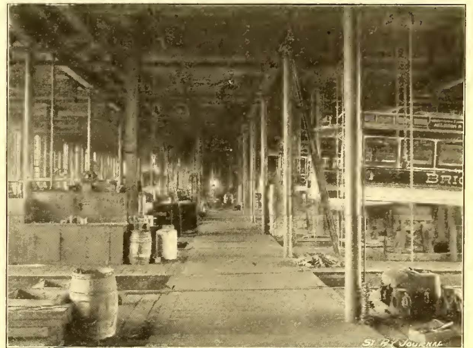
FIG. 7.—VIEW IN EQUIPMENT ROOM—WEST END RAILWAY.
