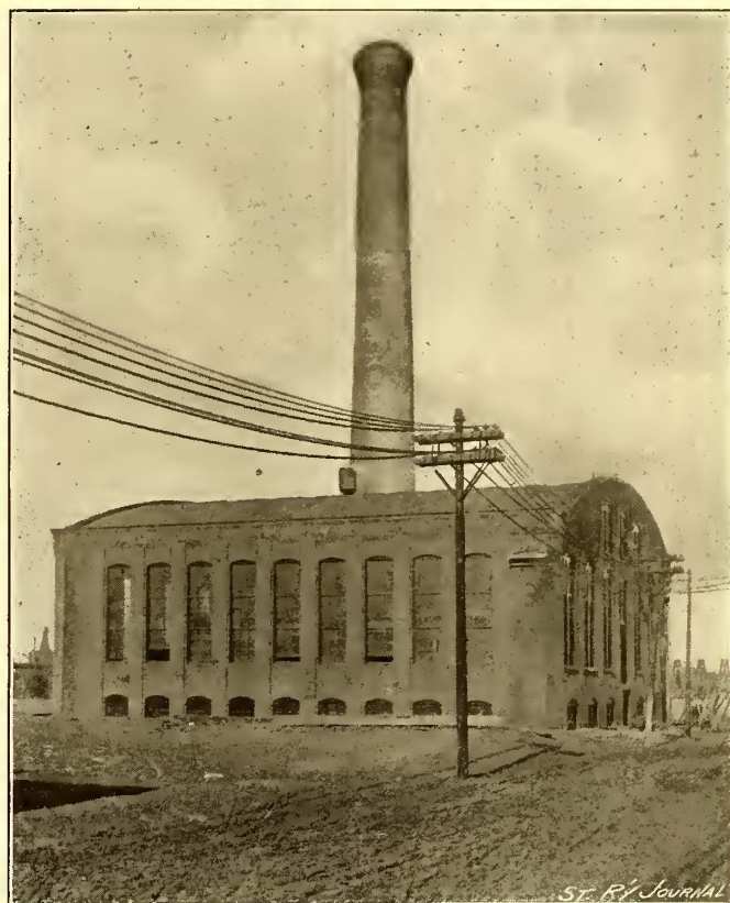
FIG 1.—EXTERIOR OF CHARLESTOWN STATION
