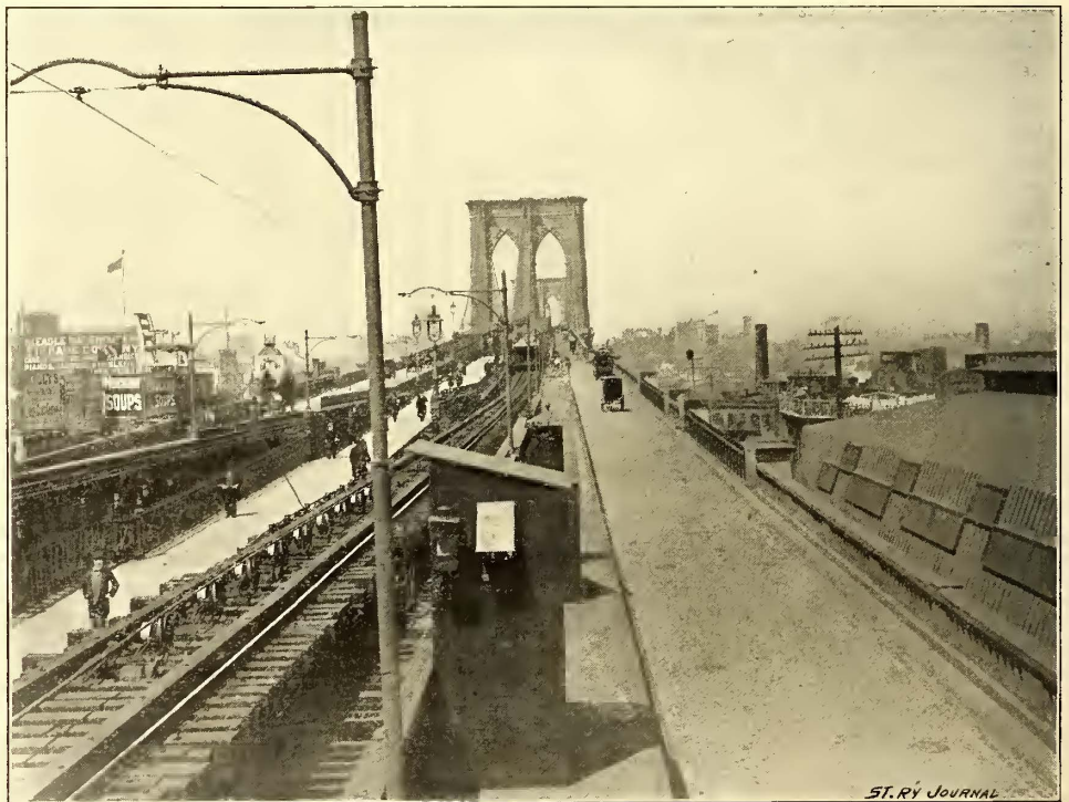
FIG. 2.—VIEW OF TILTING SHEAVES AND OVERHEAD WIRE SYSTEM ON BROOKLYN BRIDGE.
