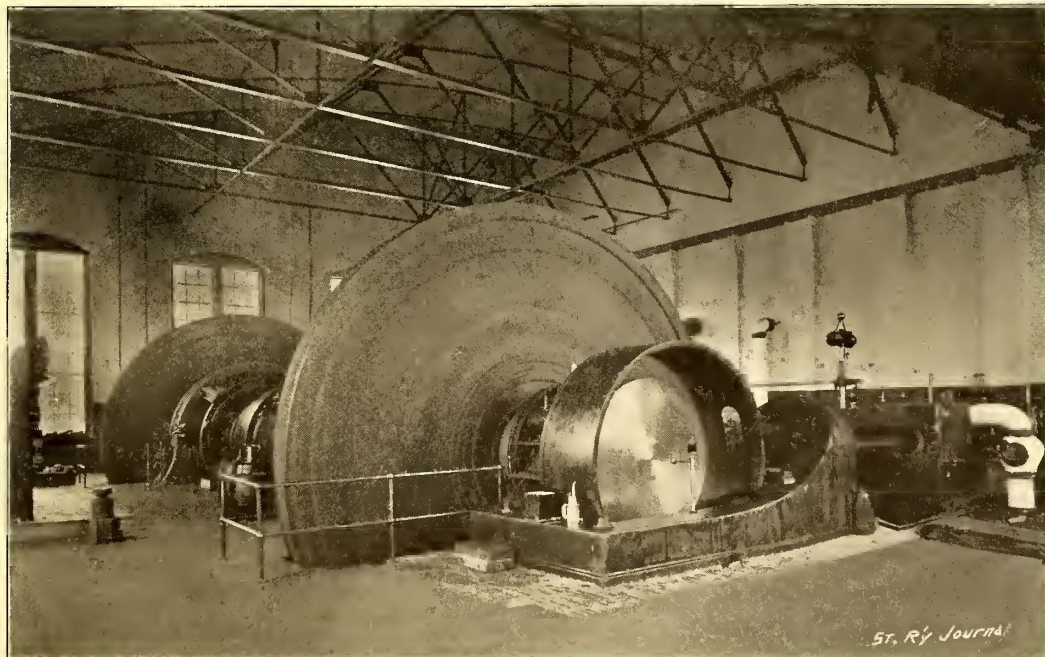
FIG. 2.—INTERIOR OF STATION, SHOWING PLATE FLYWHEELS IN MOTION.
