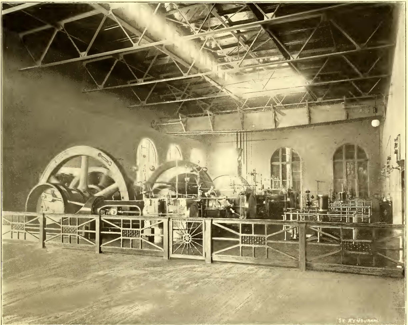
FIG. 1.—INTERIOR OF POWER STATION—PORTLAND RAILROAD CO.
