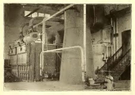
FIG. 14.-INTERIOR OF BOILER ROOM, SHOWING DUPLICATE PIPING.
