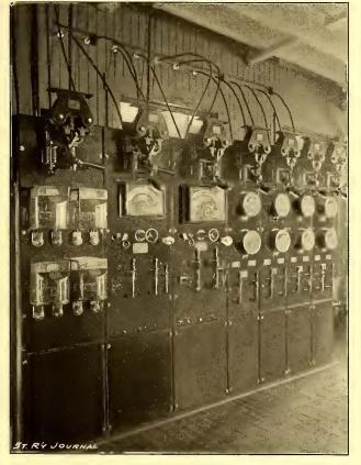
FIG. 1.—SWITCHBOARD WITH FOUR WATTMETERS— MANCHESTER
