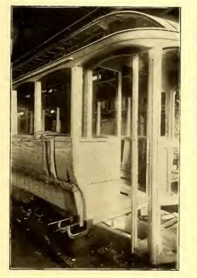
FIG. 2.--METHOD OF PUTTING PANELS IN PLACE,
