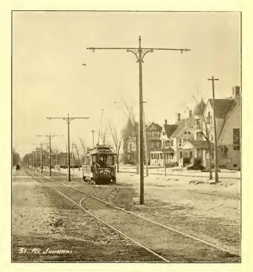
FIG. 2.—DOUBLE BRACKET CONSTRUCTION—MANCHESTER.
