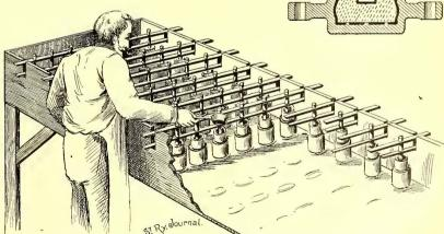
FIG. 2.—METHOD OF ASSEMBLING INSULATORS.
