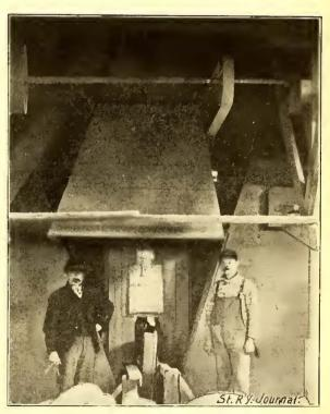
FIG. 6.—CLEANING WHEELS BY SAND BLAST.
