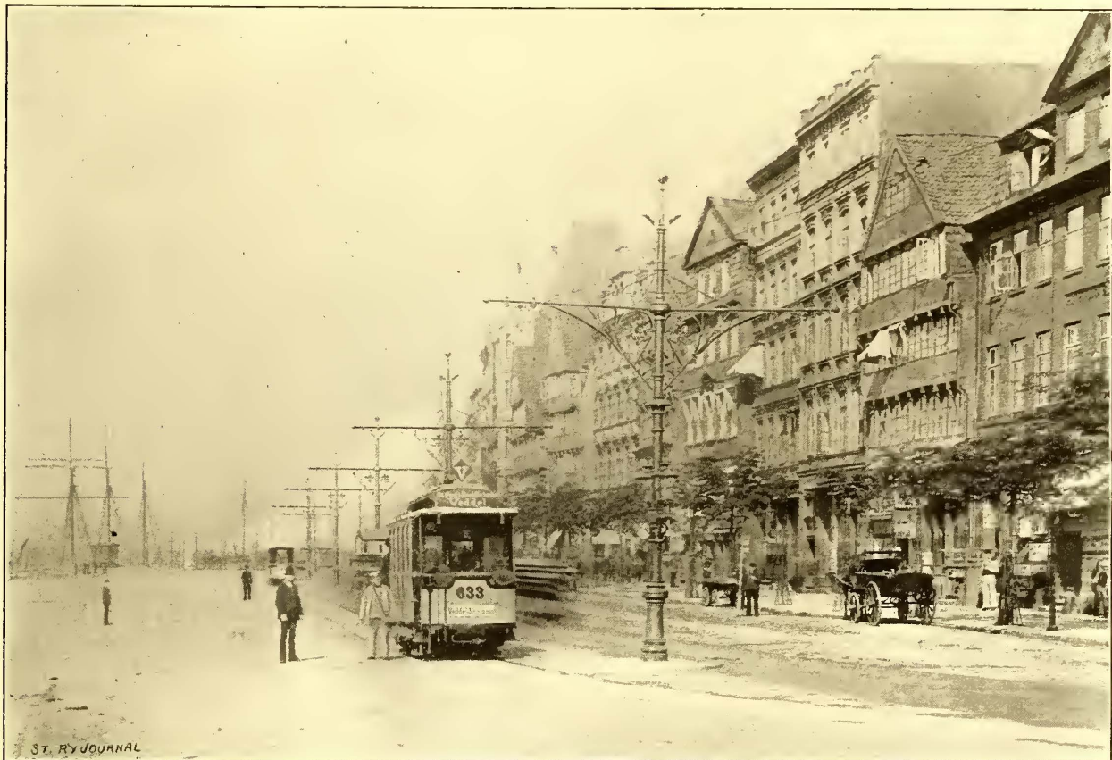
HANDSOME CENTER POLE CONSTRUCTION IN HAMBURG.
