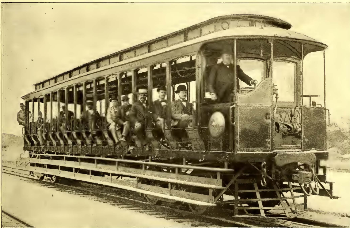
FIG. 2.—CAR OPERATING ON THIRD RAIL SYSTEM—NANTASKET.
