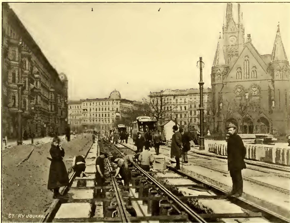
VIEW OF CONDUIT CONSTRUCTION IN BERLIN—SHOWING YOKES UNDER SIDE RAIL.
