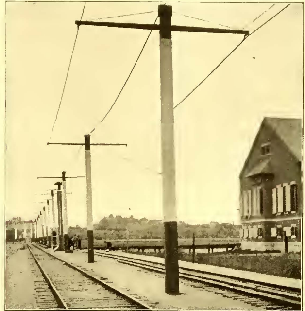
FIG. 1.—TRACK WITH OVERHEAD AND THIRD RAIL CONSTRUCTION.
