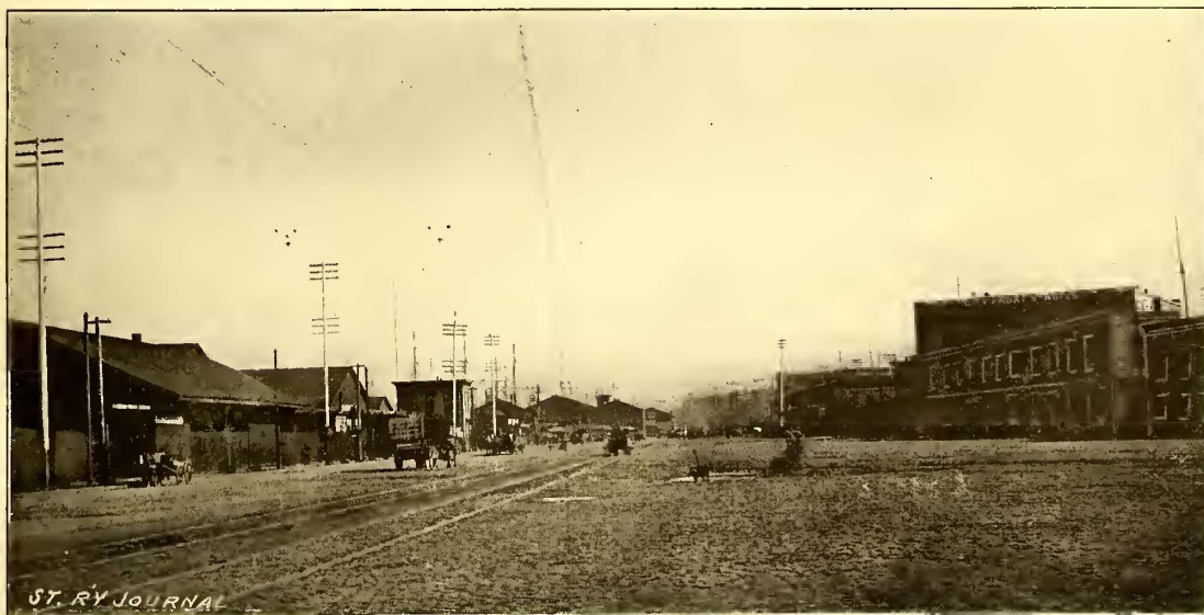
FIG. 4.—TWO HUNDRED FOOT SPAN CONSTRUCTION.
