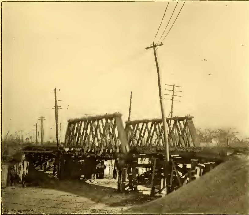
ELECTRIC RAILWAY TRESTLE AT ELBERON.
