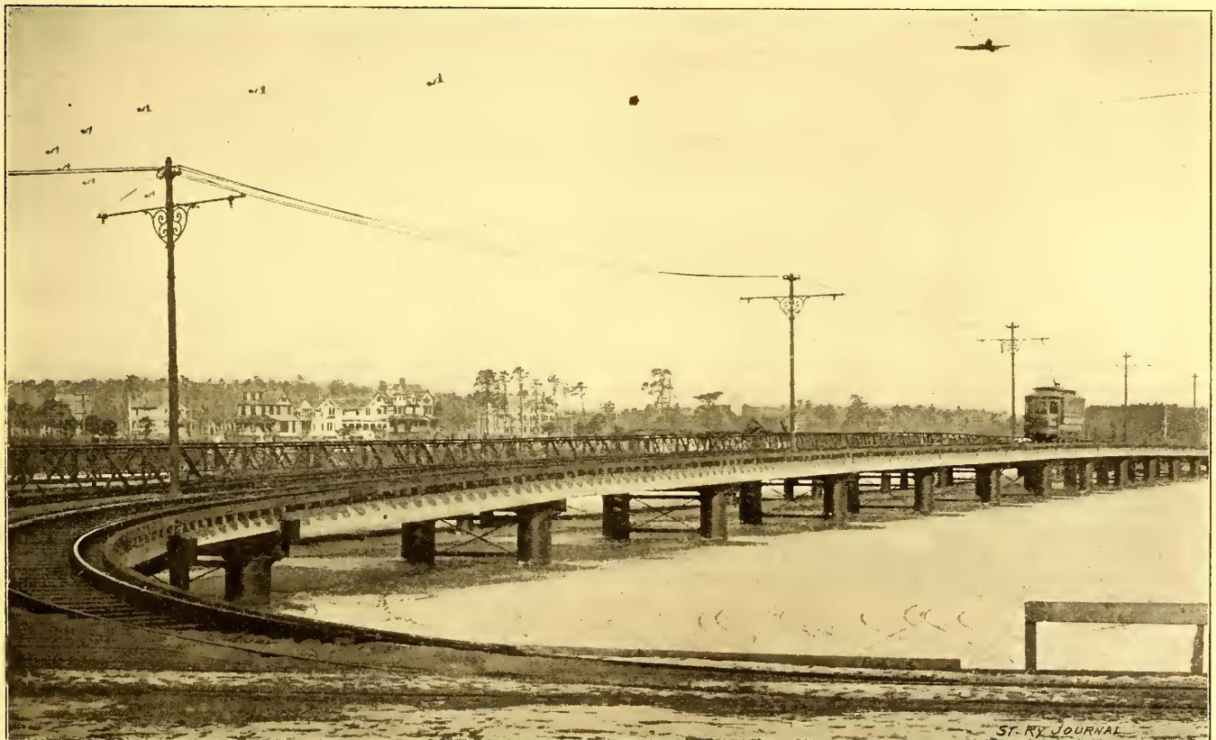
STEEL BRIDGE OVER DEAL LAKE.
