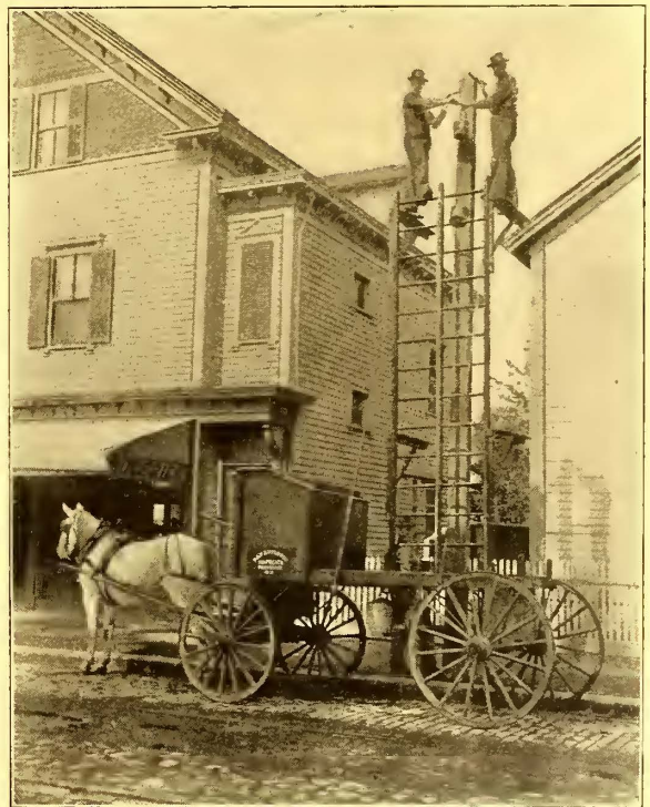
FIGS. 1 AND 2.—SECTION OF POLE PAINTING WAGON AND METHOD OF USING.
