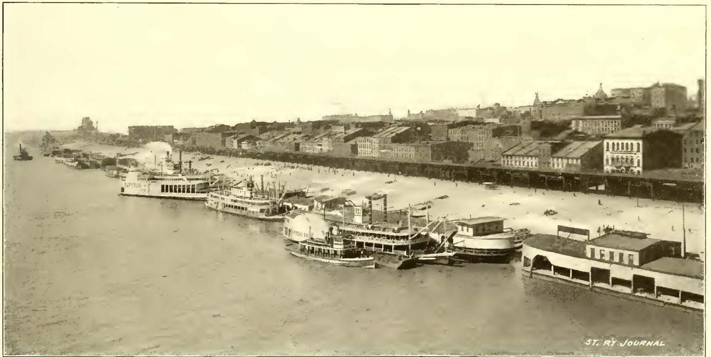
THE LEVEES OF THE MISSISSIPPI RIVER AT ST. LOUIS.
