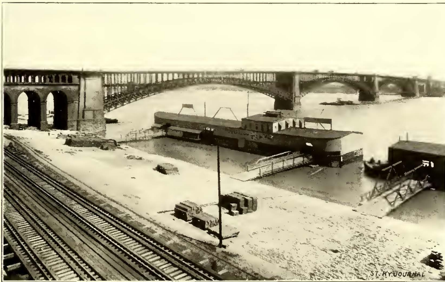
EADS BRIDGE FROM THE LEVEES.
