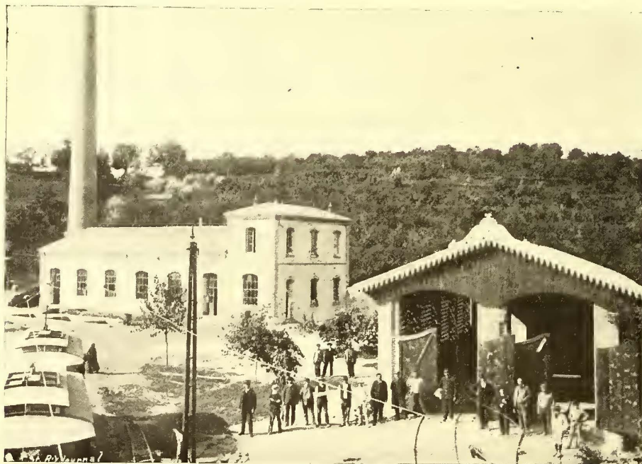
FIG. 2.—STATION AND CAR HOUSE AT ST. AMBROZIO.
