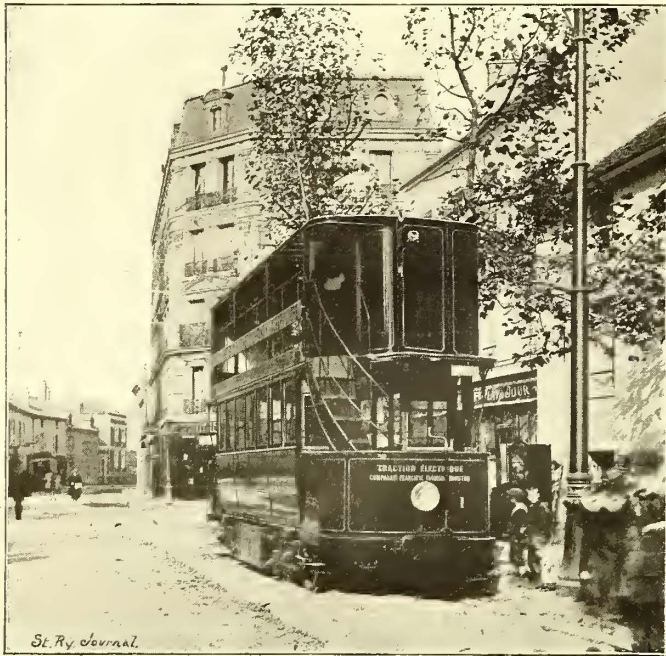
COMBINED STORAGE BATTERY AND TROLLEY CAR--PARIS
