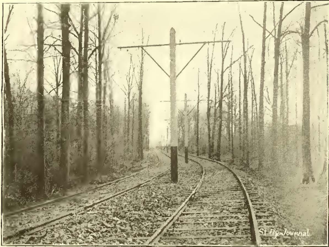
FIG. 2.—DOUBLE BRACKET CONSTRUCTION ON CURVE
