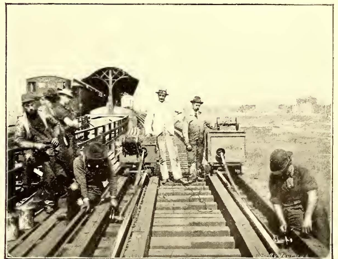
FIG. 4.—METHOD OF DRILLING RAILS
