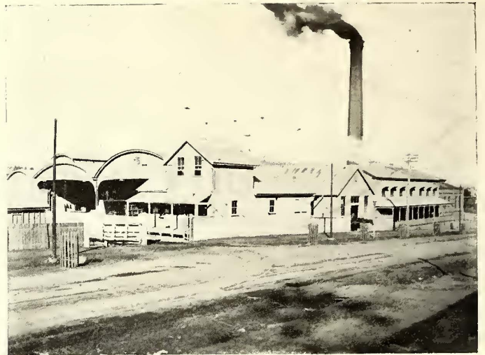
EXTERIOR OF POWER STATION
