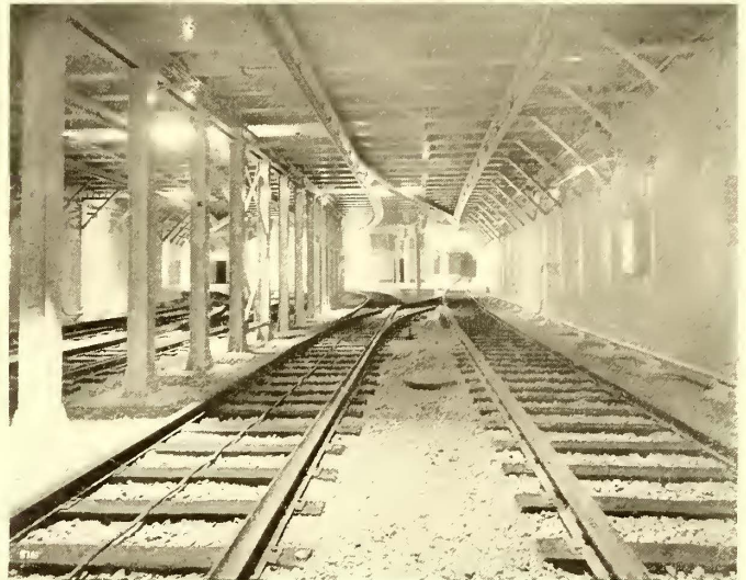
FOUR-TRACK SUBWAY STEEL WALL CONSTRUCTION
