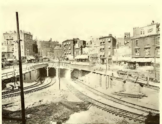
SHAWMUT AVENUE INCLINE
