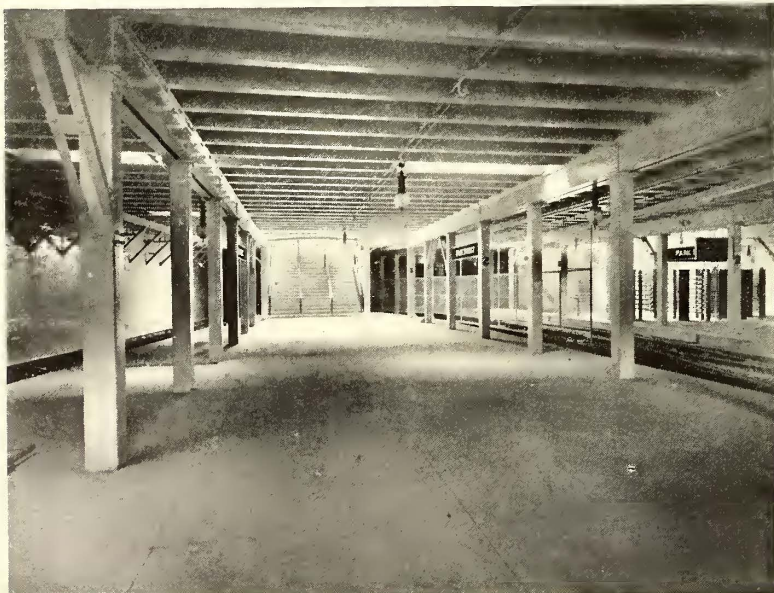
PARK STREET STATION
