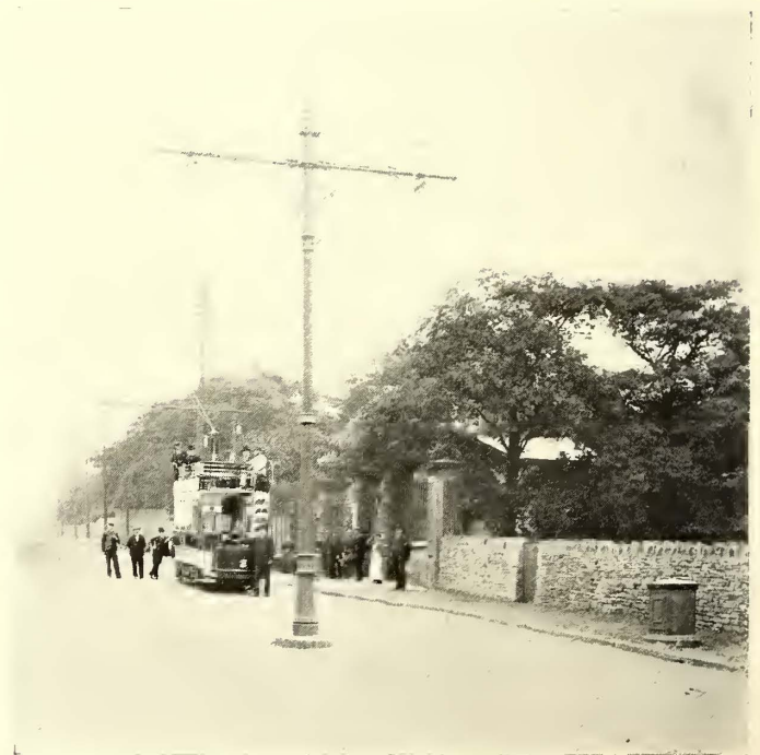
DOUBLE BRACKET CONSTRUCTION
