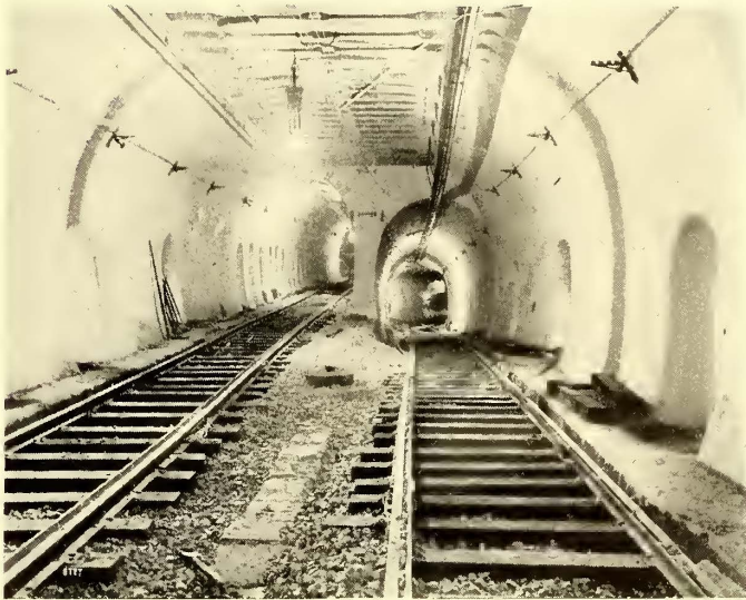
BELLMOUTHS UNDER TREMONT STREET, PASSAGE OF SOUTH-BOUND SHAWMUT AVENUE TRACK UNDER NORTH-BOUND TREMONT STREET TRACK
