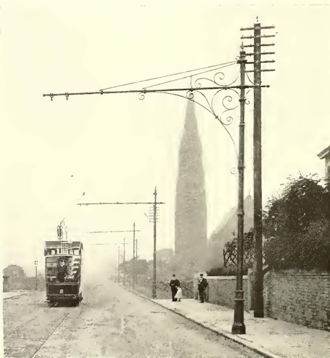
SINGLE BRACKET CONSTRUCTION
