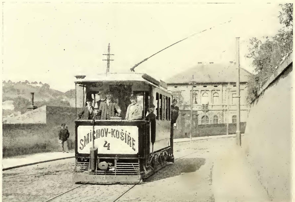
FIG. 1.—MOTOR CAR AT SMICHOV-KOSIRE, USING DICKINSON TROLLEY
