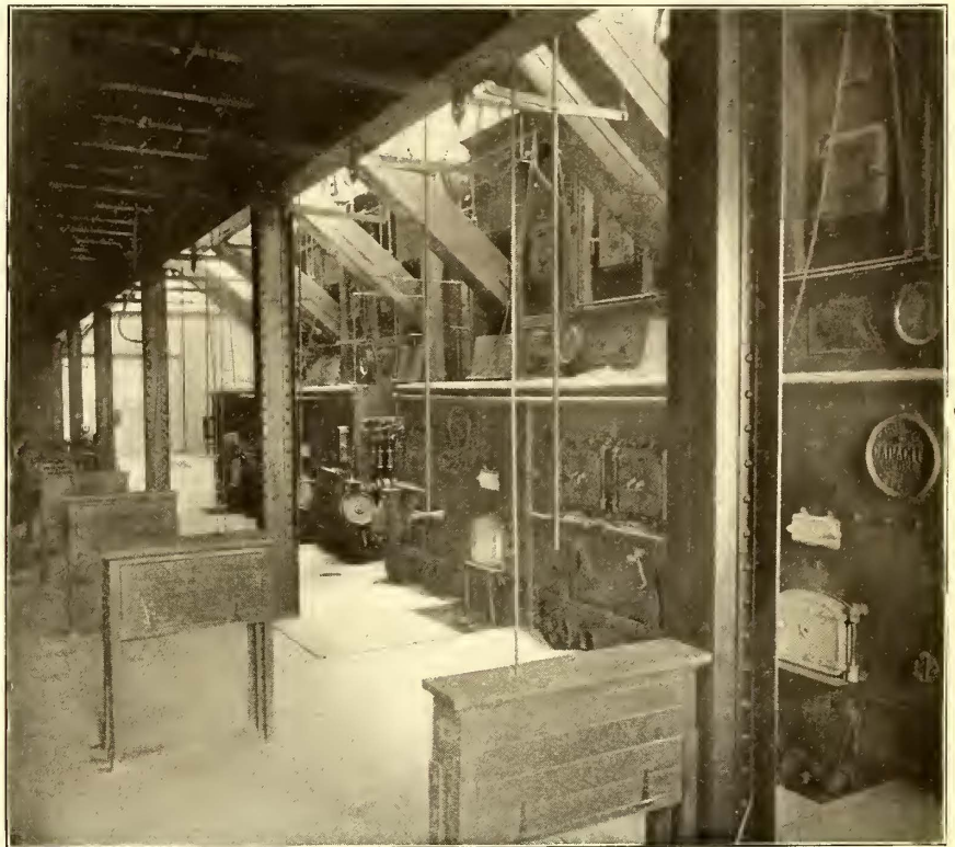
BOILER ROOM AND COAL SCALES
