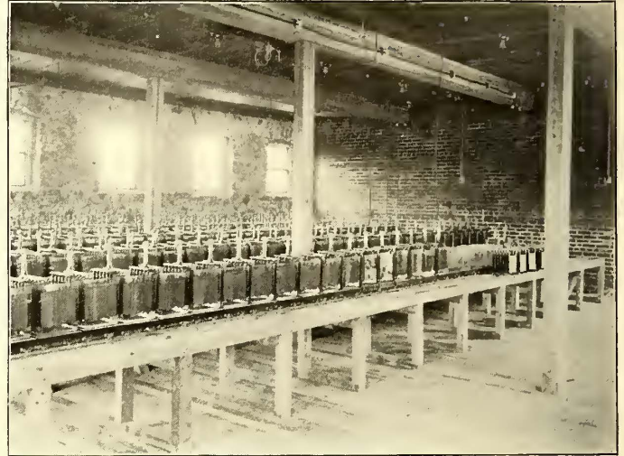
STORAGE BATTERY ROOM IN TRANSFORMER STATION
