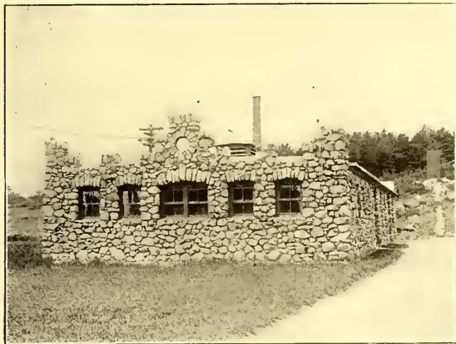
TRANSFORMER STATION AT WESTWOOD
