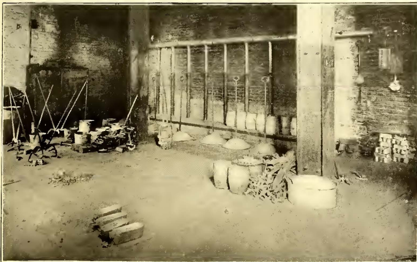
FIG. 6.—BRASS FOUNDRY, SHOWING INDIVIDUAL BLAST PIPE FOR EACH FURNACE PIT
