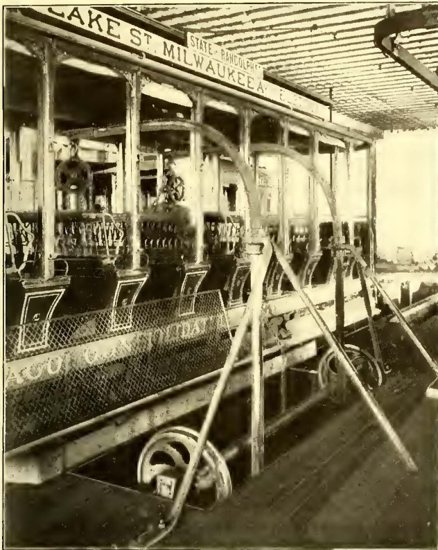
FIG. 4.—CRANE FOR LIFTING MOTORS FROM CAR ON TRANSFER TABLE
