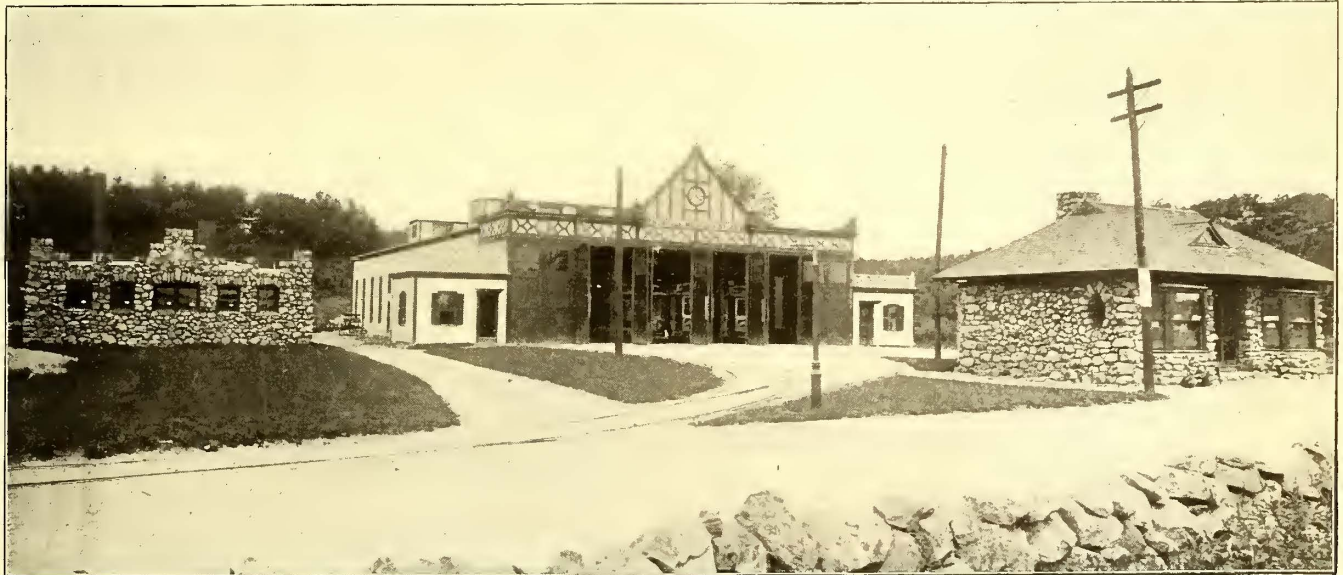
CAR HOUSE, TRANSFORMER STATION AND WAITING ROOM OF THE NORFOLK WESTERN STREET RAILWAY
