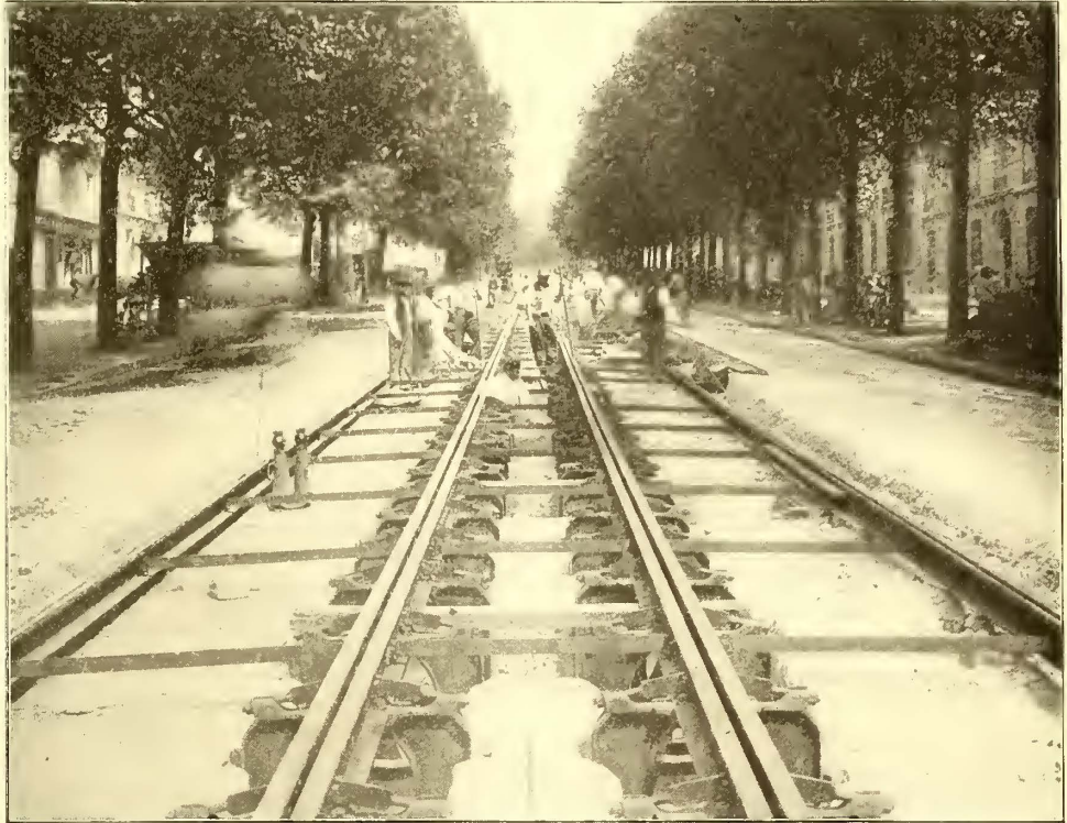
VIEW SHOWING CONDUIT LINE IN COURSE OF CONSTRUCTION
