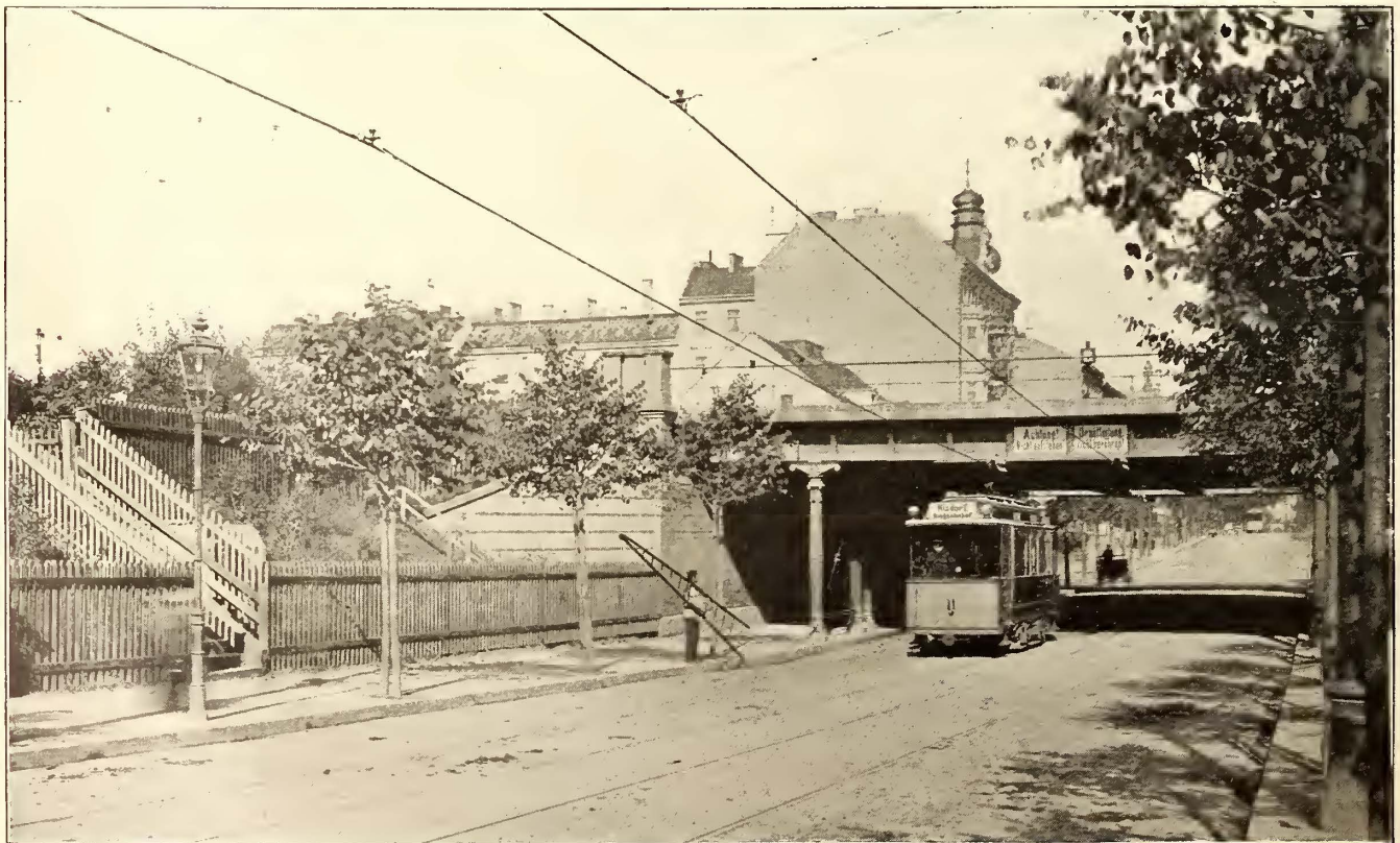
FIG. 11.—PASSING UNDER BRIDGE WITH 14 FT. 10 INS. HEADROOM
