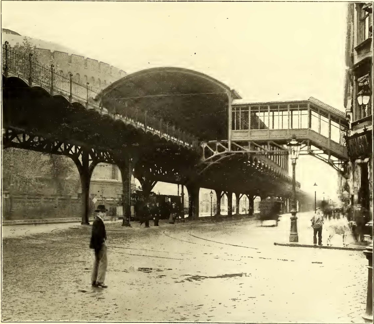
FIG. 3.—TYPICAL STATION, BERLIN ELEVATED RAILWAY
