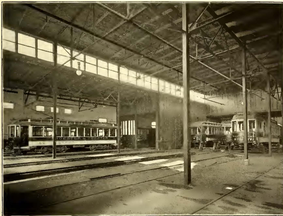
INTERIOR OF CAR HOUSE
