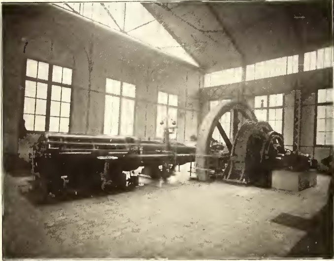
FIG. 3.—INTERIOR OF ENGINE ROOM
