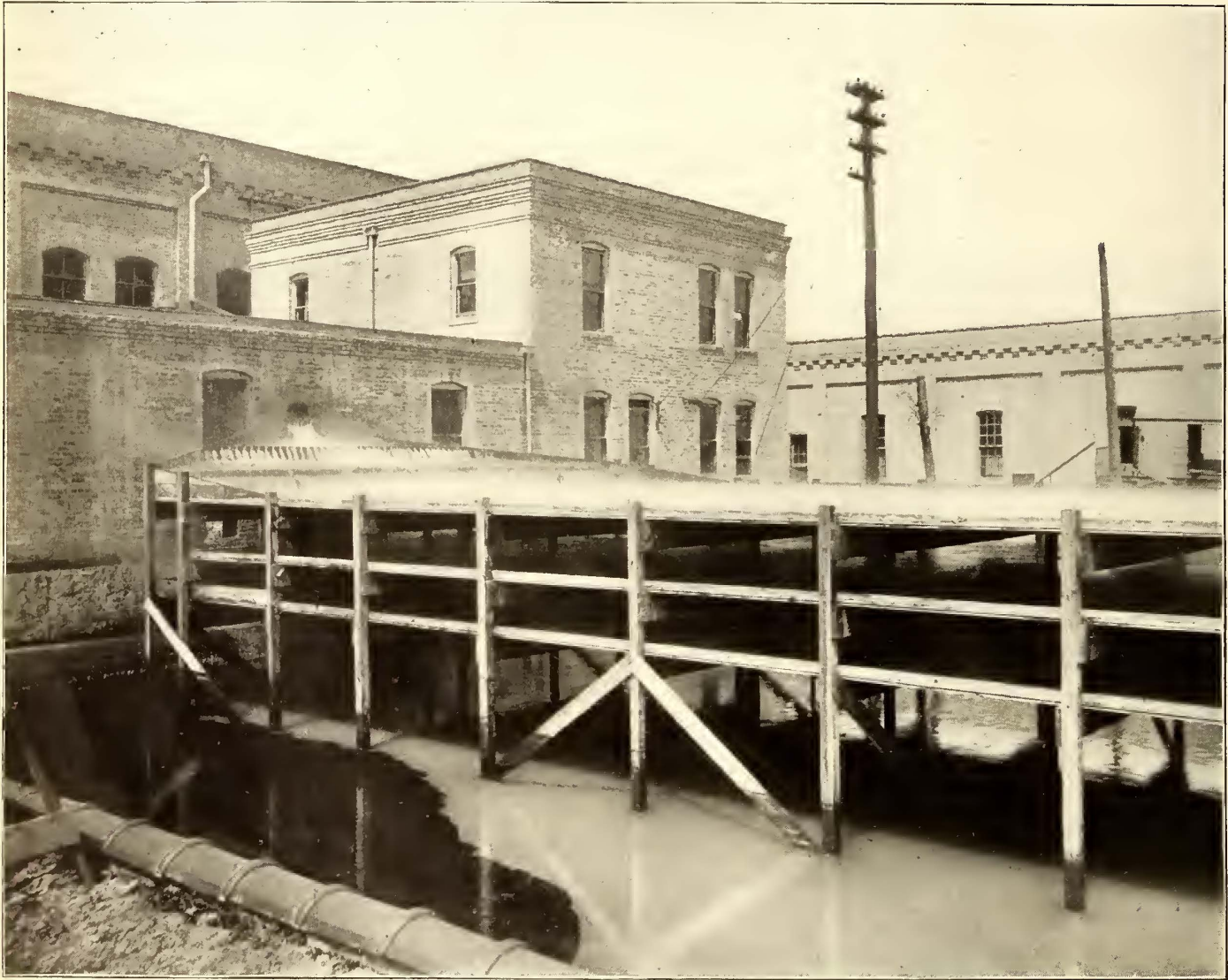
FIG. 2.—COOLING TABLE AND POND
