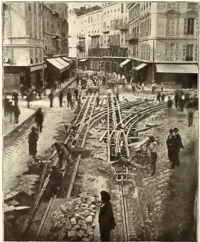
LAYING A PART OF THE CONDUIT SECTION
