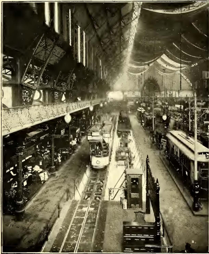
VIEW OF ONE SIDE OF HALL
