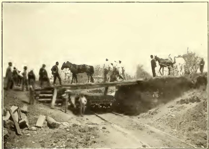
FILLING GRAVEL CARS
