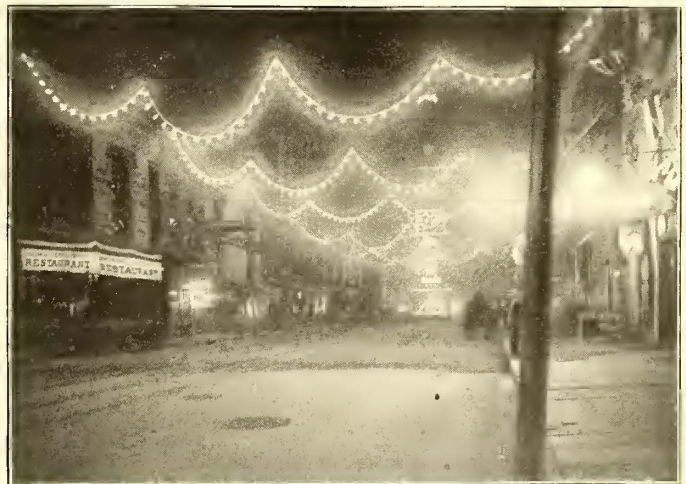
ILLUMINATED STREET, MILWAUKEE
