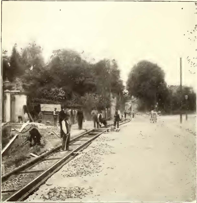
LAYING TRACK ALONG ROUTE D'HERMANCE, NEAR PARK DES EAUX VIVES
