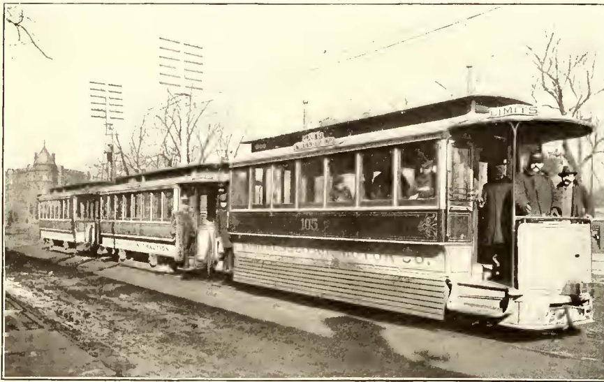
FIG. 1.—COMPRESSED AIR MOTOR CAR AND TWO TRAILERS, NORTH CLARK STREET, CHICAGO
