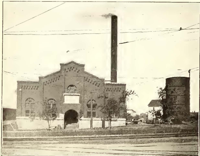
EXTERIOR OF POWER STATION
