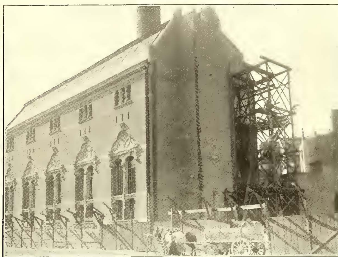
FIG. 17.—VIEW OF POWER STATION WITH SCAFFOLDING FOR ERECTION OF BOILERS
