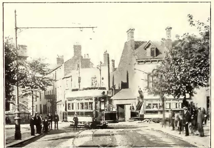
LONG BRACKET POLE AT TURNOUT
