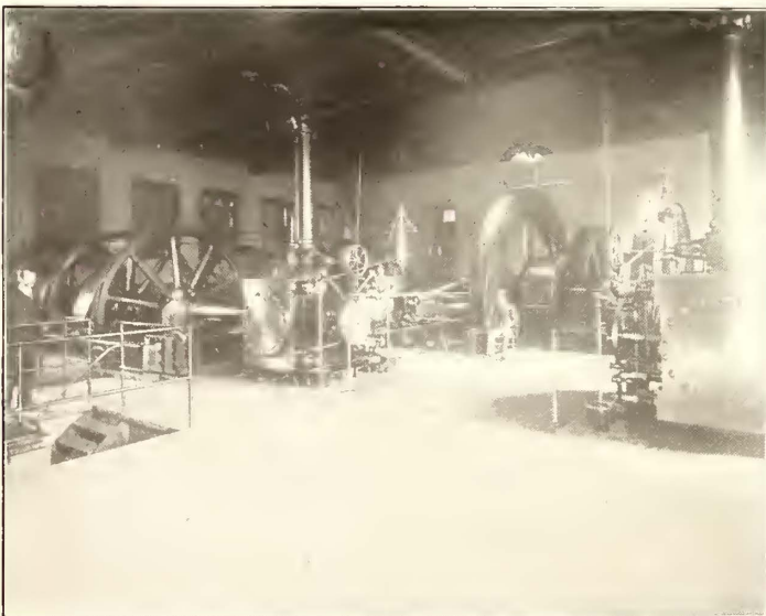
CABLE STATION AND TENSION RUNS, FIFTEENTH STREET AND GRAND AVENUE
