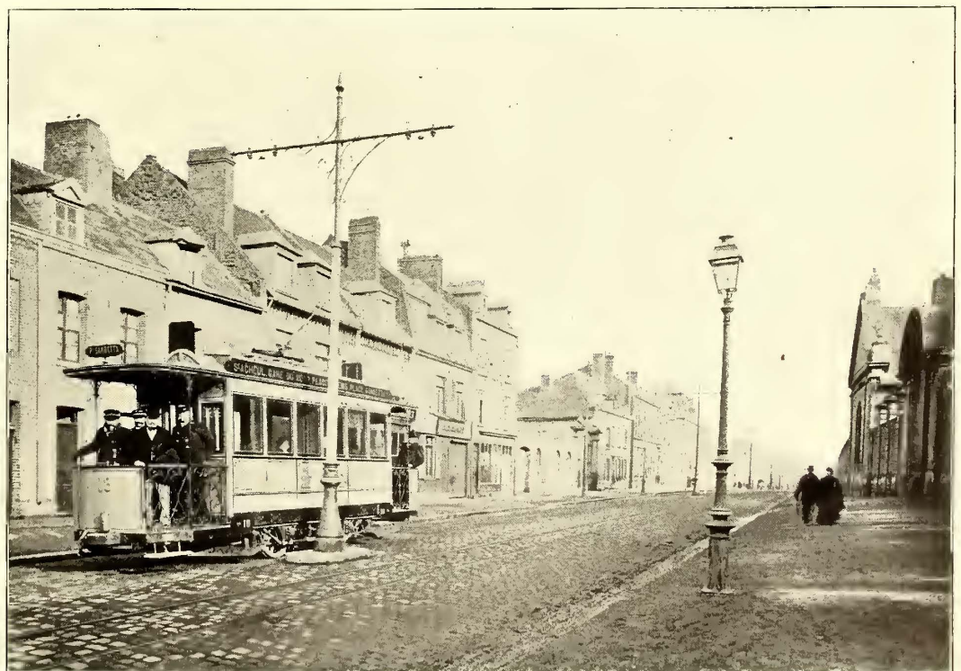
FIG. 16.—CENTER POLE CONSTRUCTION IN PROVINCIAL CITY
