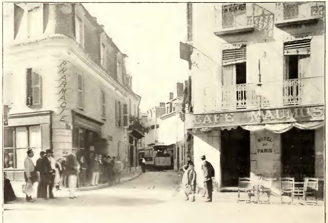
FIG. 19.—OVERHEAD CONSTRUCTION WITH ROSETTES IN LOURDES
