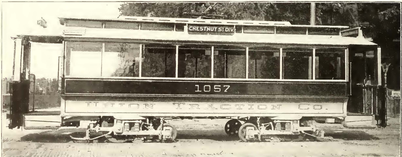
TRACK AND WHEEL BRAKE ON MAXIMUM TRACTION TRUCKS
