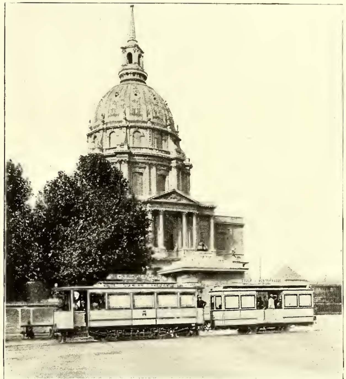
FIG. 31.—TRAIN ON THE NEW CONDUIT LINE OF THE CIE. GENERALE PARISIENNE DE TRAMWAYS
