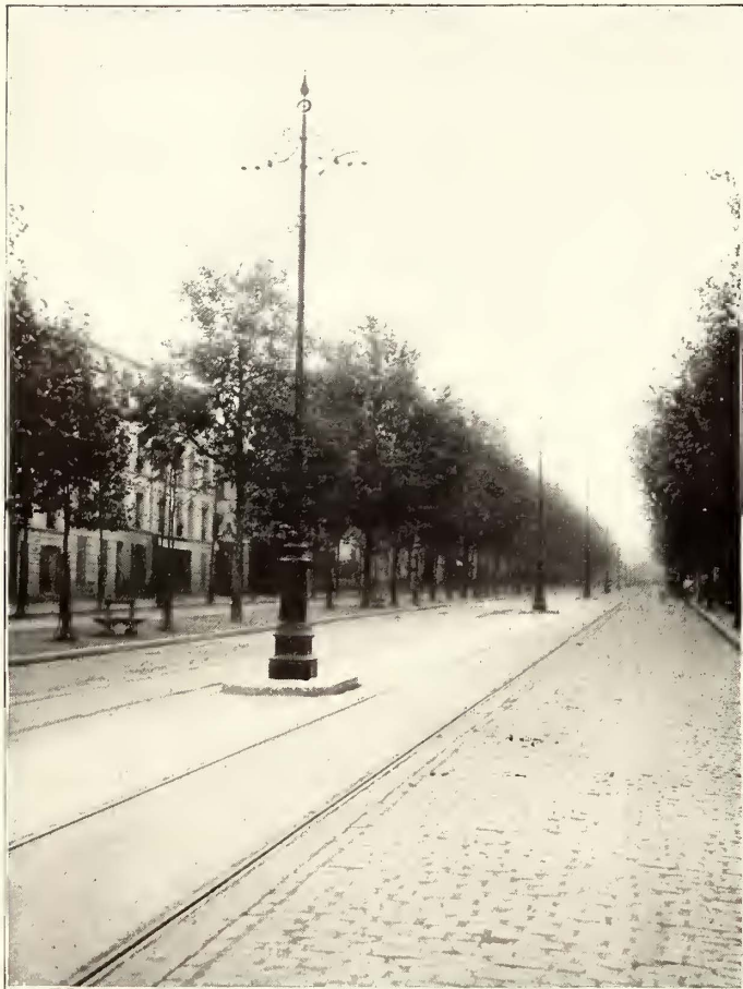
FIG. 14.—CENTER POLE CONSTRUCTION ON AVE. DUMESNIL, PARIS
