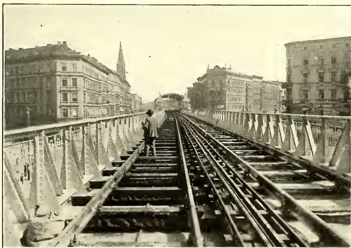
FIG. 16.—VIEW OF STRUCTURE WITH TEMPORARY TRACK FOR WORK TRAINS
