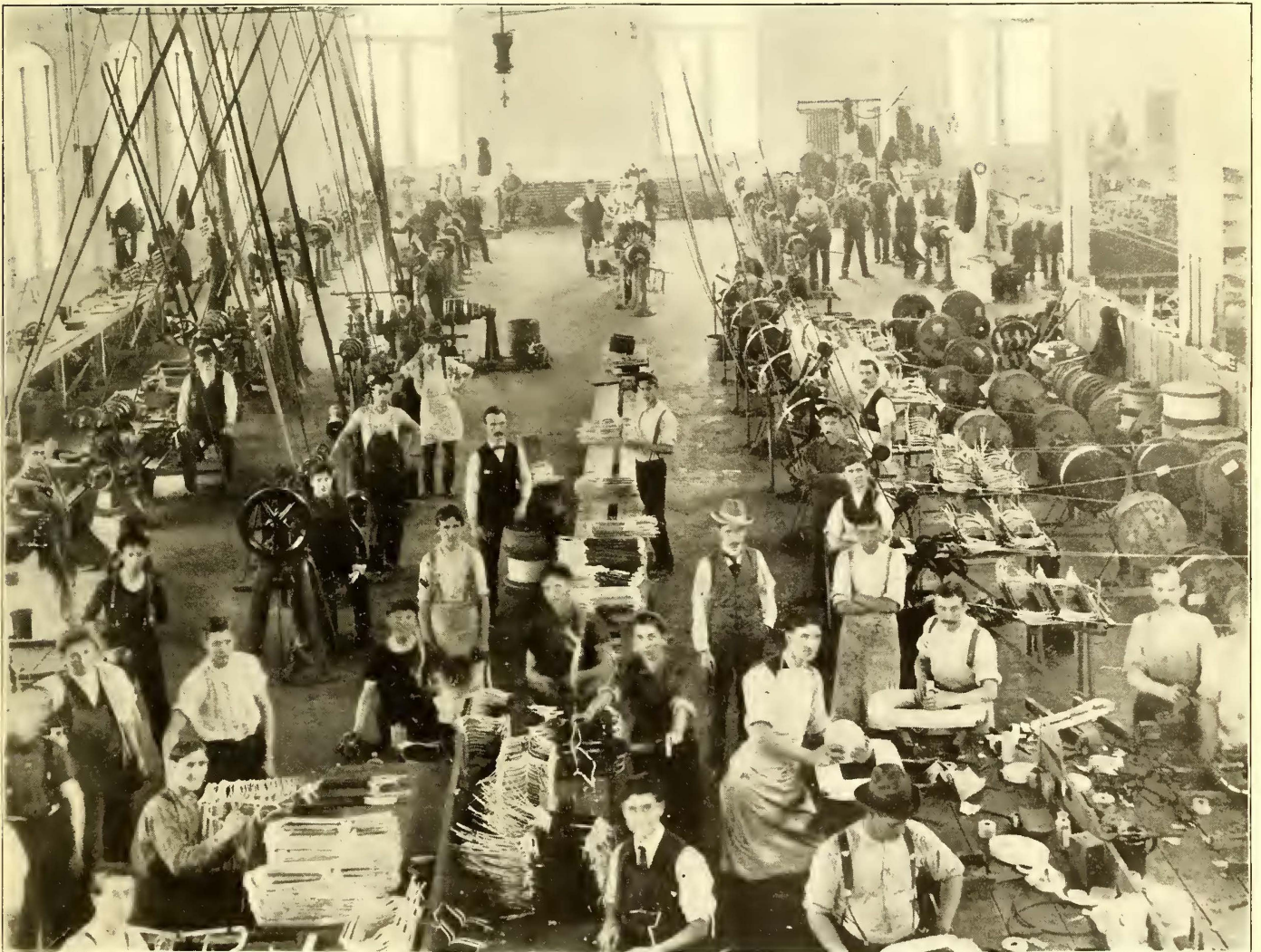
GENERAL VIEW OF ELECTRICAL DEPARTMENT
