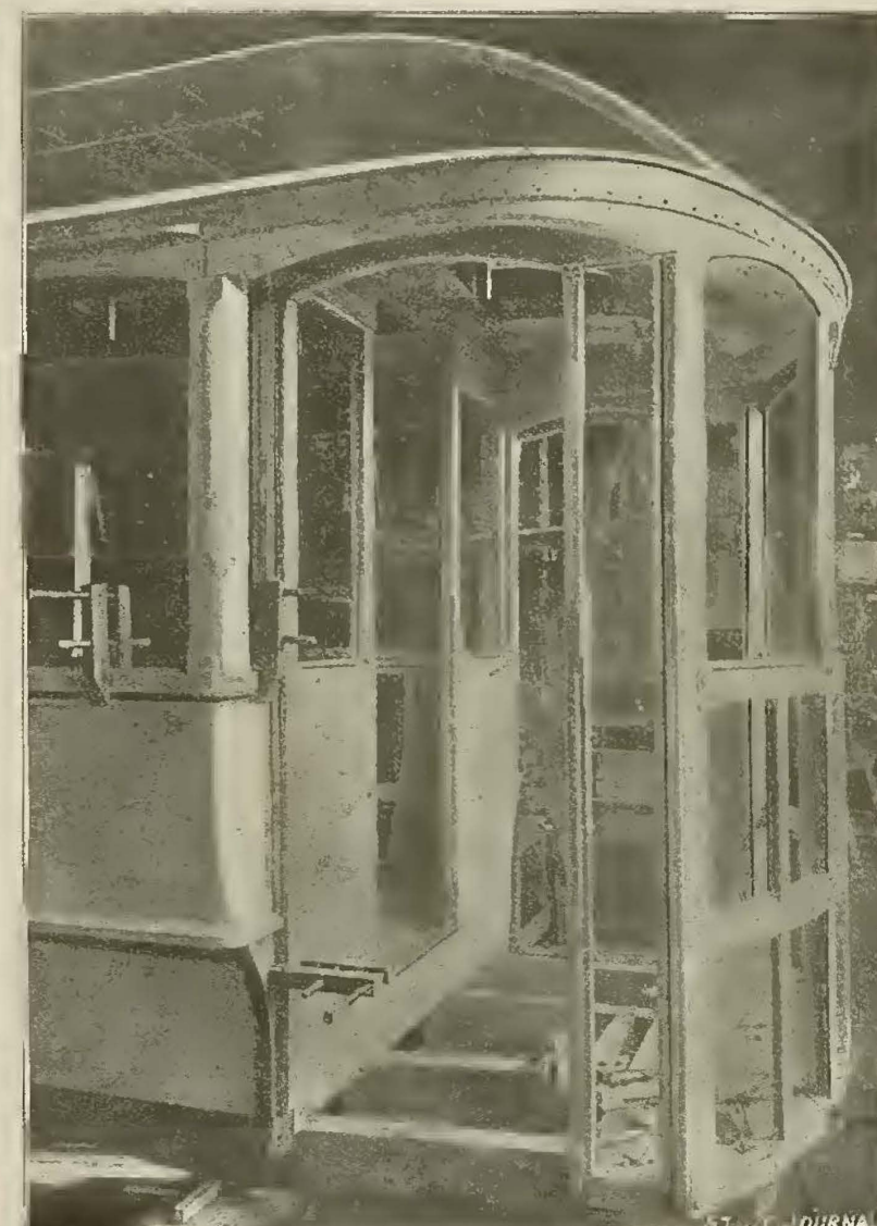
FIG. 625. FRAMING OF VESTIBULE
