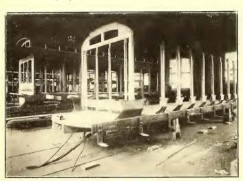
The step supports, which are bolted to the sills, are made very heavy, and the guard behind the step, instead of being made of light wood, is a strip of  $\frac{3}{4}$ -in. iron, which is intended to help out the channel iron sills in acting as a truss. The construction of the ends is easily seen. The dash is flush with the end of the platform. The cars are "single enders," made to be operated only one way, as is the universal practice in Detroit.
