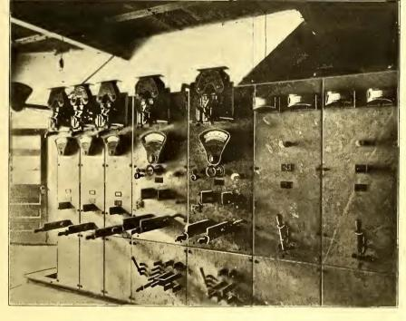
FIG. 7.—SWITCHBOARD OF WASH STREET SUBSTATION
