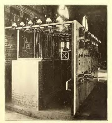
FIG. 4.—SWITCHBOARD WIRING AND BRICK CELLS FOR OIL SWITCHES
