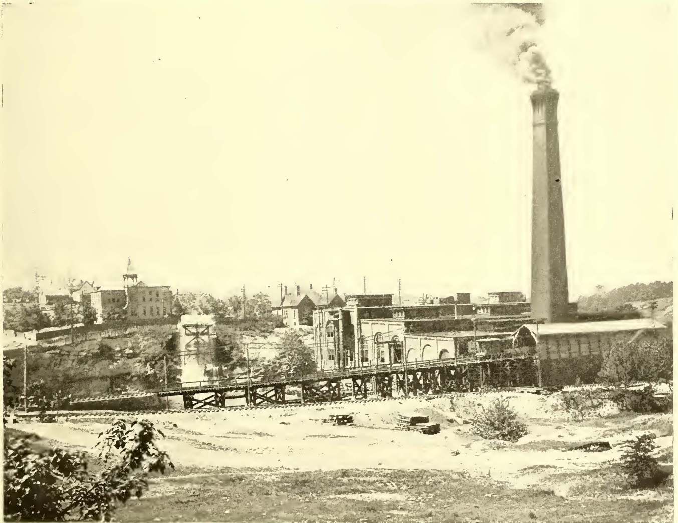
THE GEORGIA ELECTRIC LIGHT COMPANY'S PLANT WHICH FURNISHES POWER TO THE ATLANTA RAPID TRANSIT CO.
