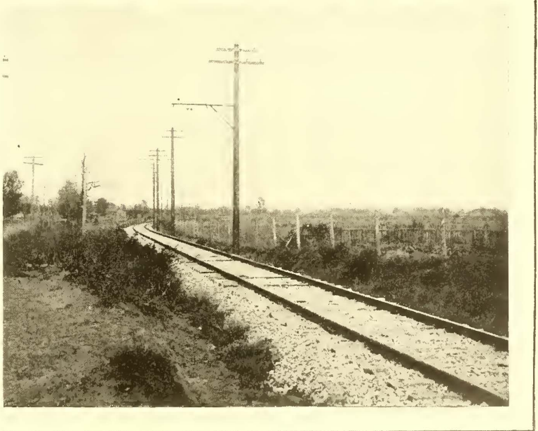
VIEWS OF CURVE AND TANGENT TRACK CONSTRUCTION
