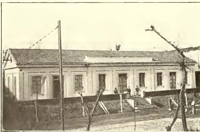
SUBSTATION AT MELITO
