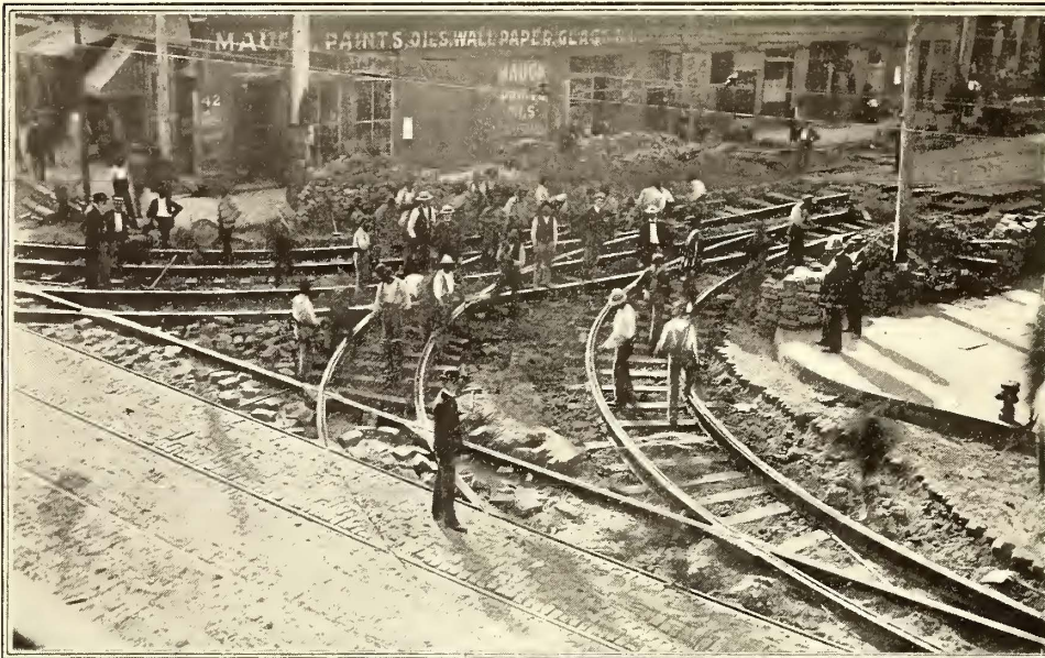
LAYING SPECIAL WORK
