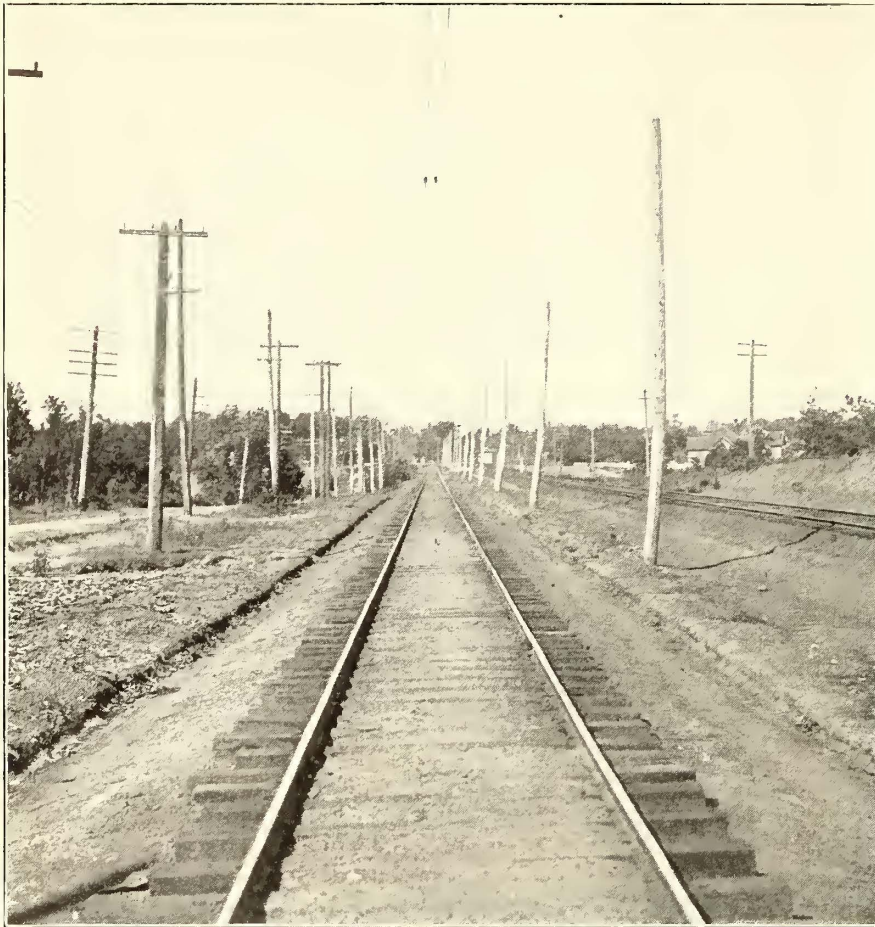
TWO-WIRE CONSTRUCTION—DECATUR LINE
