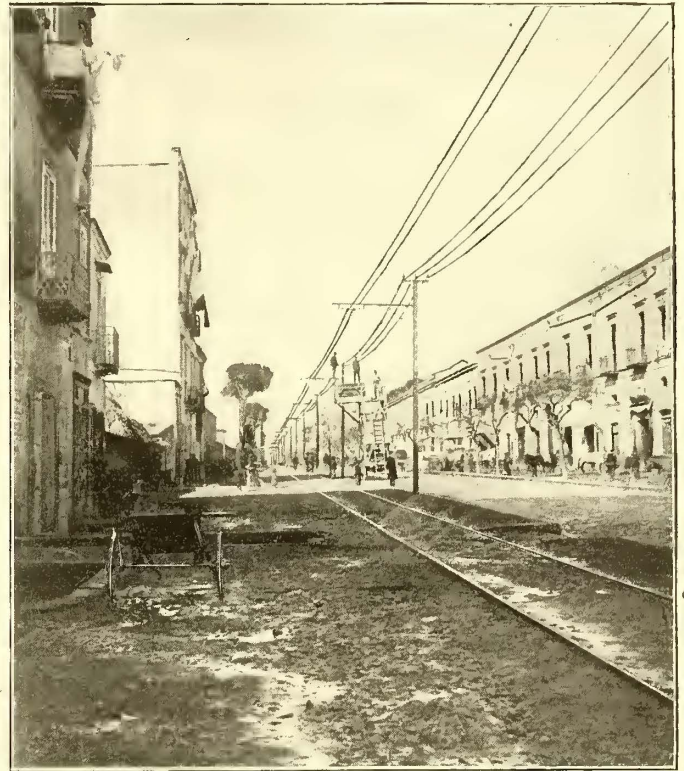
VIEW, SHOWING LINE CONSTRUCTION
