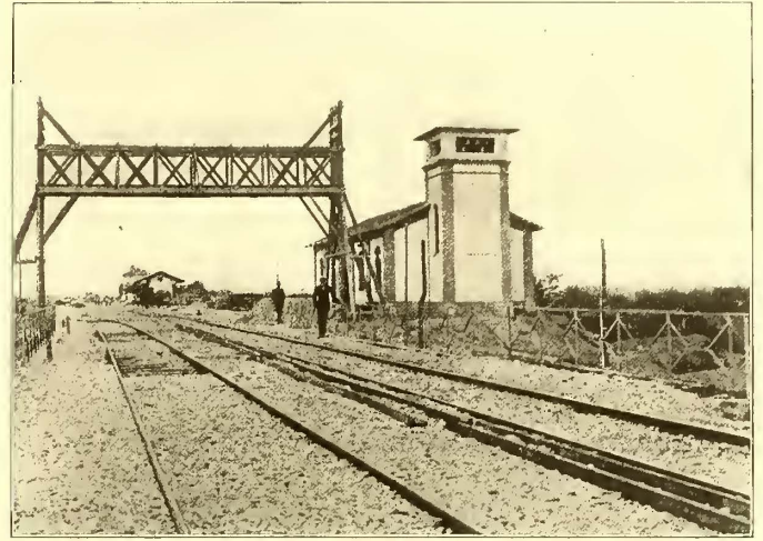
ONE OF THE SUBSTATIONS
