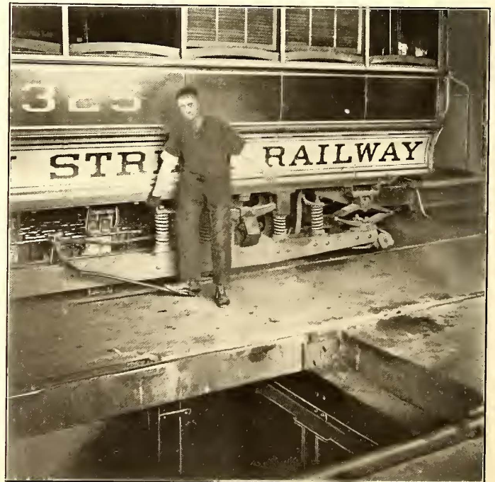
LOADING BATTERY ON TO CAR
