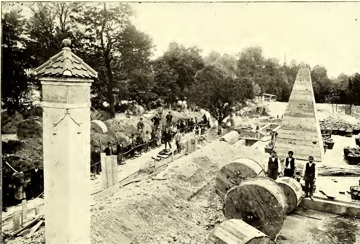
Laying of Felten & Guilleaume's Electric Light Cables in Munich.
