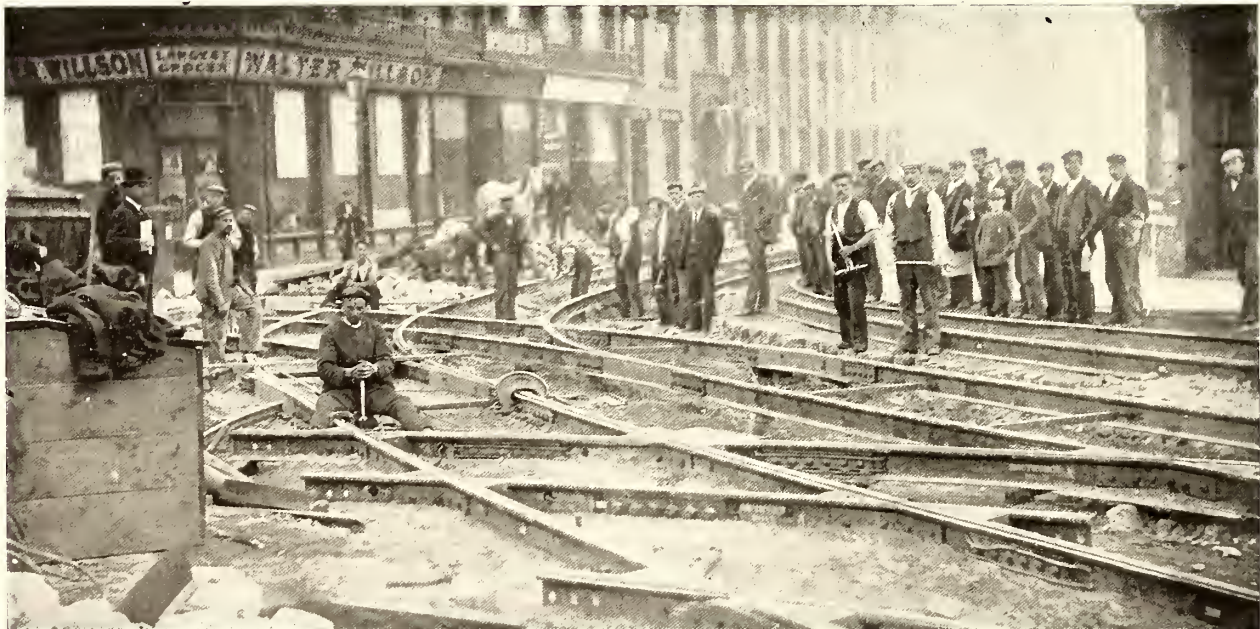
PERMANENT WAY CONSTRUCTION SUNDERLAND, ENGLAND
