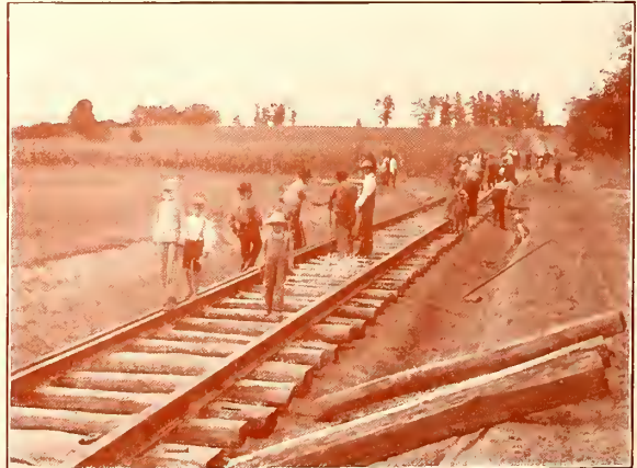
Track Construction, Canton-Akron Railway.
