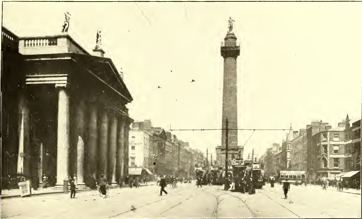
LOWER SACKVILLE STREET, SHOWING GENERAL POST OFFICE AND NELSON'S PILLAR. DUBLIN UNITED TRAMWAYS
