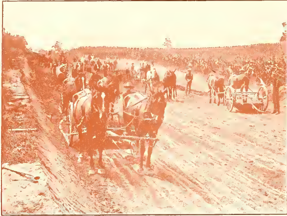
Grading Outfit, Crescent Extension Peoria & Pekin Terminal Railway.
