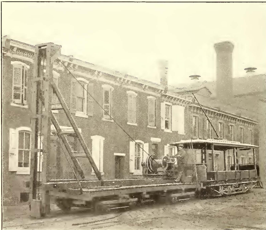
FIG. 2.—DROP HAMMER IN OPERATION
