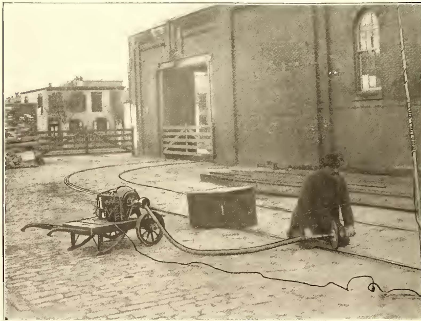
FIG. 12.—ELECTRICALLY DRIVEN PORTABLE EMERY WHEEL
