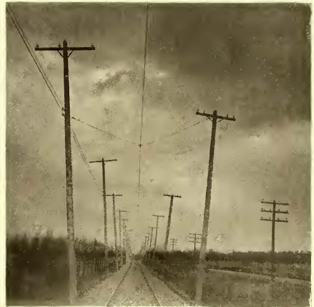
FIG. 1.—TYPICAL VIEW OF A SECTION OF TRACK
