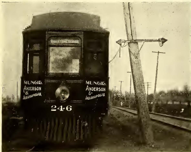
FIG. 2.—METHOD OF RECEIVING DISPATCHERS' ORDERS. TELEPHONE IN CAB
