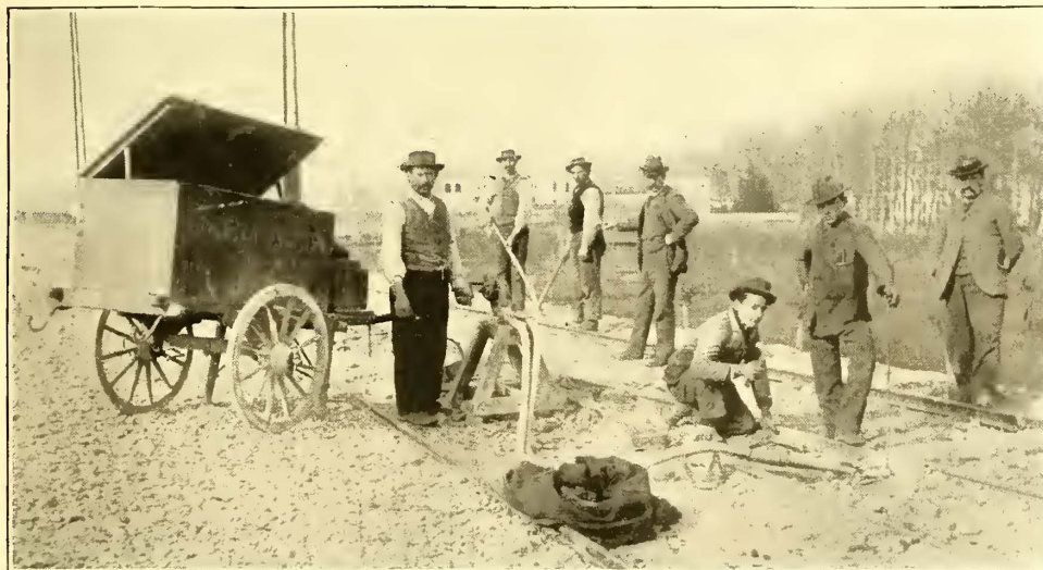
FIG. 2.—METHOD OF BRAZING RAIL BONDS
