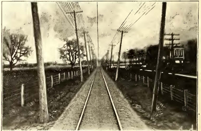
FIG. 5.—A GOOD TRACK FOR 50 MILES AN HOUR
