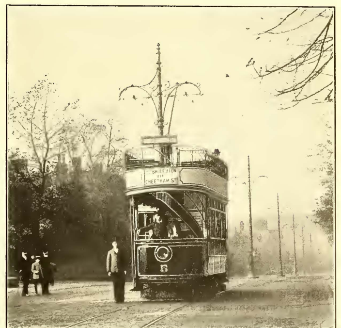
CENTER POLE CONSTRUCTION
