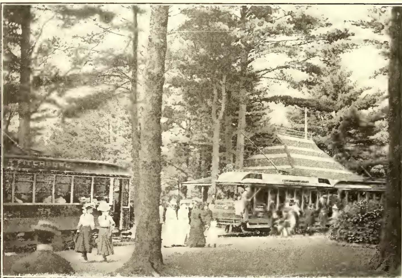
TERMINAL STATION AT PARK
