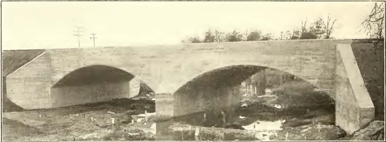
35-FT MASONRY ARCHES
