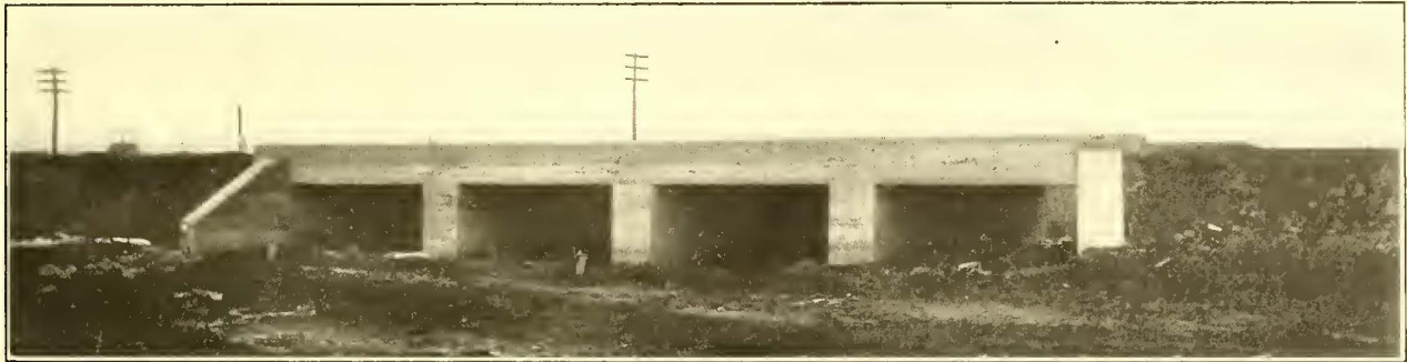
MASONRY AND STEEL BRIDGE—AURORA, ELGIN & CHICAGO RAILWAY
