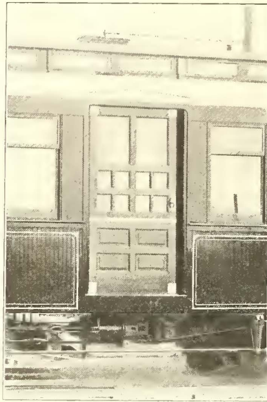
FIG. 11.—CENTRAL ENTRANCE FOR ELEVATED RAILROAD CAR
