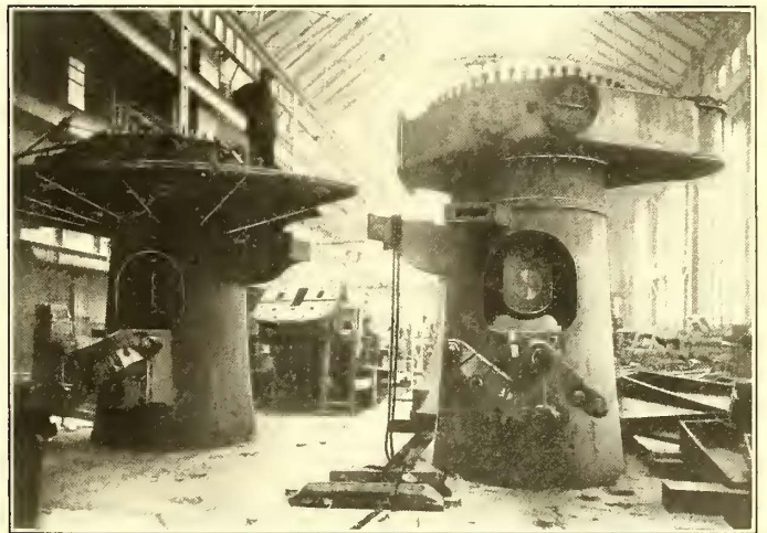
ENGINE PARTS BEFORE ERECTION
