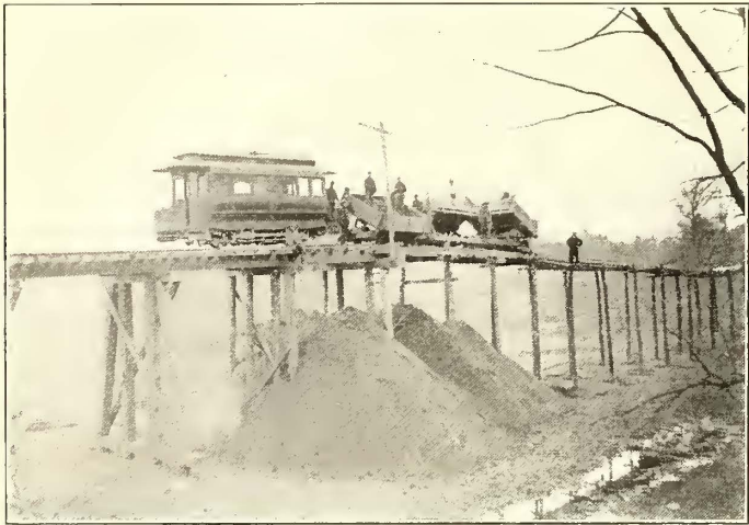
TRESTLE AND FILL AT SCANTIC RIVER
