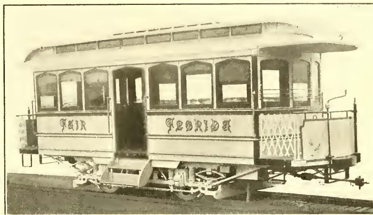
FIG. 13.—CENTRAL VESTIBULE WITH TWO STEPS
