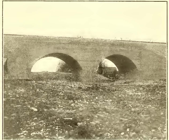
15-FT MASONRY ARCH AND FILL
