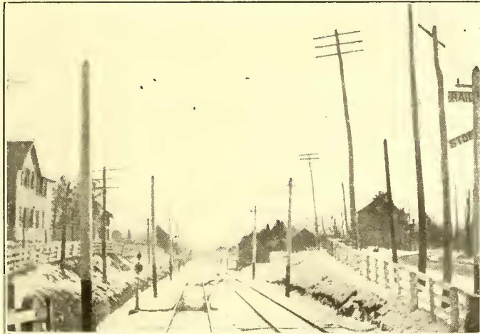
DOUBLE TRACK CONSTRUCTION
