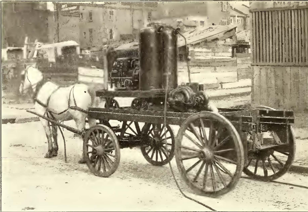
FIG. 9.—COMPRESSING APPARATUS FOR PNEUMATIC RIVETER
