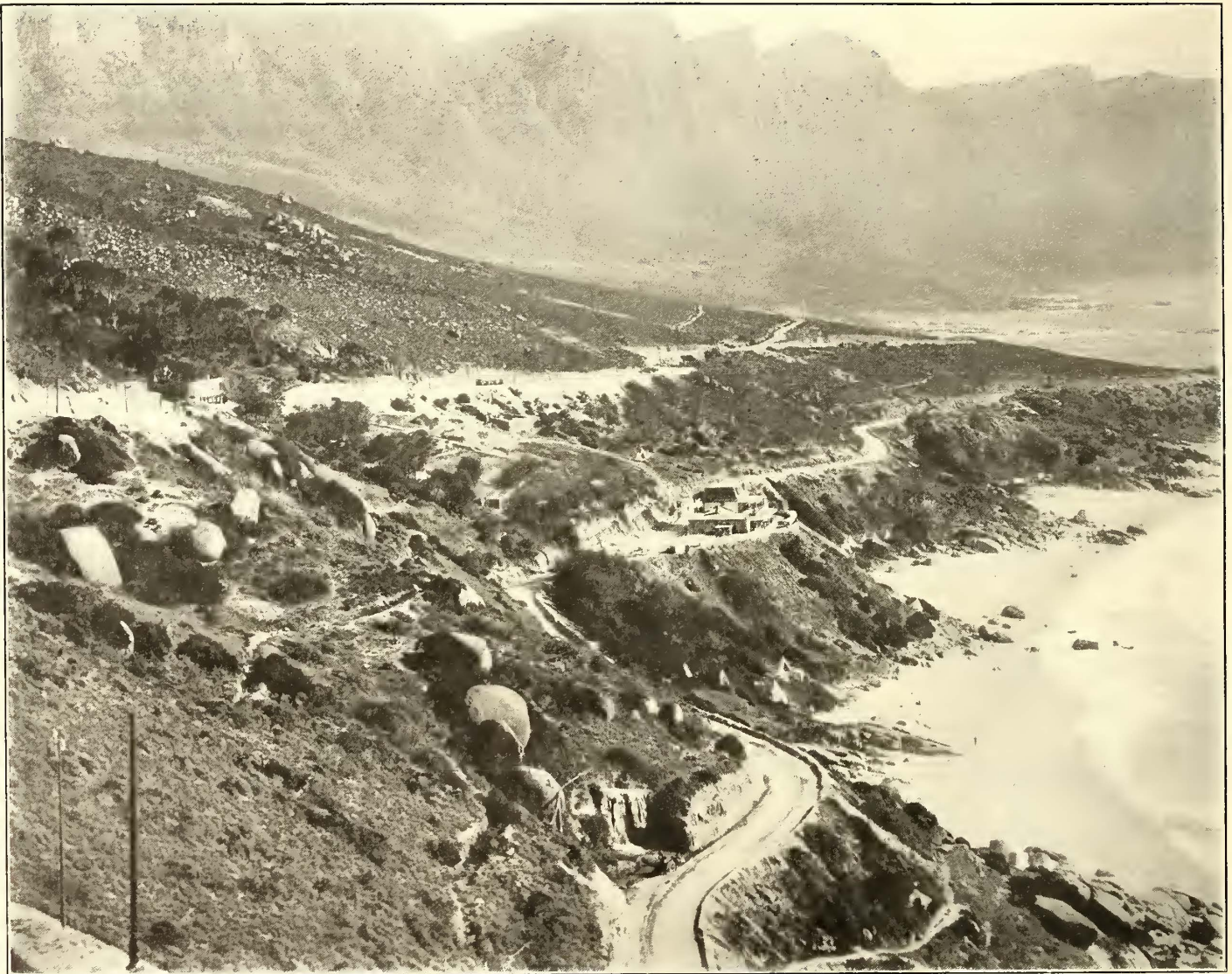
GENERAL VIEW OF PART OF ROUTE, ASCENDING GRADE
