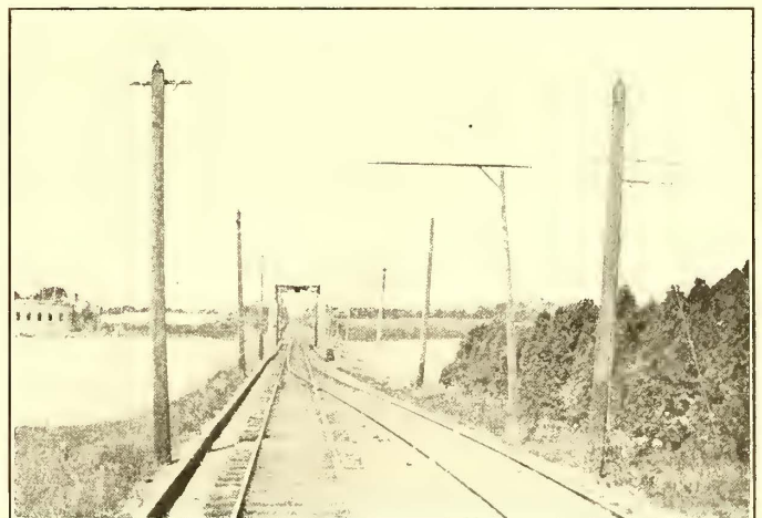
CROSSING A SINGLE TRACK BRIDGE
