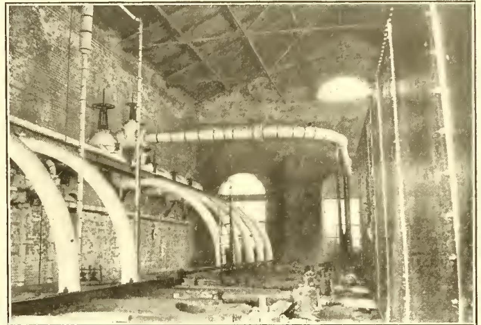
BOILER ROOM ABOVE BOILERS
