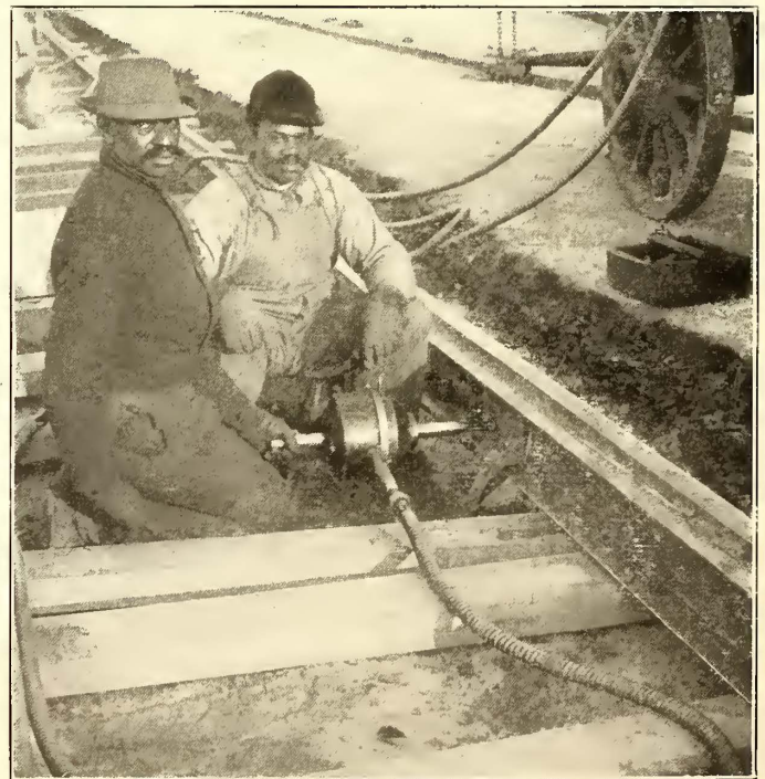
FIG. 6.—PNEUMATIC REAMER AT WORK
