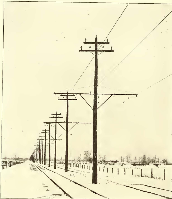
HIGH AND LOW-TENSION LINE CONSTRUCTION
