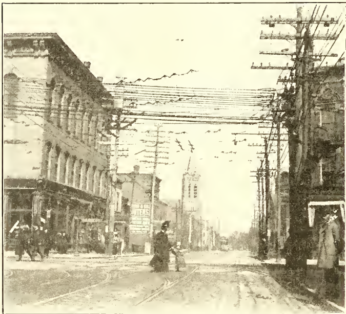
DOUBLE TROLLEY AT CINCINNATI—NETWORK OF OVERHEAD WIRES IN RESIDENCE DISTRICT
