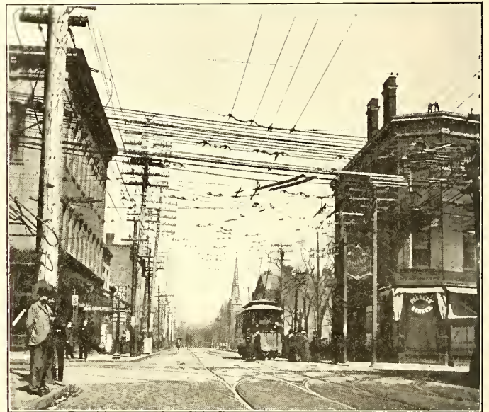
DOUBLE TROLLEY AT CINCINNATI—NETWORK OF OVERHEAD WIRES IN RESIDENCE DISTRICT
